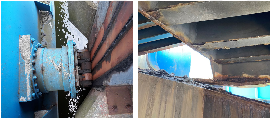
Figure 4.15 : Support at the location of dolphin (left) and pontoon (right).
