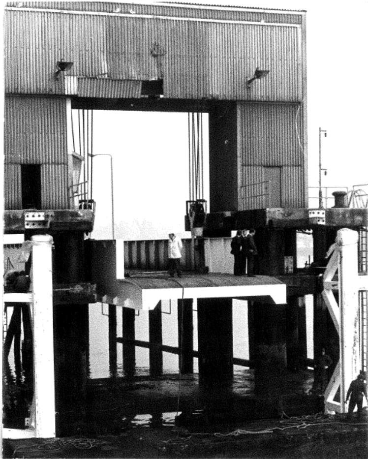
Figure 2.2 : Historic photo from seaward end of the original suspended linkspan.
