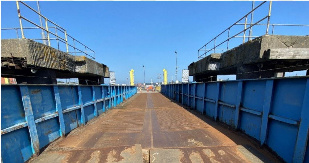
Figure 3.2 : Overall Condition of Deck Plate – Pontoon End.
