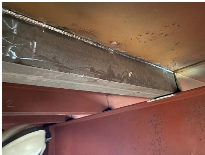
Figure 7.3 : Fit-up and welding of new longitudinal stiffeners.
