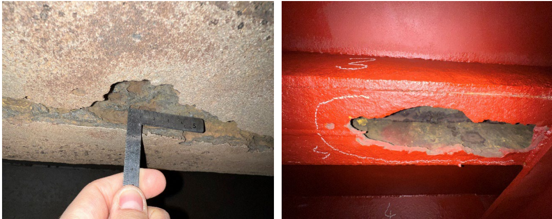
Figure 3.10 : Dimensional Inspection of Longitudinal Stiffeners.
