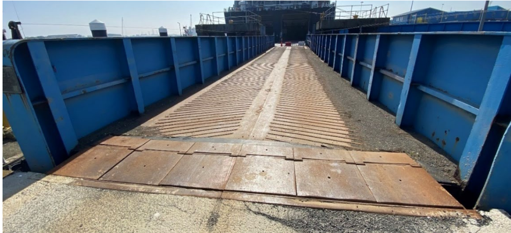
Figure 3.3 : Overall Condition of Deck Plate – Abutment End.
