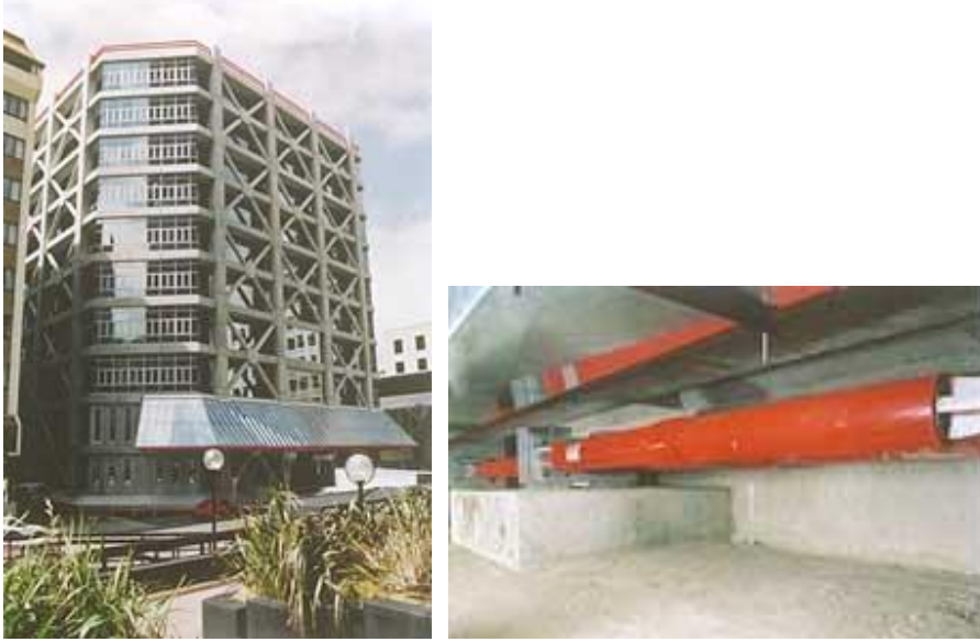
Şekil 5.11 Wellington Police Station
