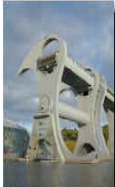
Millennium Wheel Canal Link, 2002, RMJM Mimarlık
