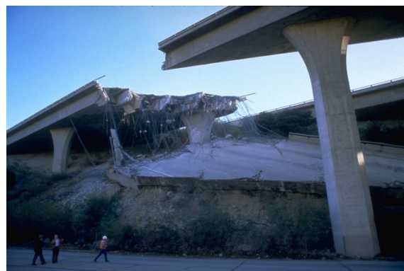
Figure 3.7 : Northridge earthquake damage (Eplett, 1994)
