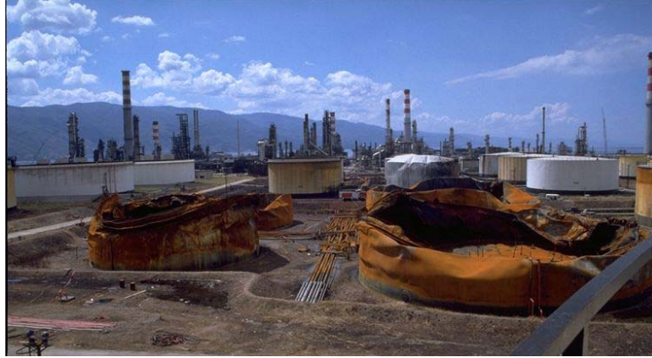
Şekil 1.1 : Tüpraş rafinerisinde oluşan yangın hasarı (National Information Service for Earthquake Engineering, University of California, Berkeley)
