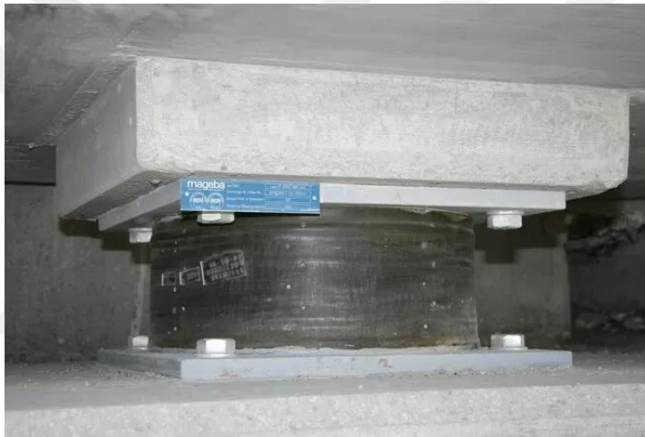
Figure 1.7 : High damping rubber bearing (URL-4).
