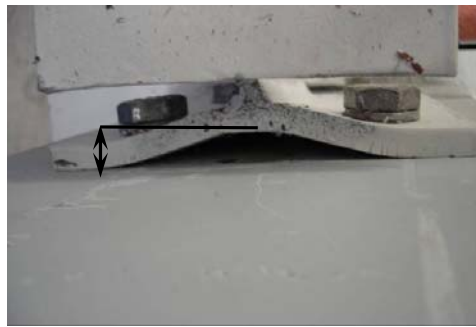
Figure 7.10: Gap between the Beam End Plate and Column Flange (Specimen BF-H, Cycle 31 and Top Disp. of 81.81mm)
