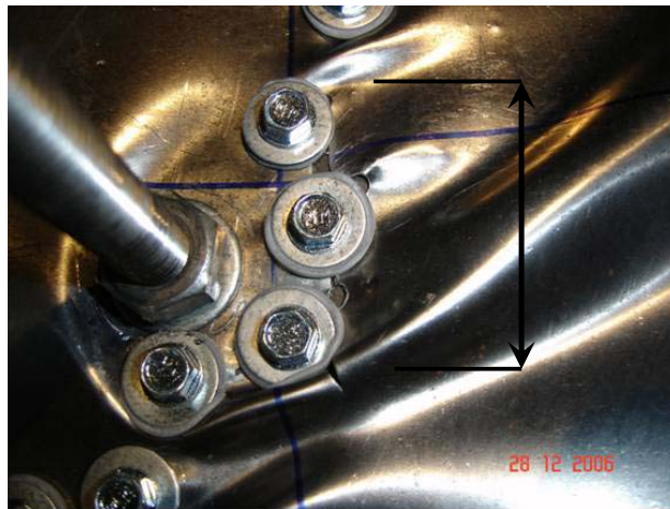
Figure 7.49: Infill Tear in Upper North Corner (Specimen SW-B-H, Cycle 34 and Top Disp. of +32.40mm)
