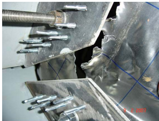
Figure 7.32: Net Section Failure in North Upper Corner (Specimen SW-A-H, Cycle 34 and Top Disp. of -58.80mm)
