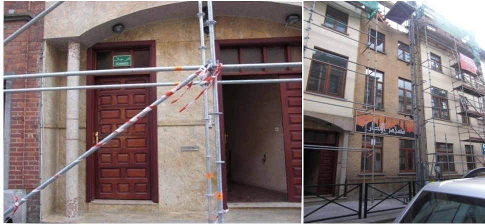
Figure 3.8: A mosque under construction in Street C, Schaarbeek
