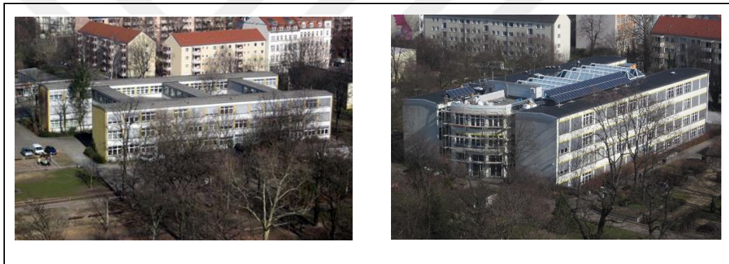
Figure 3.22 : Bertolt-Brecht-School (Left: before covering the courtyard roof) and (Right: converting courtyard to atrium).
