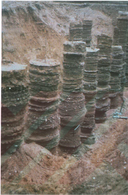
Fig. 2.2 Jet Grout Columns [20]
