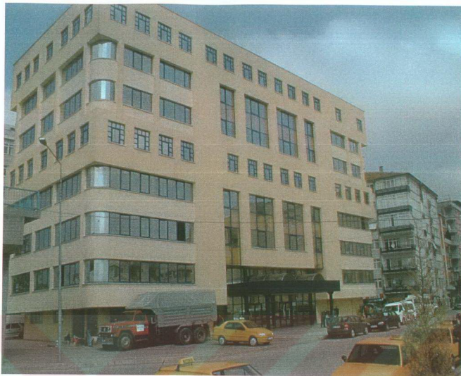
Fig. 3.1 General Directorate Building of KEDAS
