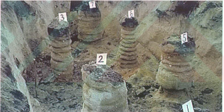
Fig. 2.1 Jet Grout Columns [19]
