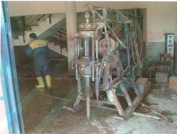
Fig. 3.19 Drilling Machine Taking Core Samples From The Jet Grout Columns
