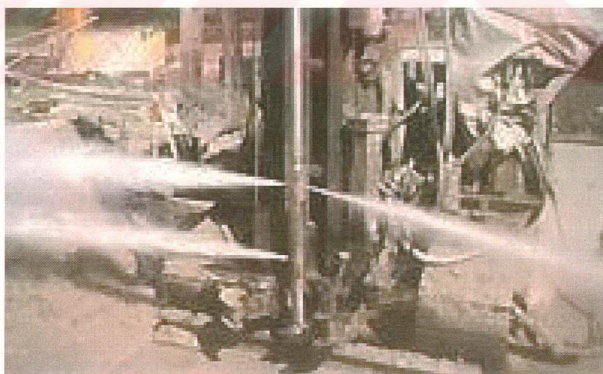
Fig. 2.8 Jet Nozzles in Process
