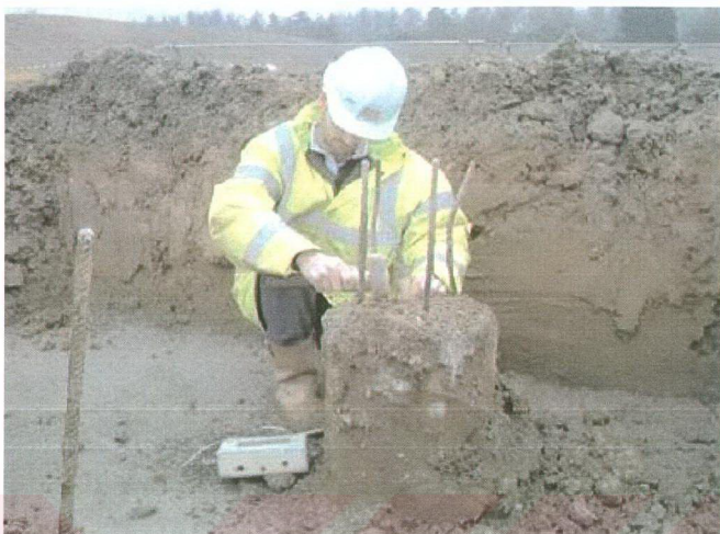
Fig. 2.23 Pile Integrity Application
