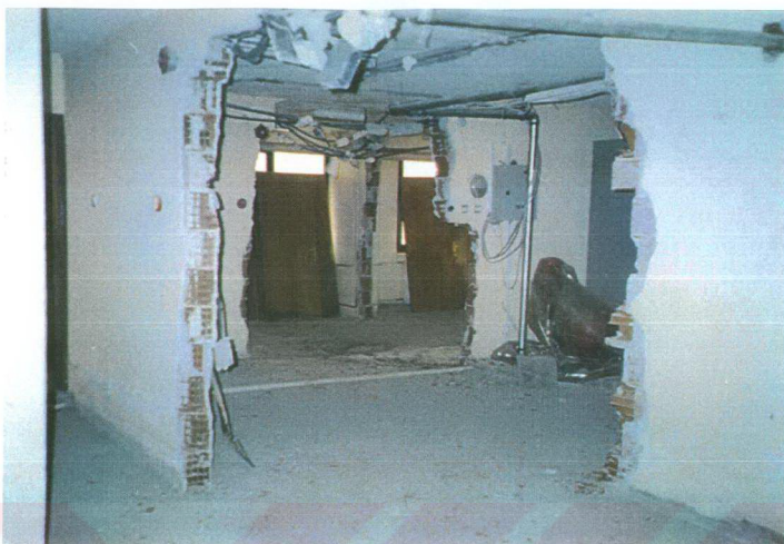
Fig. 3.15 Interior of KEDAŞ General Directorate Building Prepared For Jet Grouting Application
