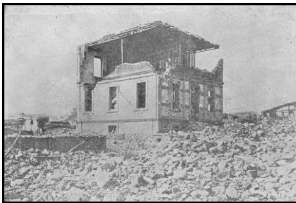
Figure A3.20 An isolated new building at Ganos experienced heavy damage by the strong tremor.
