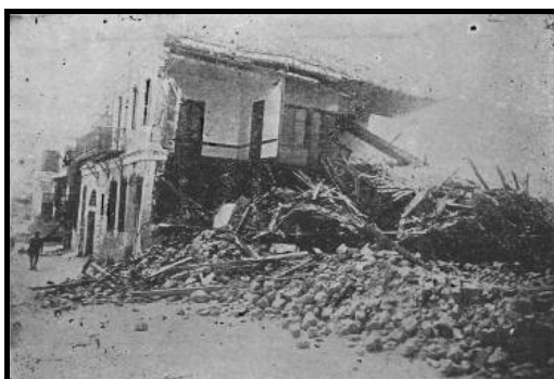
Figure A3.25 : Adjacent buldings of different type. The Stone building survived with slight damage, while the other was totally destroyed (M refte, Mihailovic, 1933).
