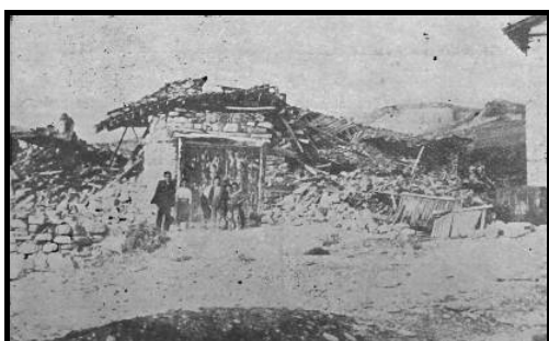
Figure A3.18: Three different type of buildings with damage at Ganos (Gaziköy). The left house was reduced to ruins, the middle was heavily damaged, the right house was slightly damaged (Mihailovic, 1933).
