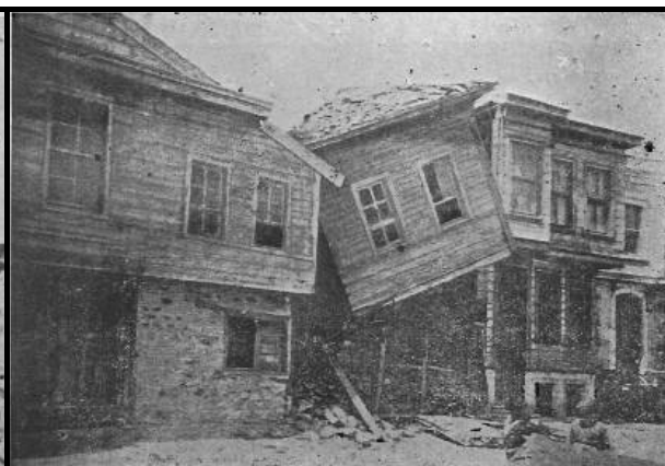
Figure A3.26 : A house, which wooden part tumbled to the side when the bricks underneath collapsed (M refte, Mihailovic, 1933).
