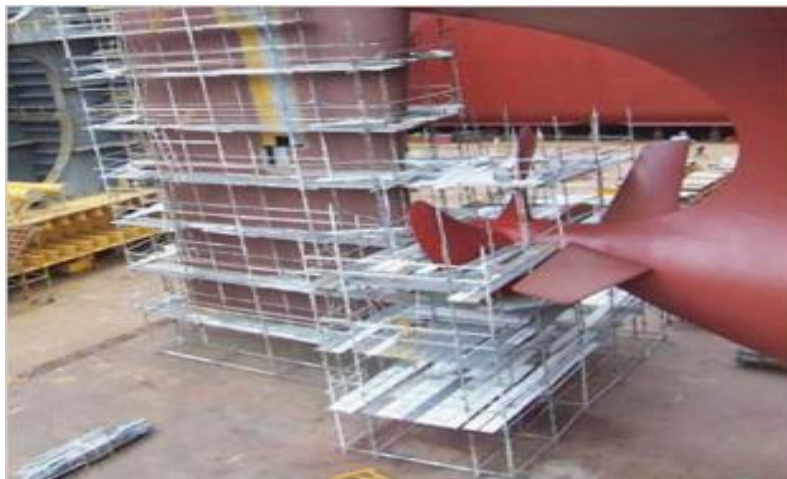
Figure 4.3 : Scaffoldings around rudder and propeller of the vessel [23].
