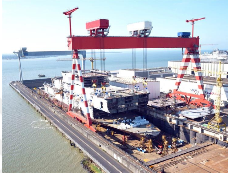
Figure 4.4 : Gantry crane at a shipyard [24].
