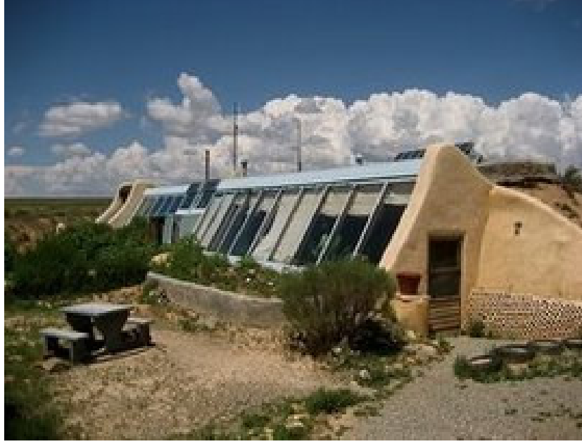
Şekil 3.11: EarthshipHome, Mike Reynolds, ( http://earthshipnews.com/2008/04/earthship-homes-gaining-appeal-during_23.html )
