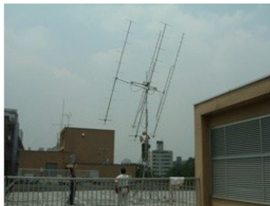
Figure 4.27 : VHF and UHF antennas on the University of Tokyo Ground Station.
