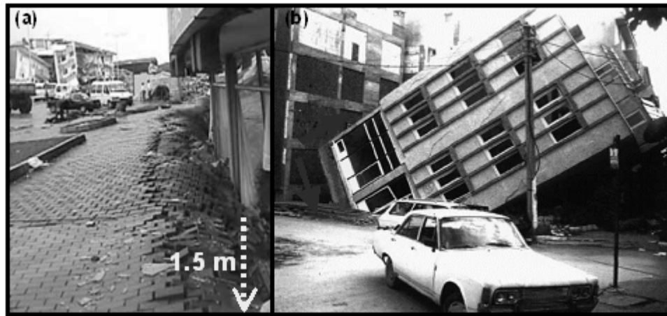
Figure 1.8 : Soil liquefaction during the 1999 Izmit Earthquake (3) (Photos from USGS, 2000 and Mollalahmutoglu, et al. 2003, respectively). The buildings in (a) and (b) were located in the city of Adapazari.
