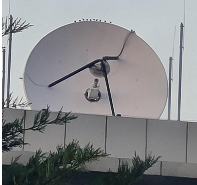
Figure 2.3 : S-band reflector antenna (UHUZAM).
