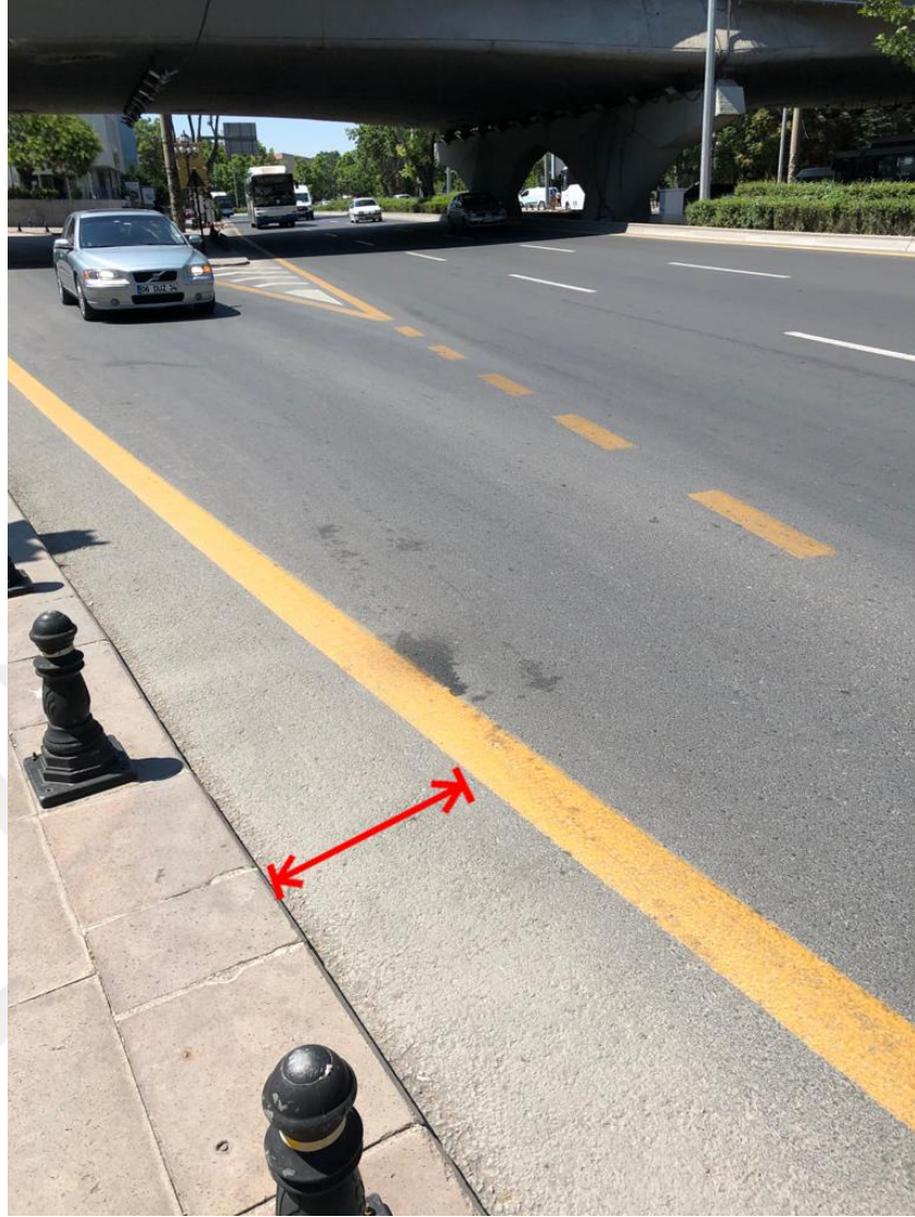
Figure 6.37 : Shoulder width in Atatürk Boulevard
