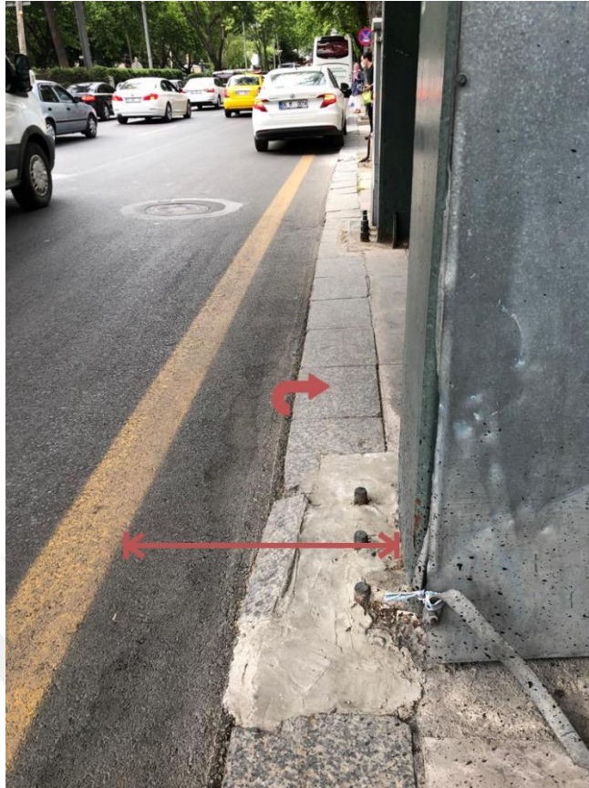
Figure 6.6 : Undesirable clear zone design
