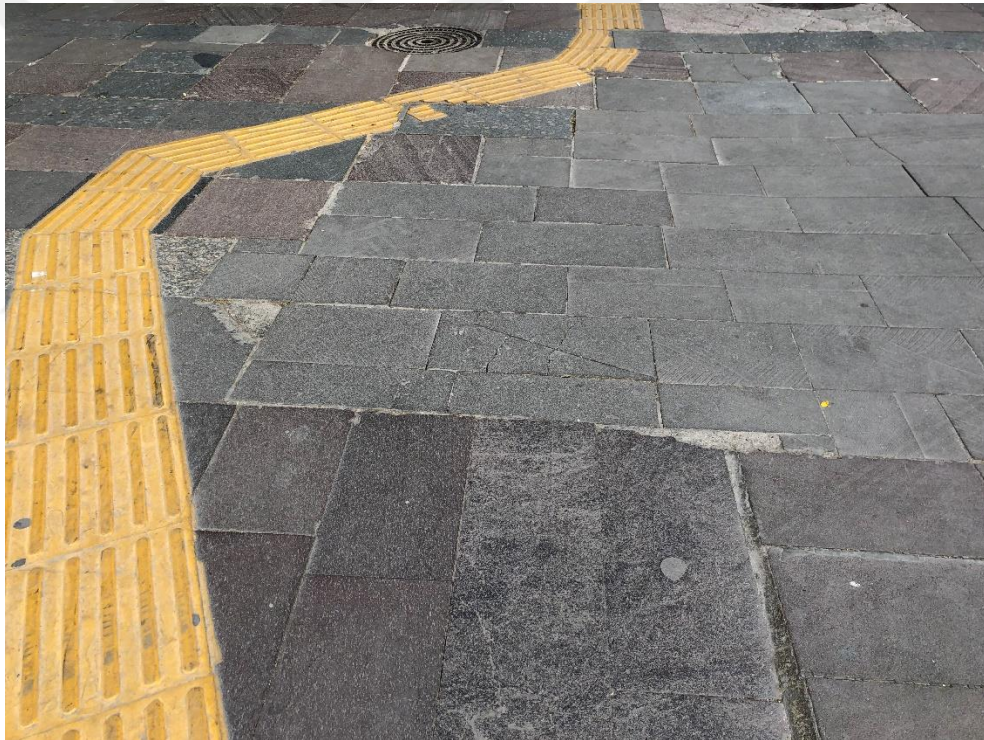
Figure 6.47 : A warning with the wrong guidance
