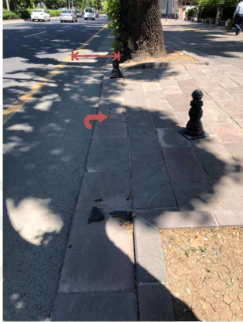
Figure 6.5 : Sample clear zone in Atatürk Boulevard
