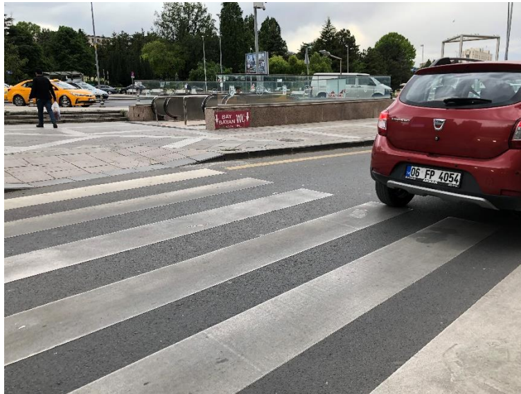
Figure 6.20 : Restricted sight distance due to metro entrance
