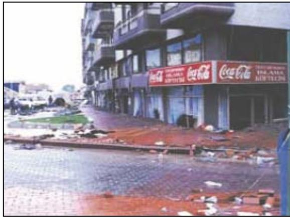
**Figure 4.13** Liquefied buildings with no structural damage (Photo: National Inst. of Standards and Technology)
