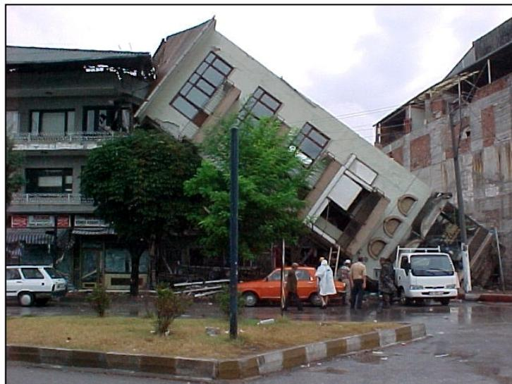
**Figure 4.11** Overturning of a five-storey building with aspect ratio about four (PEER,1999)
