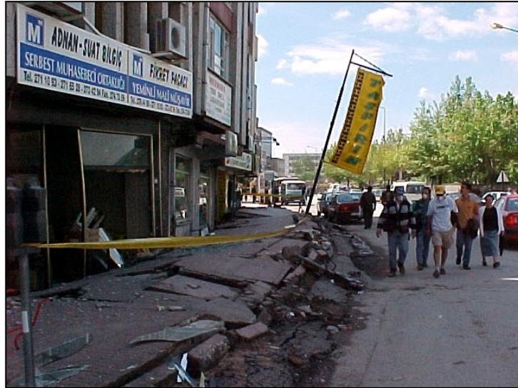
**Figure 4.10** Loss of bearing capacity and bulging of pavements (PEER,1999).
