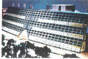
Şekil 4.16 Doxford International Business Park, Sunderland, PV'lerle kaplı güney cephesi ( www.graeme-peacock.com/e_photos/e-22.htm )
