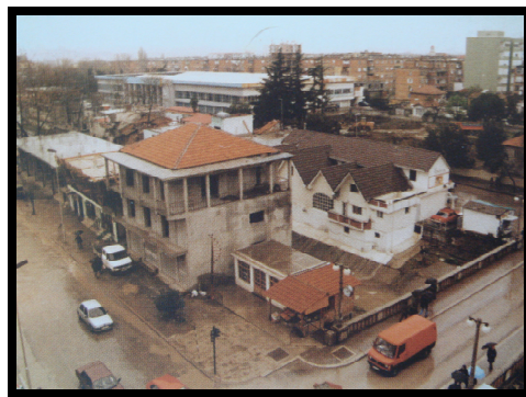
Figure 2.20 Illegal Construction over Lana River
