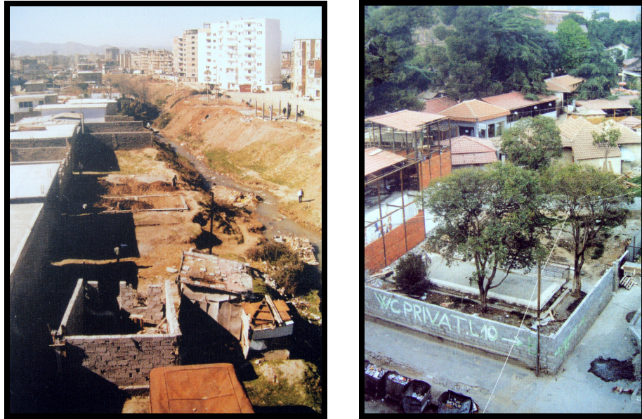
Figure 2.22 Degradation of the bed and banks of Lana (left) and occupation of the “Rinia” Park (right) by illegal constructions
