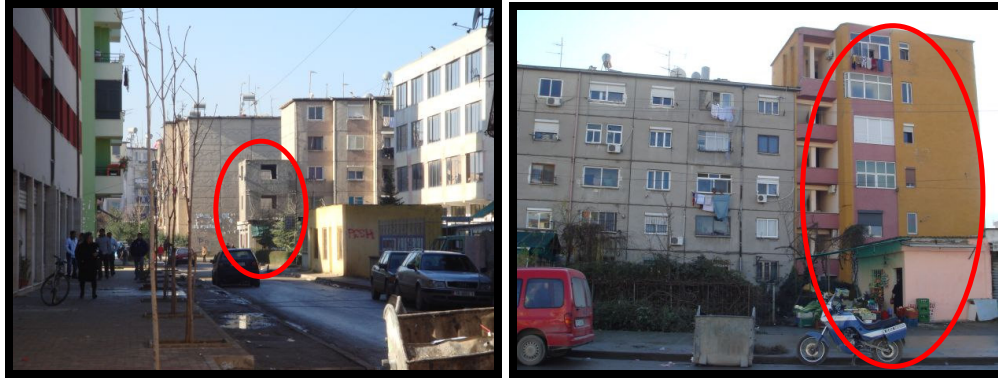
Figure 3.41 Examples of pavements and paths occupation in "Irfan Tomini" block case study area
