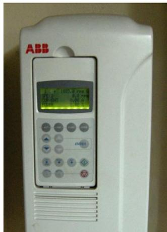
**Figure 2.3 :** Controller of the Centrifugal Pump.
