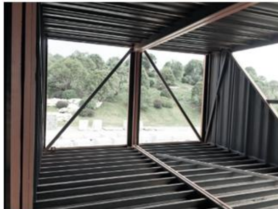
Figure 4.6: Diagonal bracing (Su et al., 2022, p. 11).
