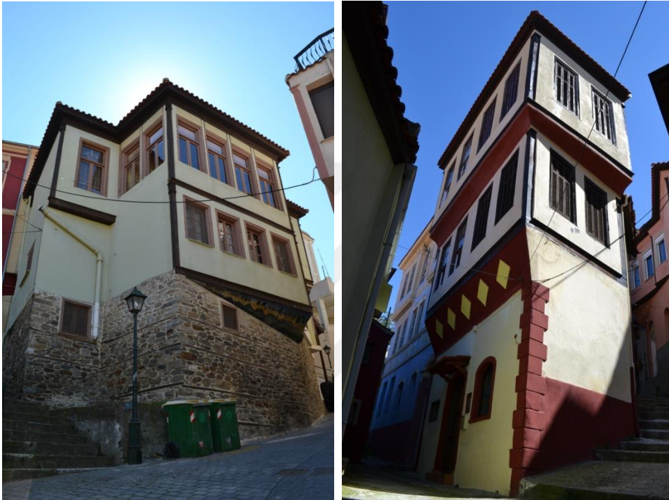
Figure 4.13 : House examples in the residential part of Ibrahim Pasha neighborhood. (Ivkovska 2016).
