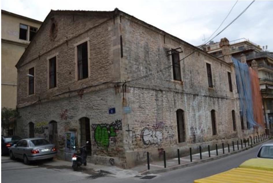
Figure 4.47 : The first offices of M. L. Herzog et Cie, built after 1891 (Ivkovska, 2015).
