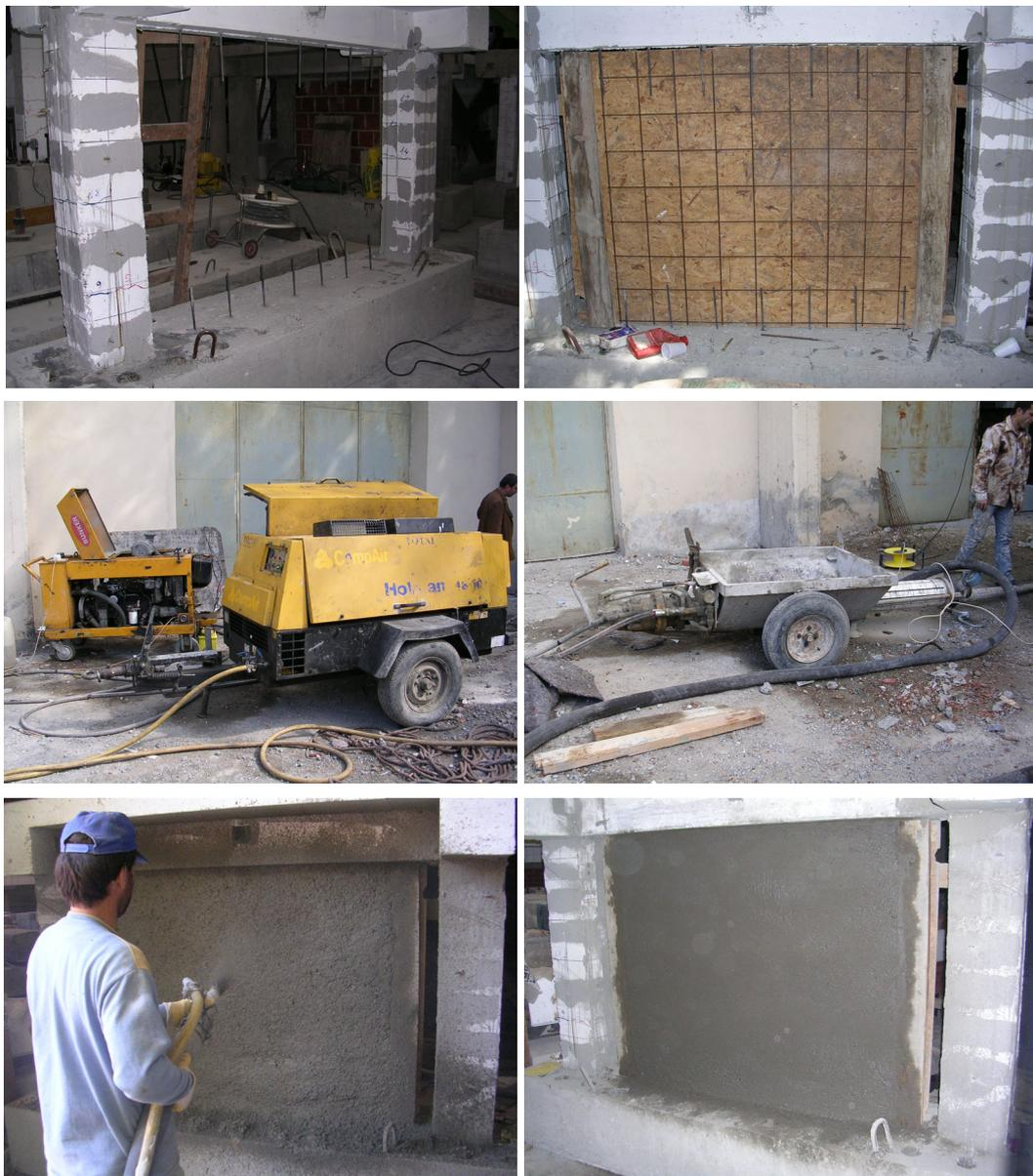
**Figure 3.7:** Construction of the shotcrete panels
