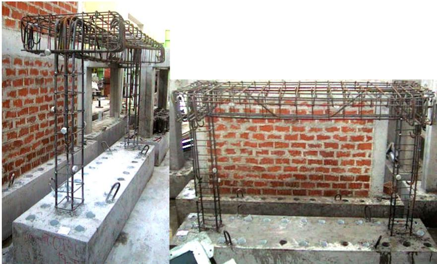
**Figure 3.4:** Reinforcement details of the frame
