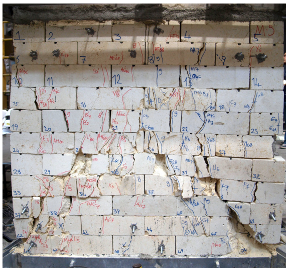
Figure C.182 : Southern face of M-50-CP after 2.0% drift ratio.
