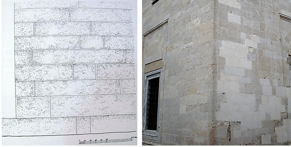
Figure 2.5 : Finely cut stone ashlar with dry joints (drawing by Tayla, 2007).
