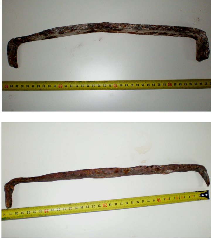
Figure 4.15 : Original cramps from Edirne II. Bayezid Mosque.
