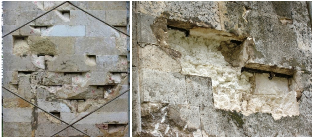
Figure 2.14 : Cramps in the Edirne II. Bayezid Mosque (Kolay, 2009).
