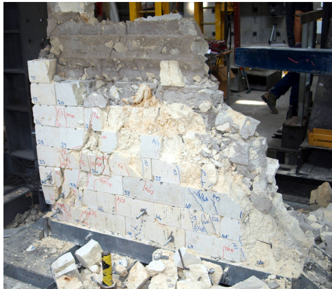
Figure C.185 : Damage on the outer and inner leaves, M-50-CP.
