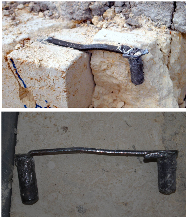
Figure C.55 : Bending of the cramps, M-50-C.
