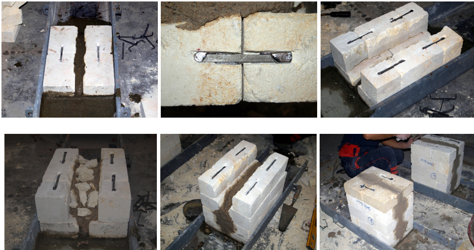
Figure 4.48 : Construction steps of the multi-leaf prisms.
