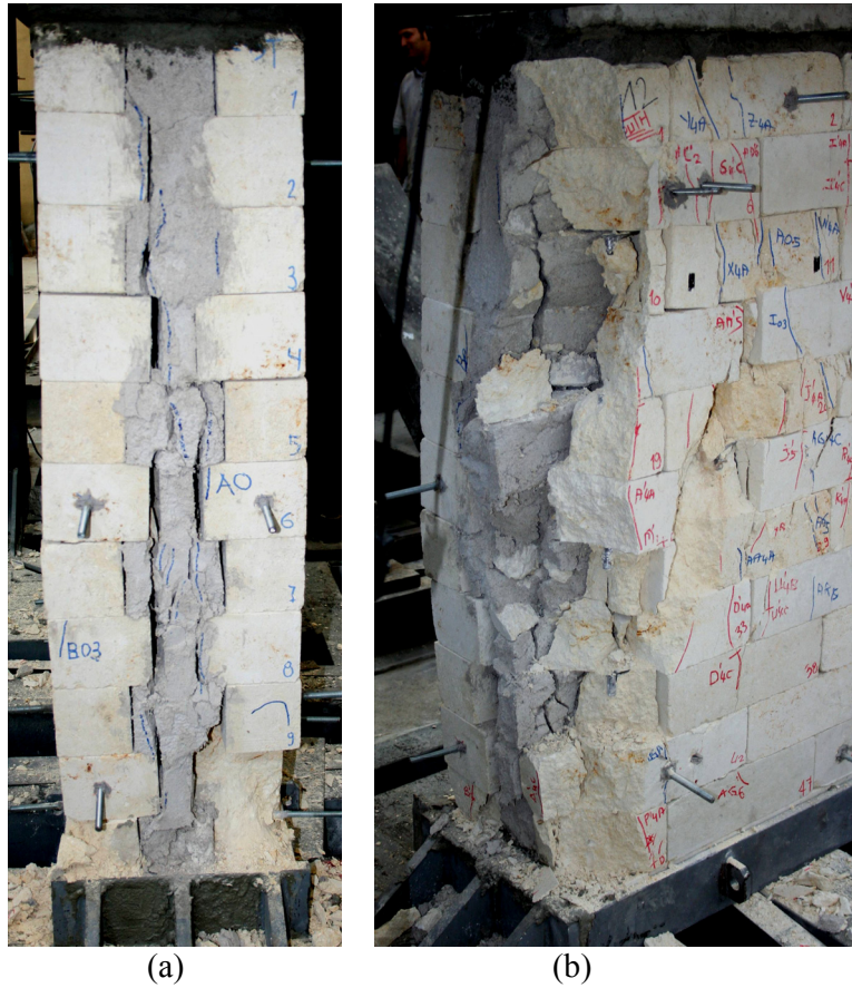
Figure C.102 : (a) East and (b) West faces of M-100-C after the test.
