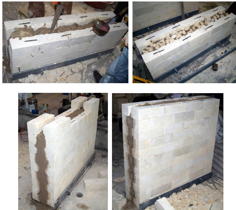
Figure 3.9 : Construction of the rubble core.
