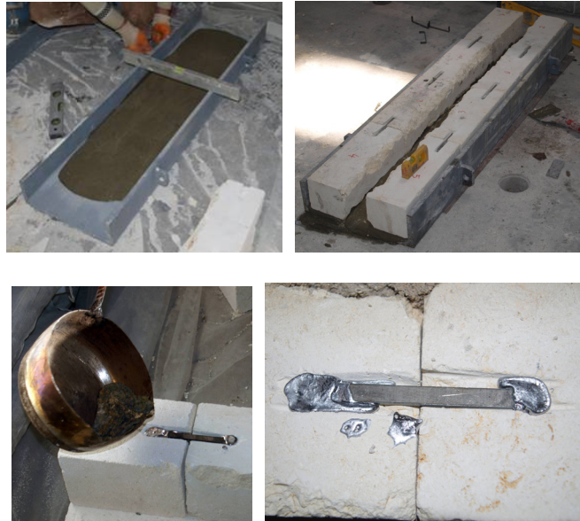
Figure 3.8 : Construction of the outer leaves.
