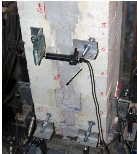
Figure C.33 : Cycle 4a, vertical cracks between the inner and outer leaves, M-50-C.
