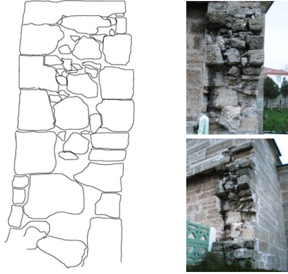
Figure 2.11 : Wall section from Havsa Sokullu Külliyesi.
