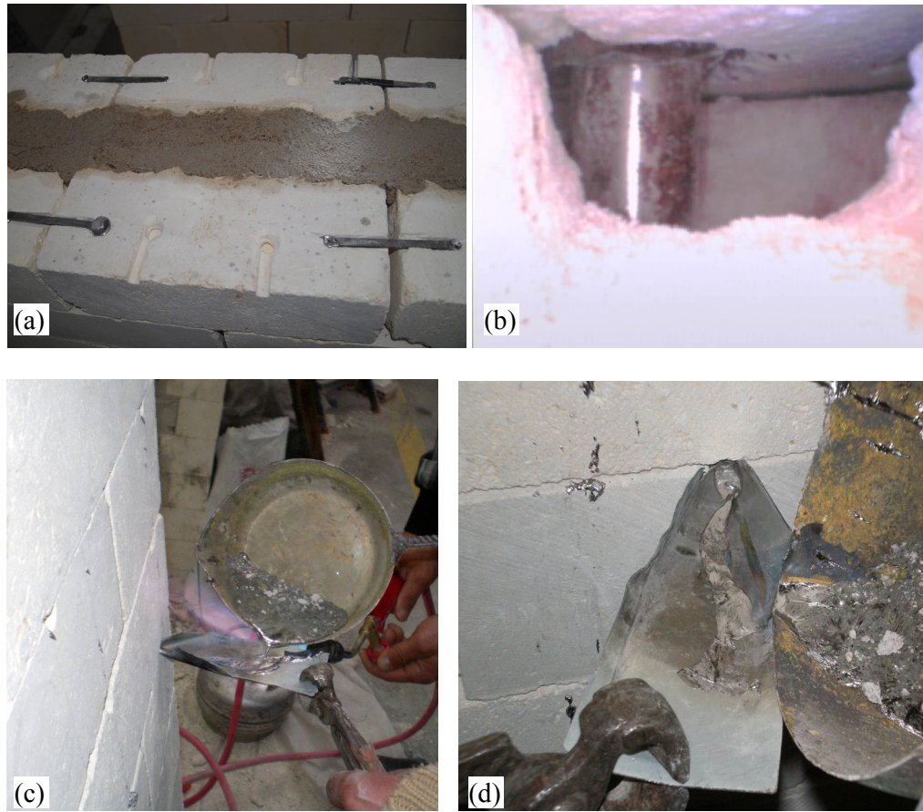
Figure 3.11 : Installation of the pins.
