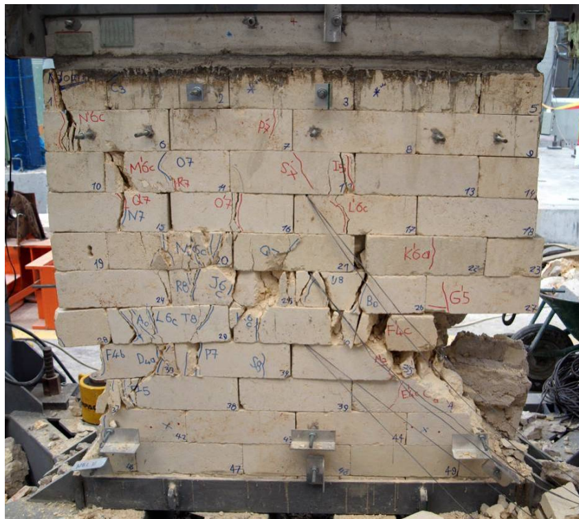
Figure C.15 : Cycle 9, North face of M-25-C after 2.0% drift ratio.
