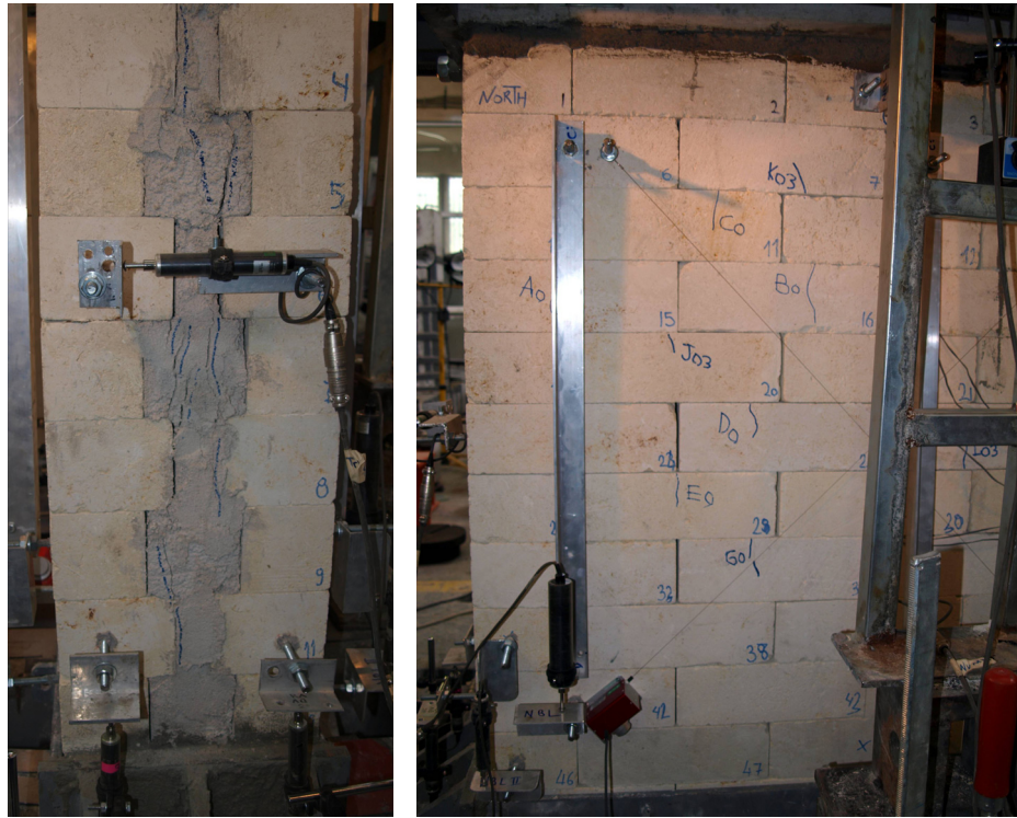
Figure C.84 : Observed damage during the axial loading of M-100-C specimen.
