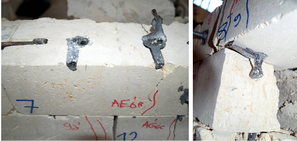
Figure C.184 : Damage in the vicinity of pins, M-50-CP.
