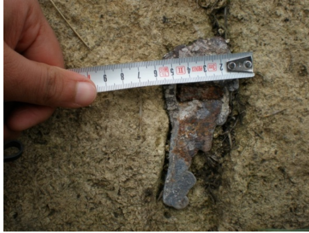
Figure 2.13 : Cramp fixed with molten lead (from ruins of Edirne Palace).
