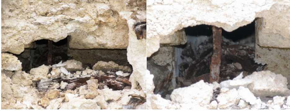
Figure 2.15 : Pin used in the Edirne II. Bayezid Mosque (Kolay, 2009).
