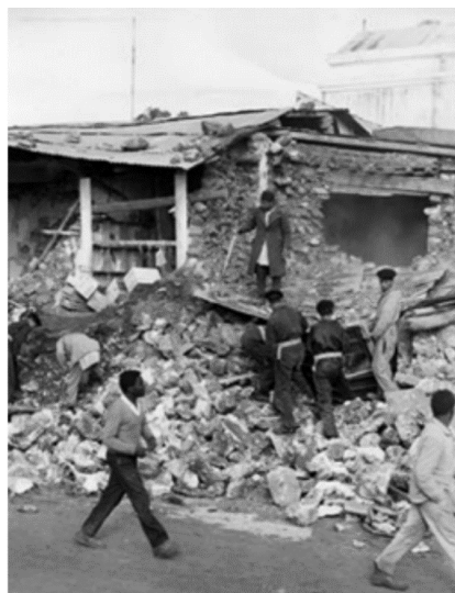
Figure 2.7 : An example of damage to a rubble stone and mud house (Sulfium Forum , 2010).
