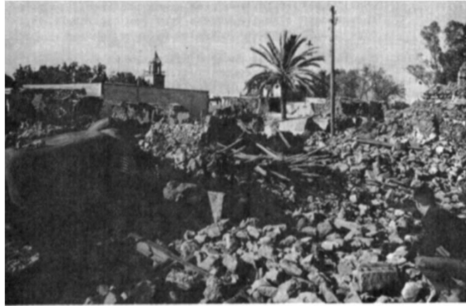
Figure 2.6 : Amid the ruins of a once thriving neighborhood lays a pile of rubble, with a collapsed roof made of wooden beams in the middle of it all. Even though the destruction is obvious, some structures, with sturdy frames and reinforced concrete columns, are still standing - though they've taken a beating from the force of nature (Minami, J.K., 1965).
