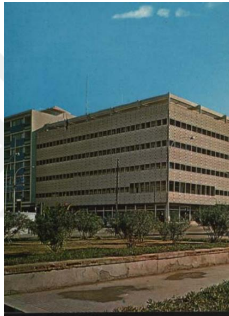
Figure 3.9 : Administrative buildings (Tošković Dobrivoje, 2006)
