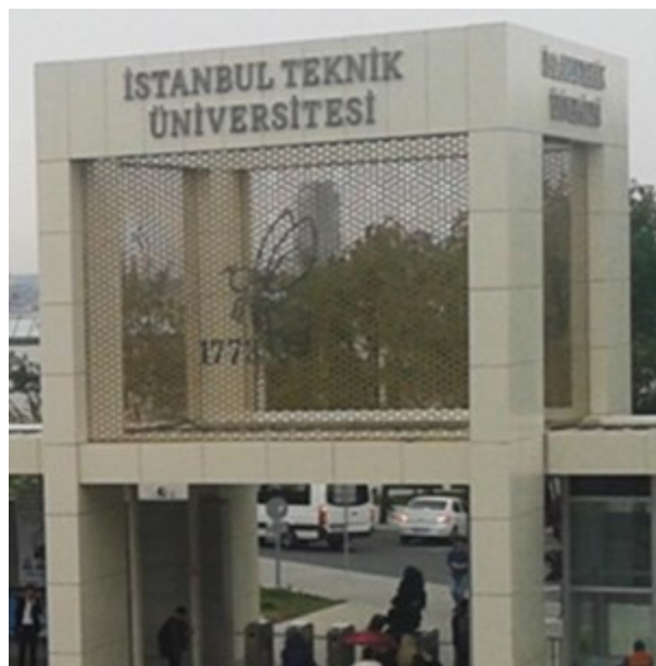
Figure 1.3 : Moire pattern on ITU entrance due to the honeycomb structure.
