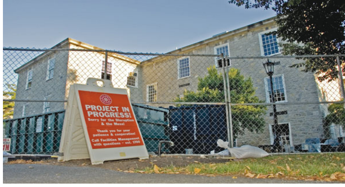
Şekil 4.7: Dickinson University Alt House Hall (Url-48).
