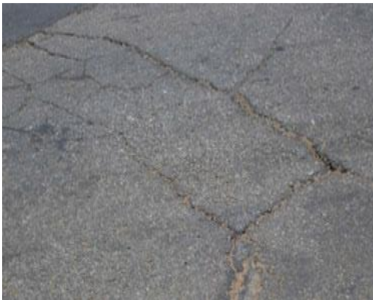
Block Crack
