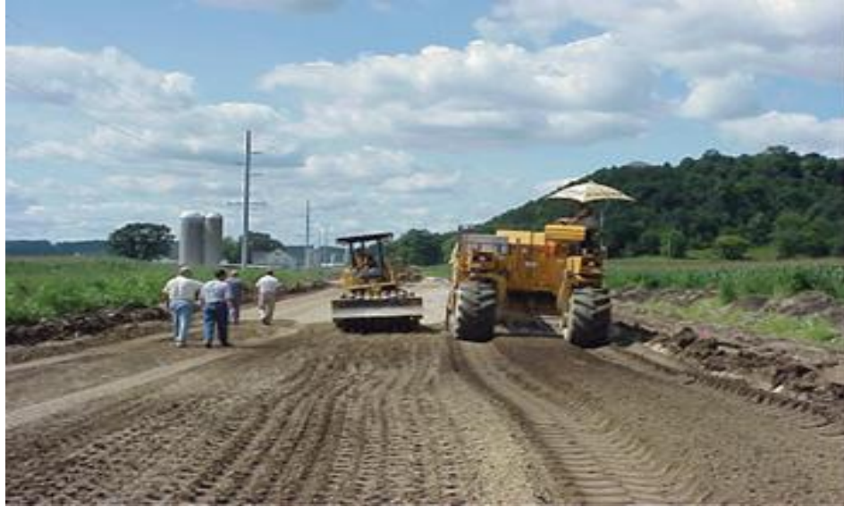
Figure 3.6 : Mixing and shaping of fly ash stabilized soil ( www.fhwa.dot.gov ).
