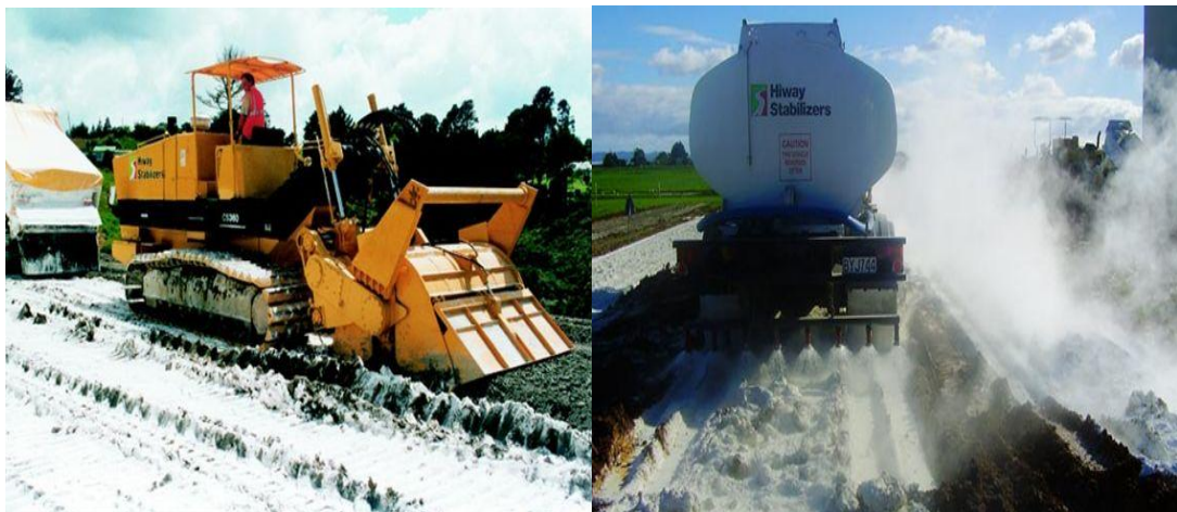
Figure 3.7 : Lime stabilization in a road construction ( http://www.hiwaystabilizers.co.nz )
