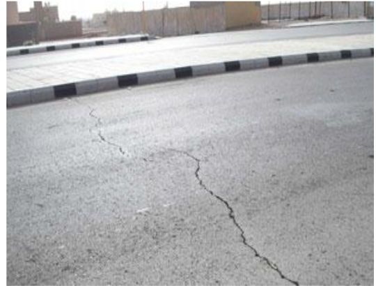
Transverse Crack
