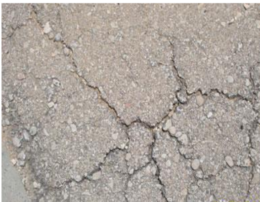
Spot Ridge Cracks
