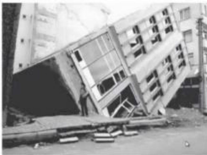
Figure2.2: Kocaeli Earthquake in 1999 (EERC library of UC Berkeley)
