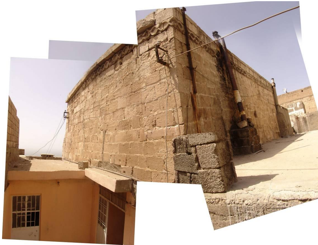
Figure 2.105 : The southeastern corner of the IIM6 volume.
