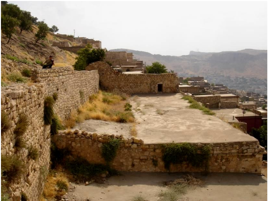
Figure 2.209 : The roof terrace of the IVU3-4-5 series – looking east.
