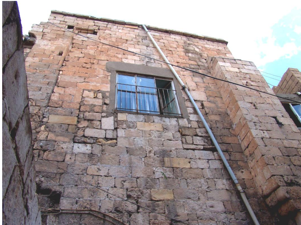
Figure 2.100 : The portal trace, window traces, an buttress/latrine on the southern face of the IIL6/IIM6 mass.
