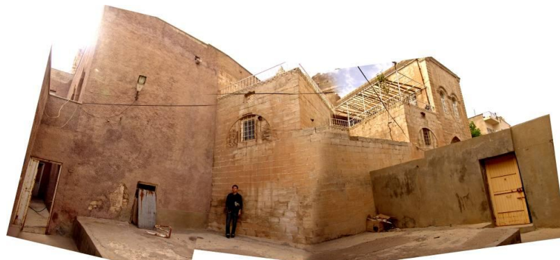
Figure 2.45 : Panoramic view of the southeastern entrance courtyard – starting from the passageway to the west (left) to the eastern independent house and the entrance to the courtyard on the east (right).
