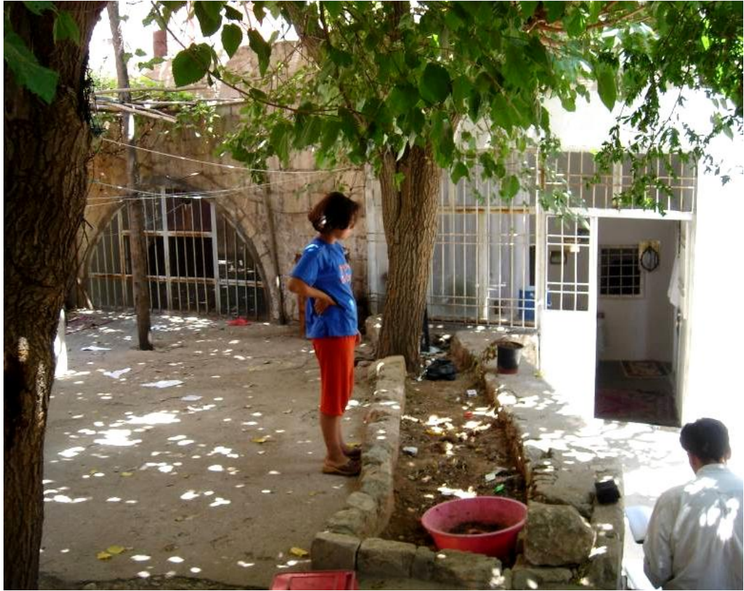
Figure 2.289 : The western exterior wall of the VM L 5 and VM L 7 volumes standing partially submerged within the courtyard.
