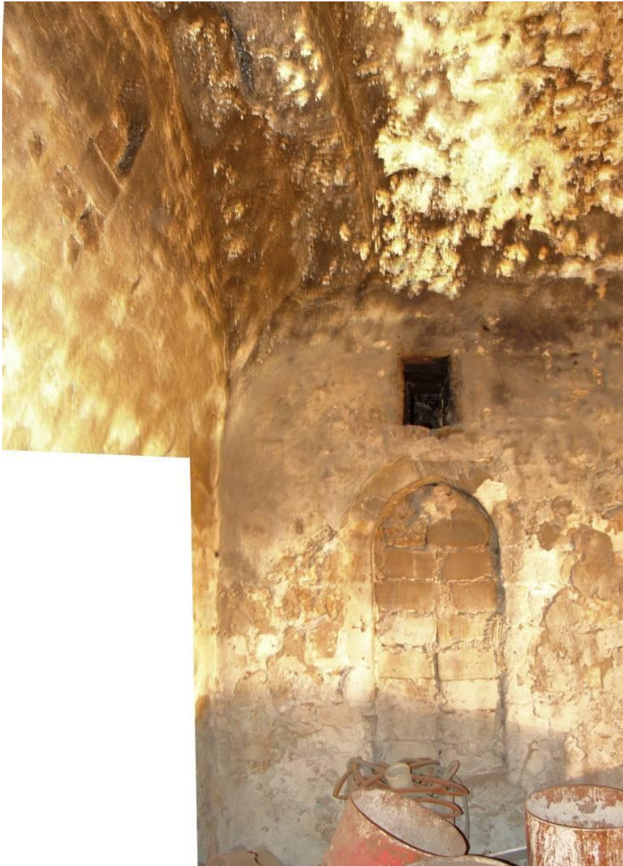
Figure 2.322 : The northern window of IL5/zaviye volume opening to the IL4 volume – seen from IL4.
