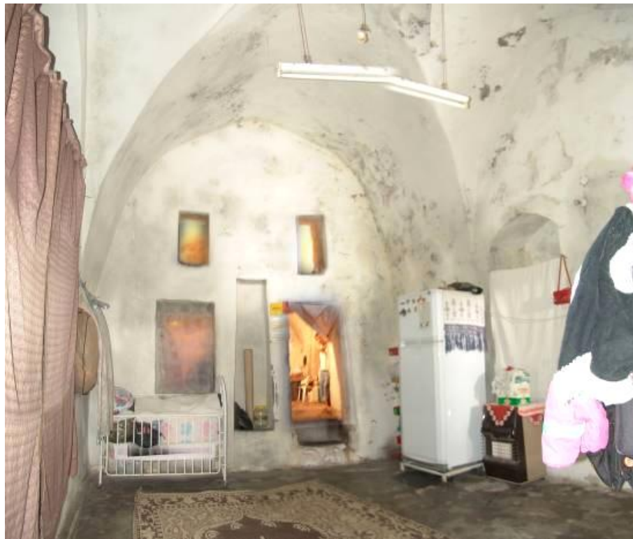
Figure 2.125 : The IIL14 volume opening to IIL15 – looking north.
