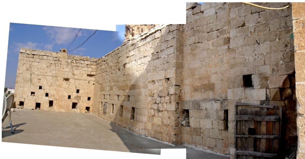
Figure 2.383 : The IIIMtx terrace – looking west.
