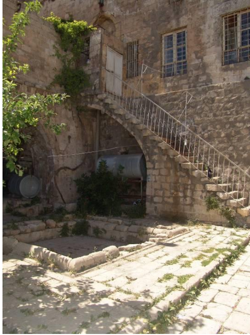
Figure 2.142 : The northeastern corner of the central courtyard and the staircase leading to the upper level.
