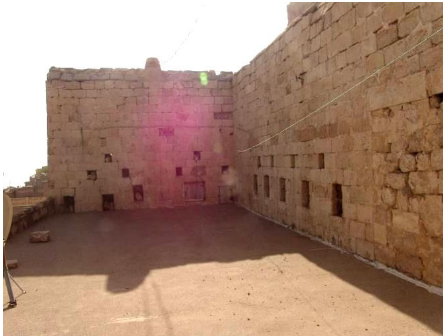
Figure 2.191 : The IIIMtx terrace – looking west.
