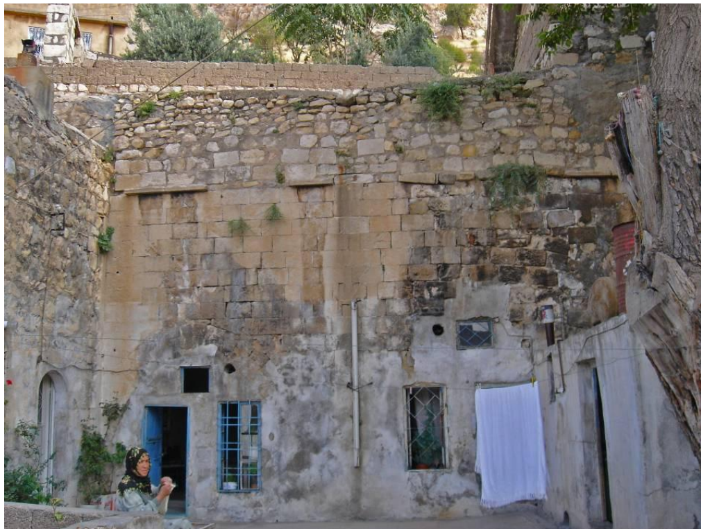
Figure 2.30 : The living units opening to the terrace by two arches that are seen to have been closed by stone walls.
