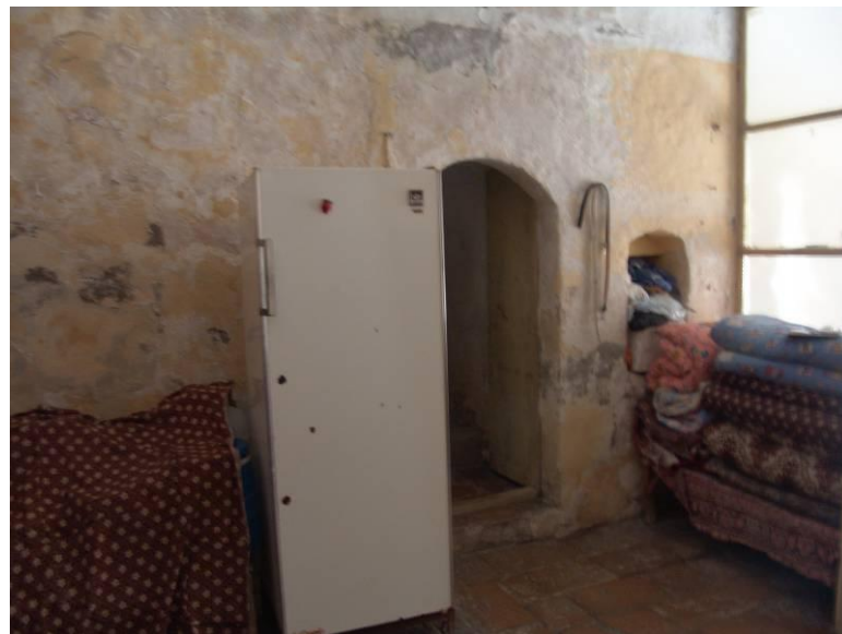
Figure 2.215 : The eastern wall of the IVU7 volume/aiwan and the opening leading to IVU9.
