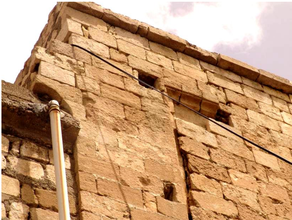
Figure 2.101 : Detail of the portal trace.
