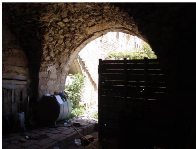
Figure 2.143 : The arch of the IIM13 aiwan volume opening to the central courtyard.
