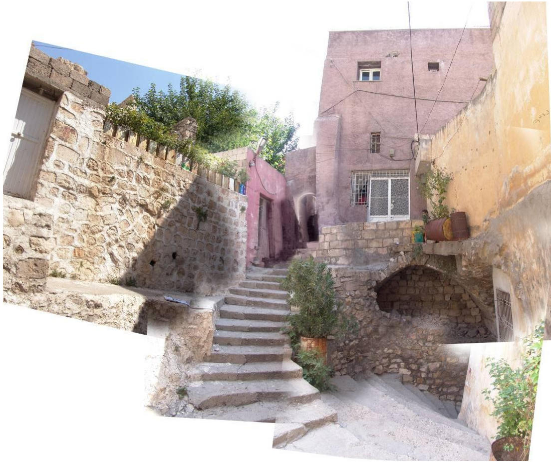
Figure 2.81 : The collapsed IIL2 volume the main entrance to the internal street – looking west with the internal street stepping up to the entrance to the Sincar wing and the eastern entrance of Block-V.
