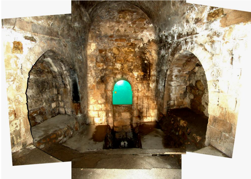
Figure 2.375 : The Altunboğa Fountain – looking north.
