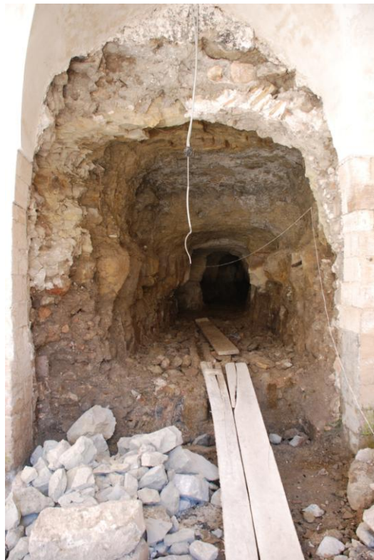
Figure G.4 : The first leg of the tunnel – looking north.
