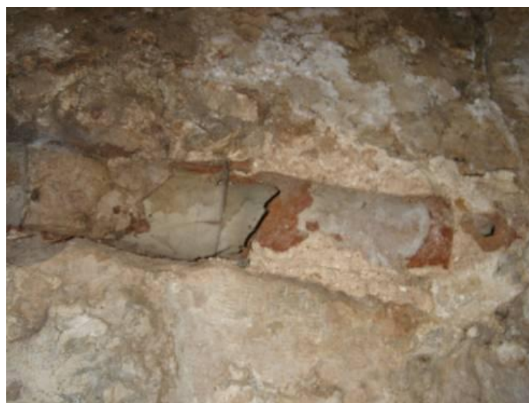
Figure 2.156 : The terracotta water pipe within IIM14.
