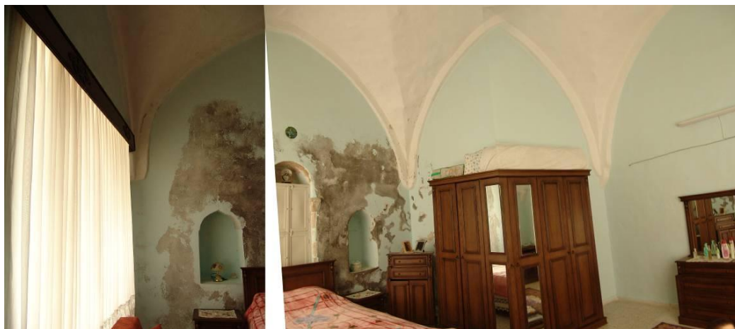
Figure 2.276 : Panoramic view of the VM8 volume showing its western wall.
