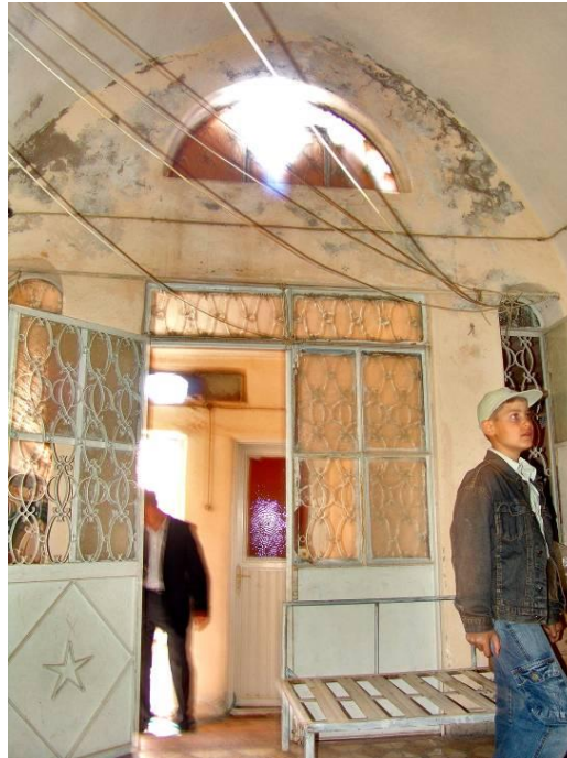
Figure 2.355 : The eastern wall/entrance of the IM8 volume.
