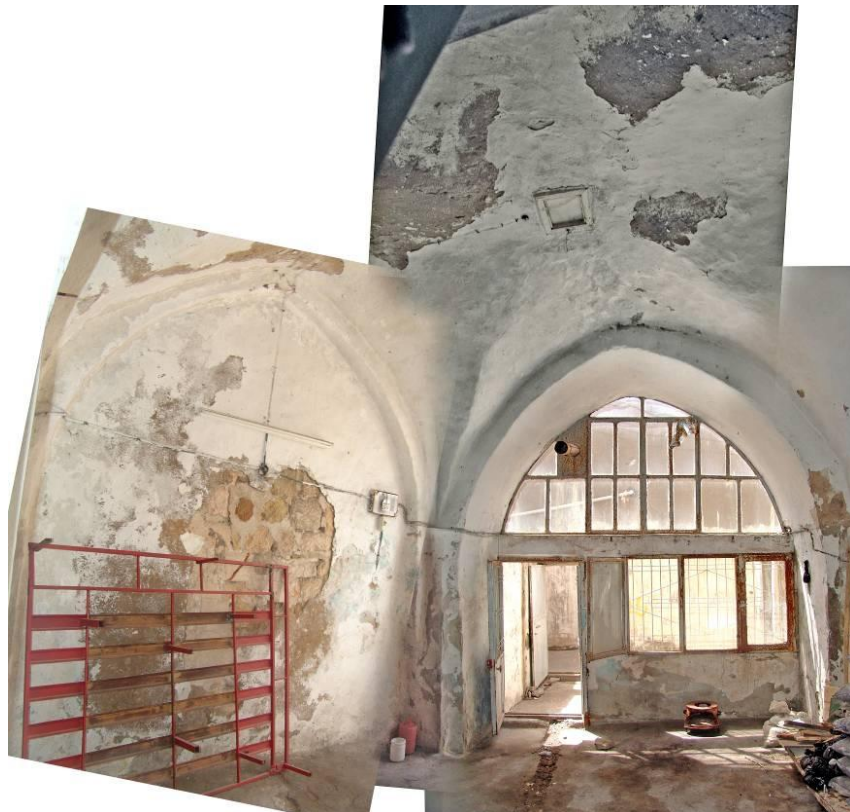
Figure 2.113 : The IIL8 volume opening to the Pınarcık street – looking south.
