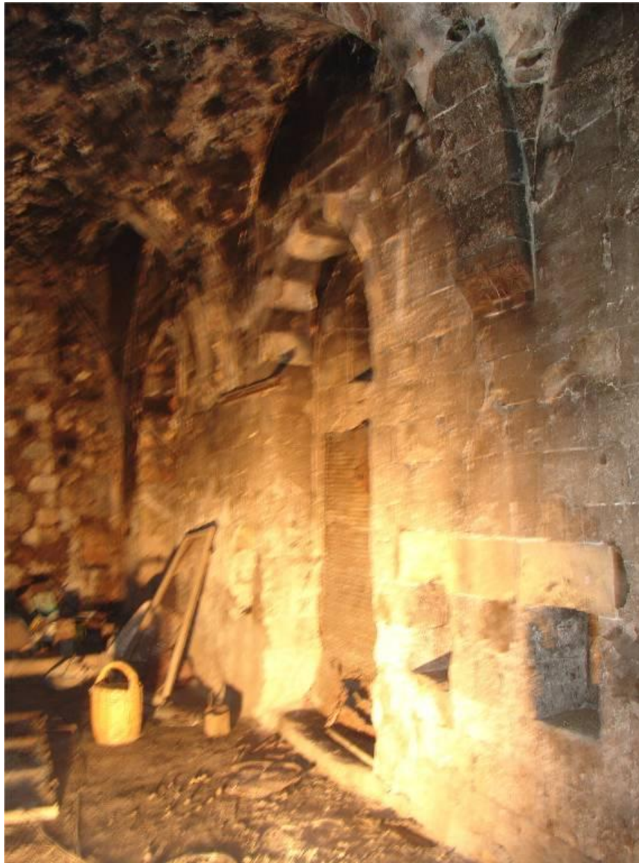
Figure 2.56 : The northern wall of IL5 – looking west.
