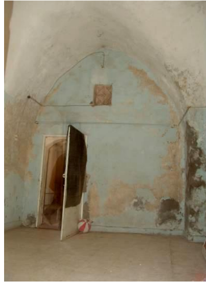
Figure 2.352 : The IM7 volume – looking west.
