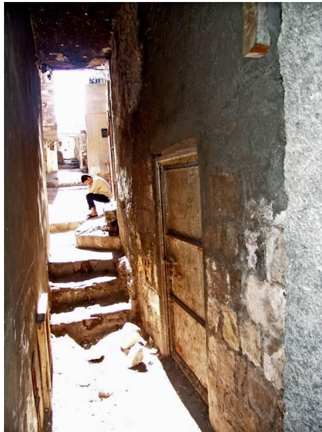
Figure 2.302 : The eastern end of the Pınarcık Alley, and the entrance doorway of the IL3 volume.
