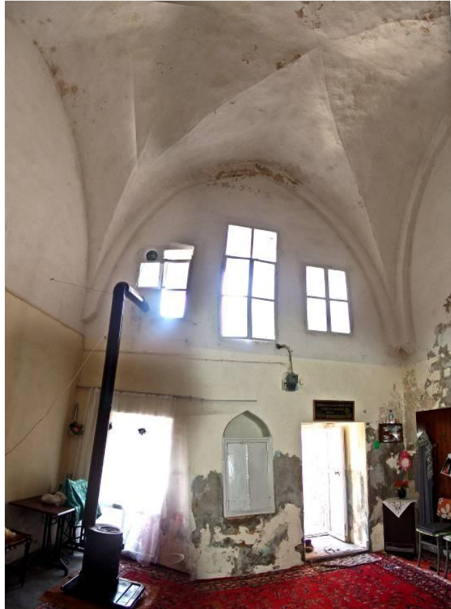
Figure 2.220 : The groin vault and southern interior wall of the IVU10 volume.
