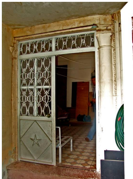
Figure 2.356 : The entrance of the IM8 volume seen from the outside.
