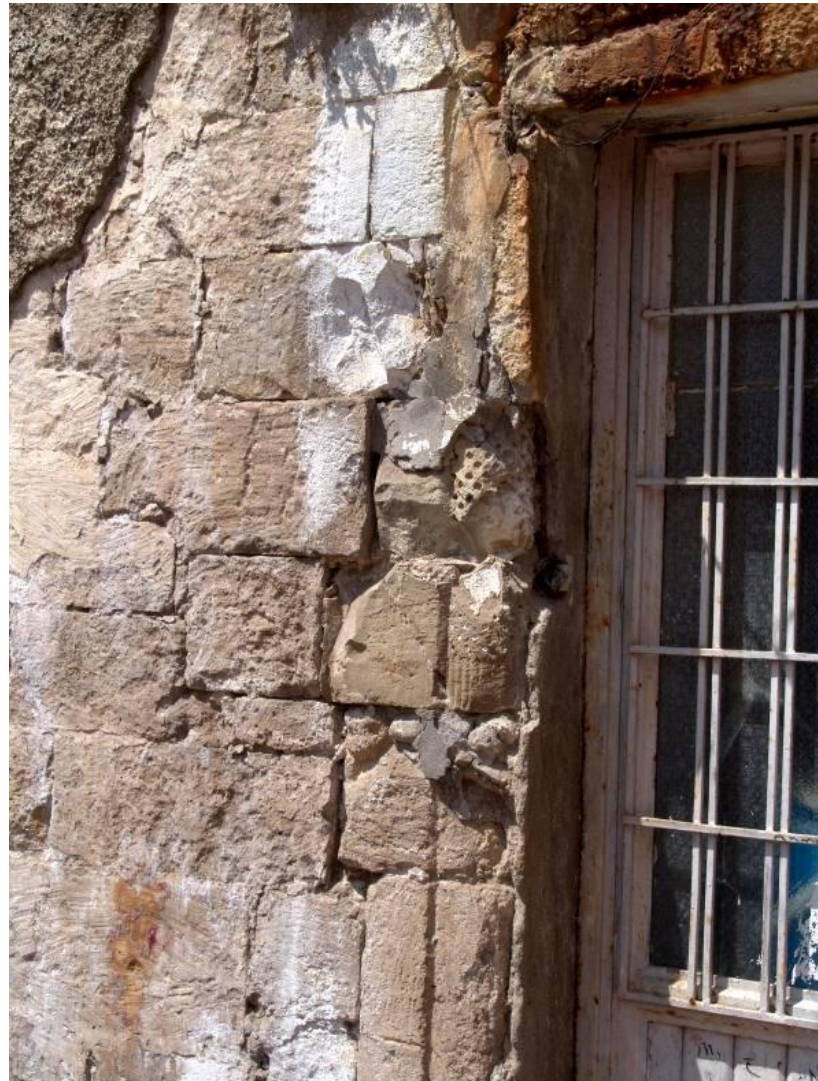
Figure 2.152 : Detail of the IIIM1 entrance doorway.
