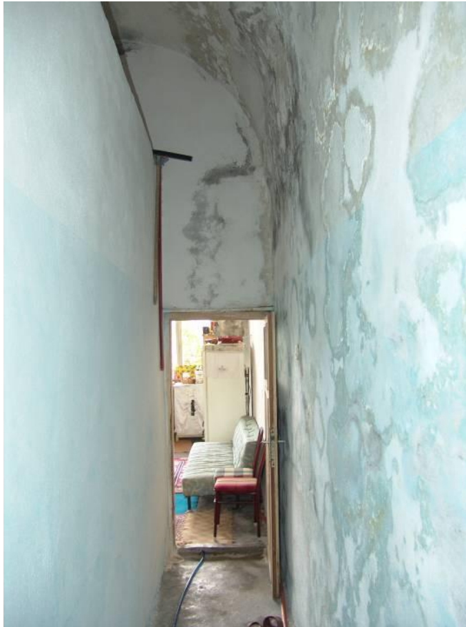
Figure 2.168 : The southern wall of the IIIL4 volume.
