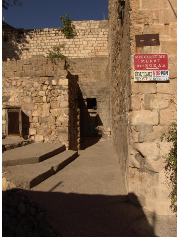
Figure 2.368 : The building block holding the Altunboğa Portal remains, and the northwestern corner of the IIIIL7 volume – looking east.
