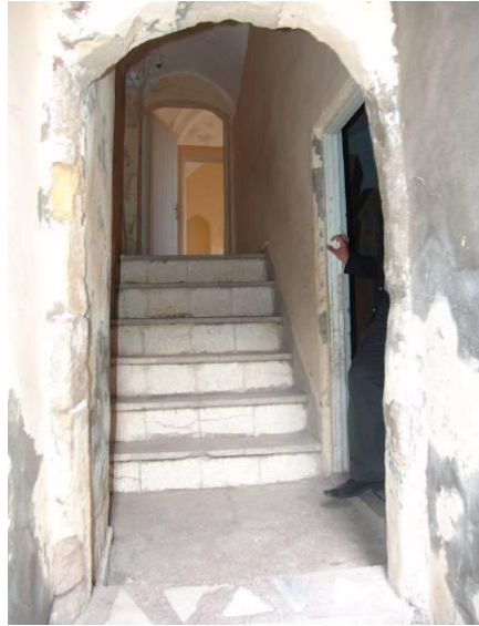
Figure 2.361 : The entrance to the IM6 volume and the staircase leading up to the IM10 volume – looking east from the eastern end from the internal street/Block-I's northern passageway.
