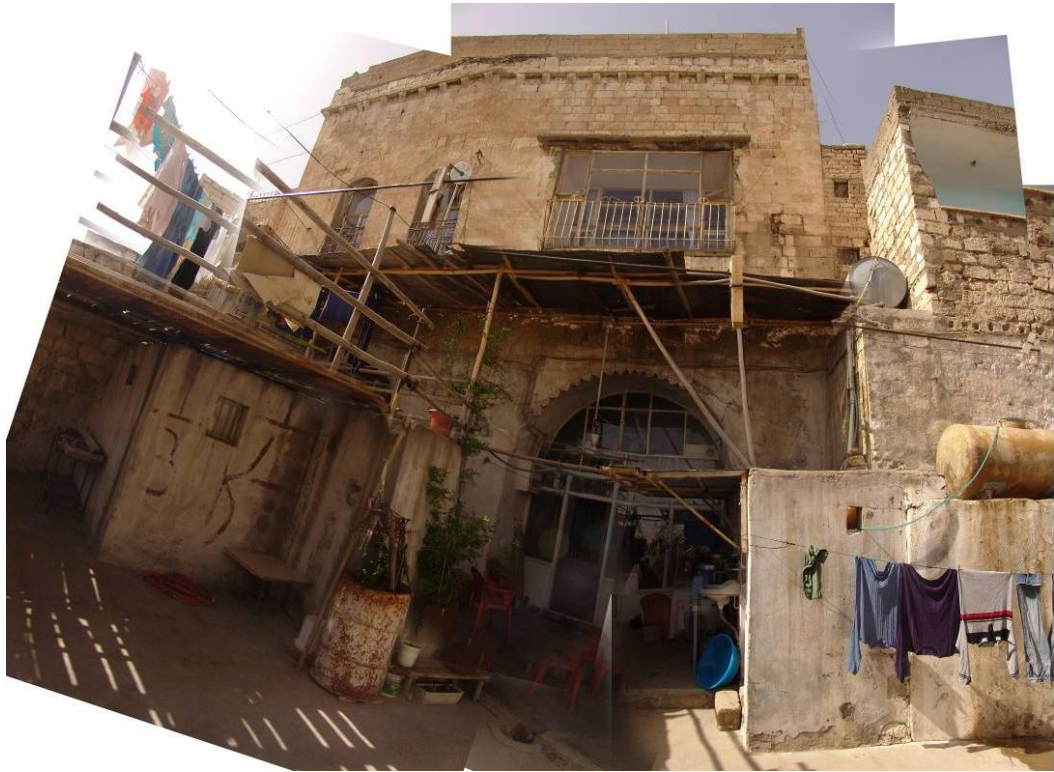
Figure 2.163 : The round arched opening of IIIL1 opening to the Pınarcık courtyard, and the southern face of Block-III.
