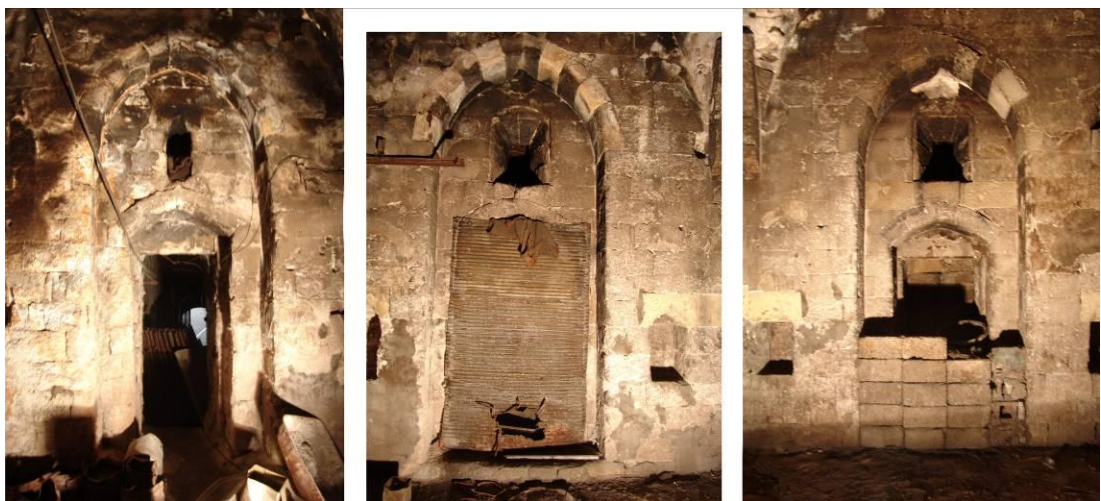
Figure 2.324 : The opening systems on the southern wall of the IL5/zaviye volume.
