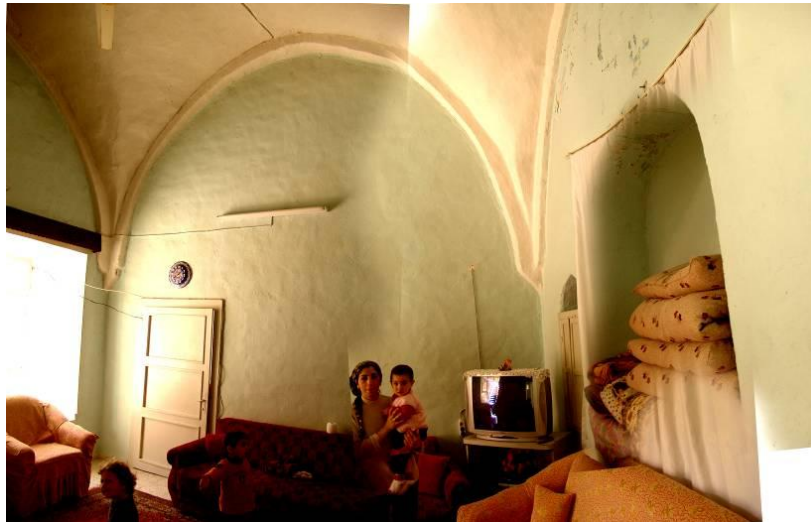
Figure 2.275 : The VM8 volume and its later added internal subdivision wall – looking west.
