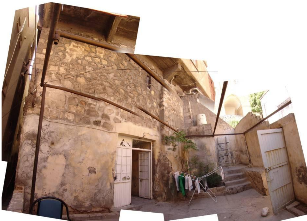
Figure 2.320 : The entrance to the IL7 volume – looking northwest from its terrace.
