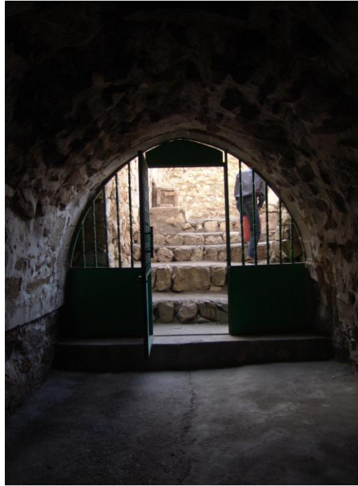
Figure 2.370 : The vaulted entrance to the passageway leading to the Altunboğa Fountain – looking south from within.
