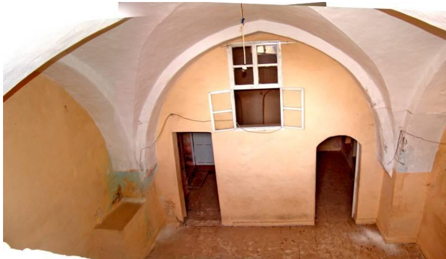
Figure 2.273 : The IM11 volume seen from its top window opening to Block-V – seen from the VMt3 terrace.
