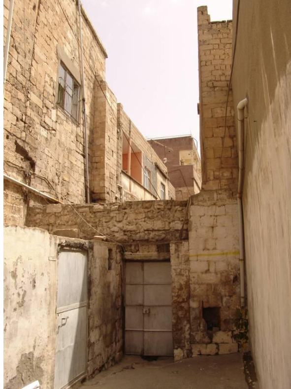
Figure 2.14 : Middle part of the Pınarcık Street - looking east.
