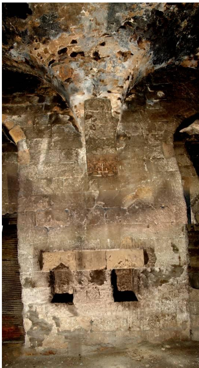
Figure 2.332 : The muqarnased niche (right) on the southern wall of the IL5/zaviye volume.
