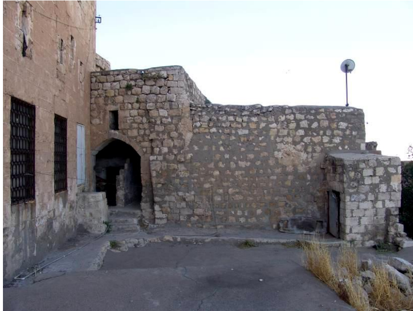
Figure 2.205 : The entrance to the eastern upper level terrace and its latrine – looking east.
