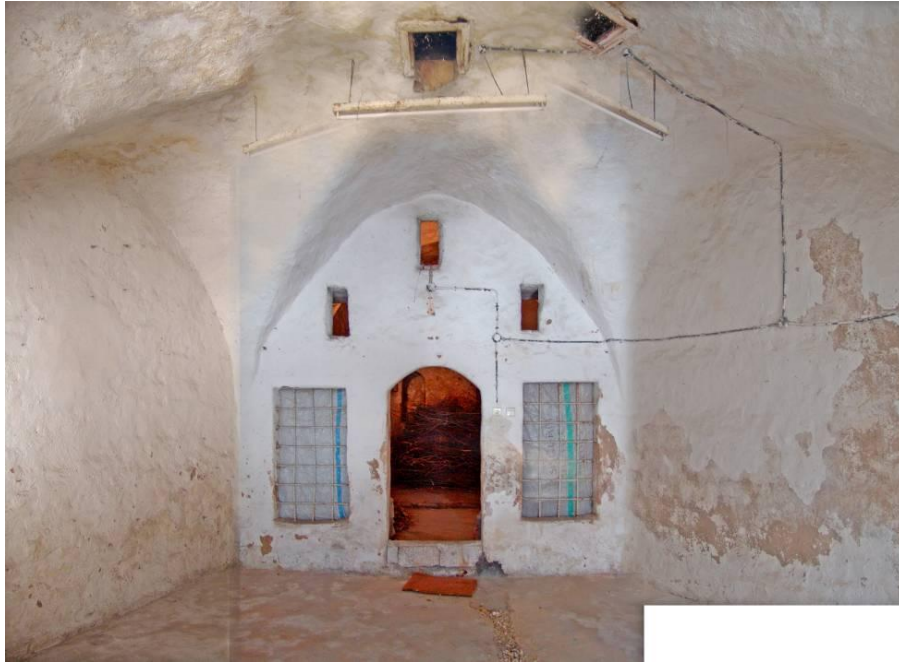
Figure 2.115 : The IIL8-9 volume opening to IIL 10-11 – looking north.
