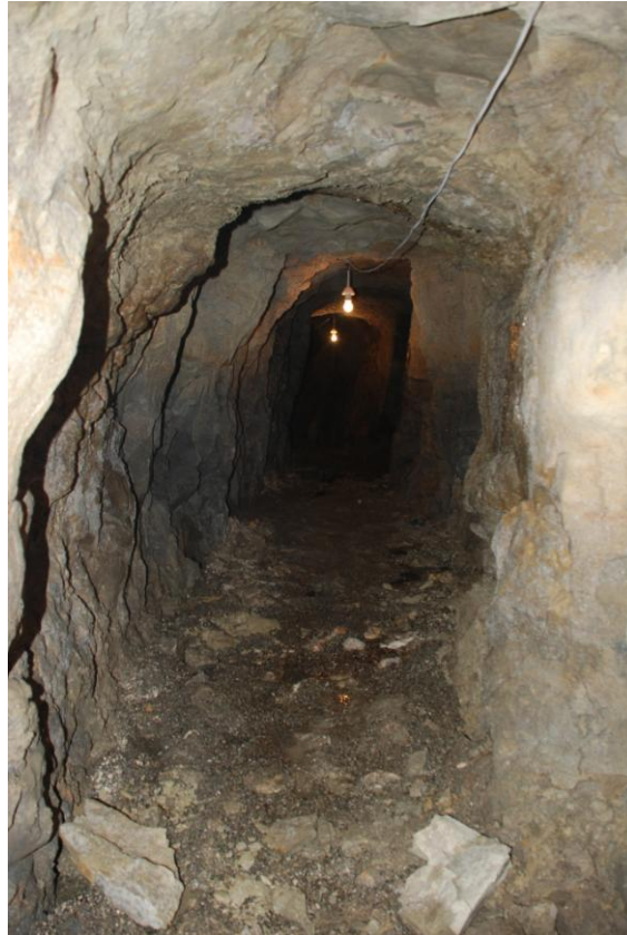
Figure G.7 : Inside the first leg of the tunnel – looking north.
