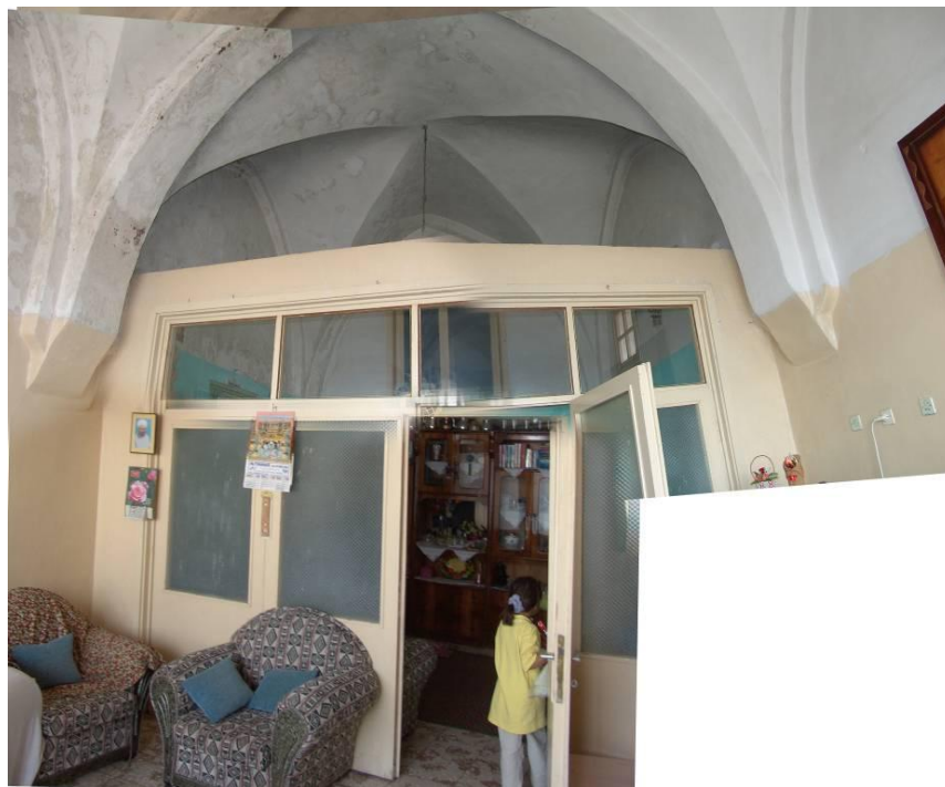
Figure 2.172 : The arch-vault system of the IIIM8-10 volumes – looking north from IIIM8.
