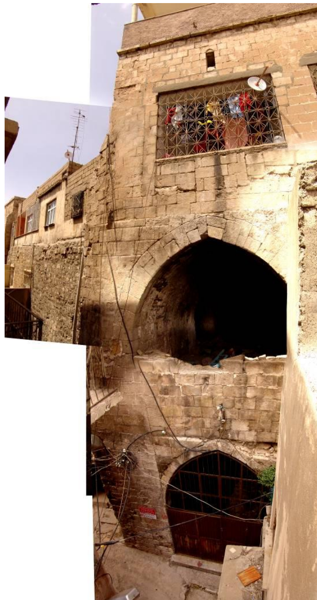
Figure 2.359 : The IM1 volume sitting above the arches of IL1 and ILL1 – seen from the terrace of the settlement's southern neighbour.
