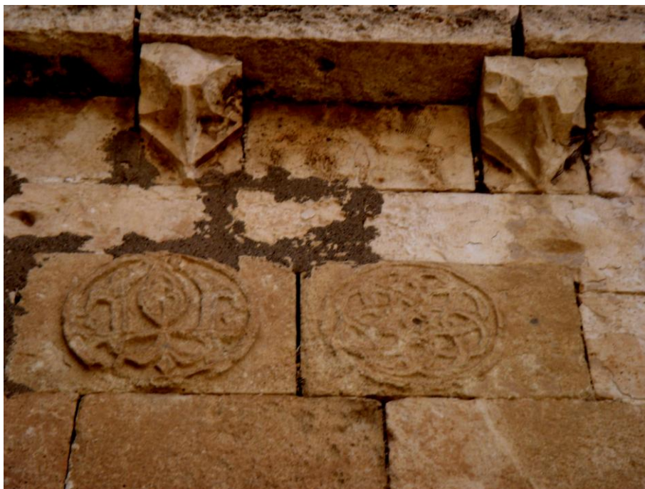
Figure 2.385 : The stone mason's seals on the eastern wall of the IIM7 volume.
