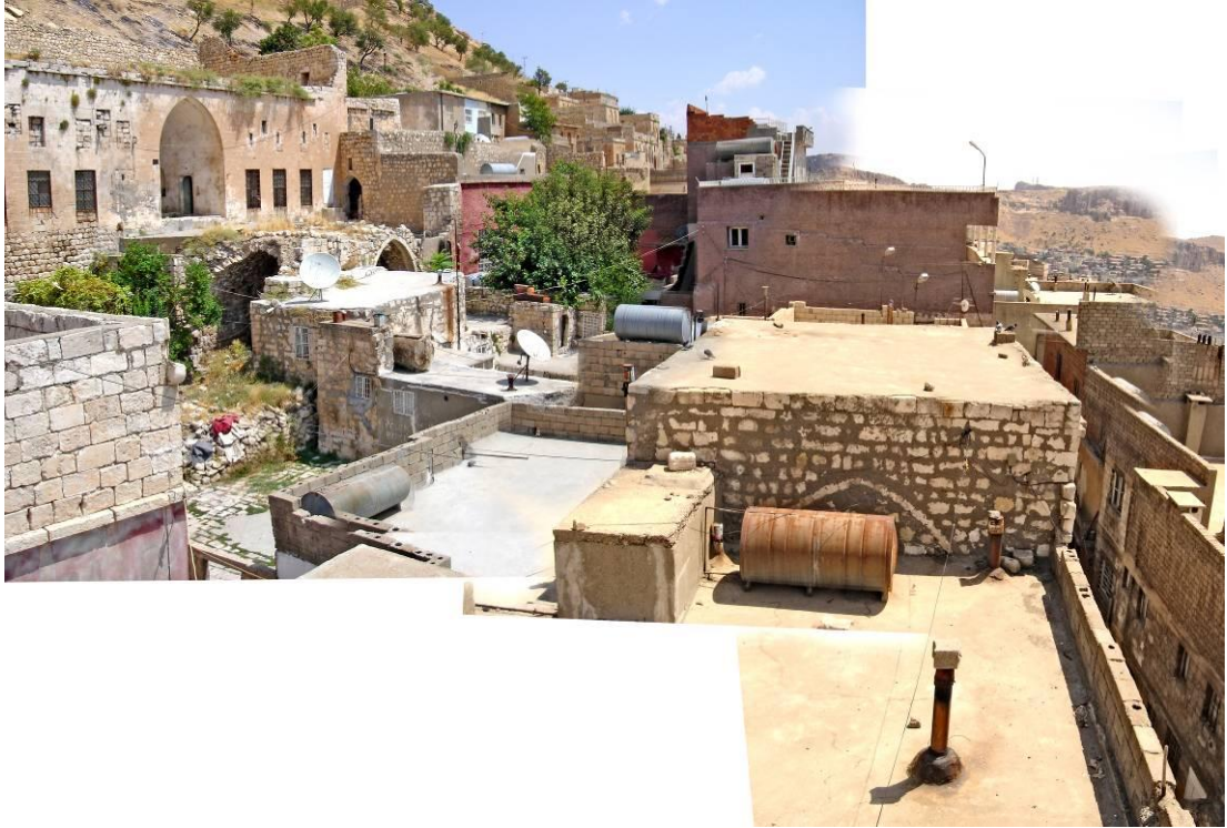
Figure 2.66 : View of Block-II and the western face of IIM6 – looking east from the terrace of IIM8.
