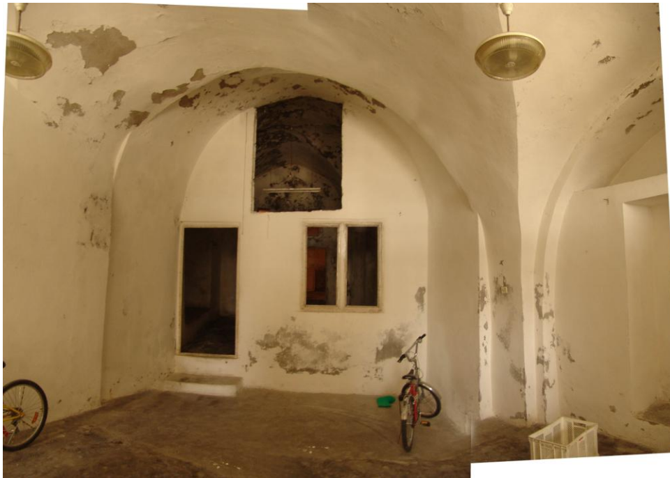
Figure 2.124 : The IIL13 volume opening to IIL14 – looking north.
