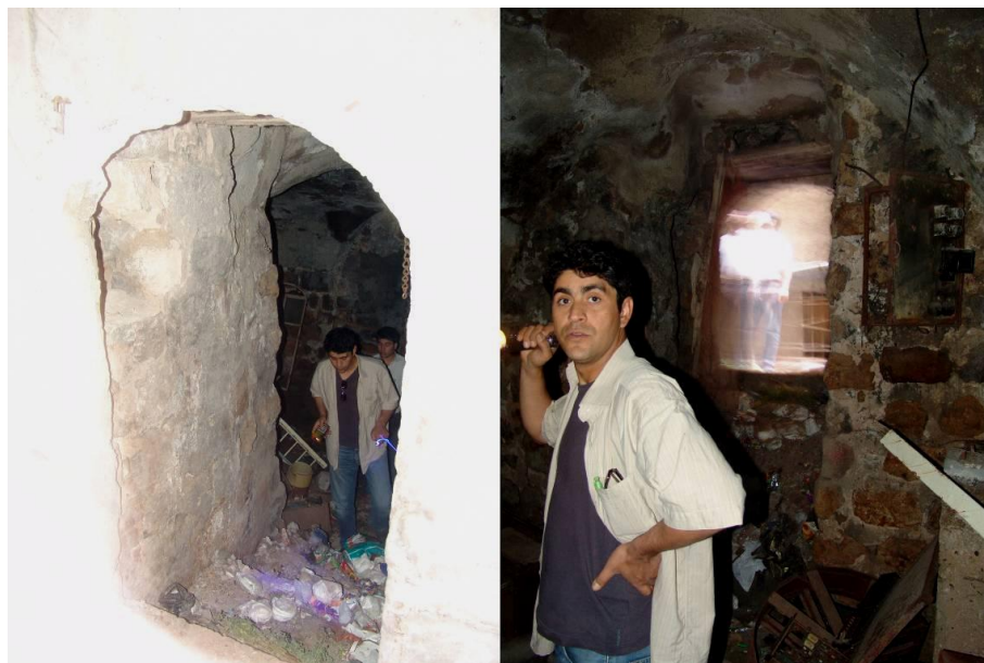
Figure 2.305 : The entrance doorway of the partially submerged the IL L 3 volume – looking south and north.
