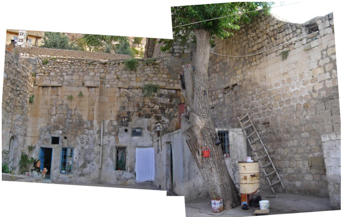
Figure 2.390 : The southern face of the residential volume over the Altunboğa fountain holding enclosed arches and the continuation of the corbel traces on the eastern face of the settlement.
