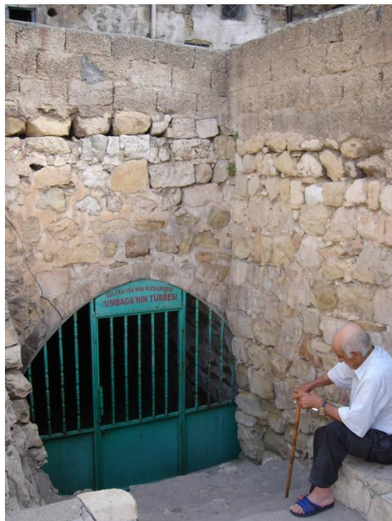
Figure 2.371 : The entrance to the vaulted passageway leading to the Altunboğa Fountain – looking north.
