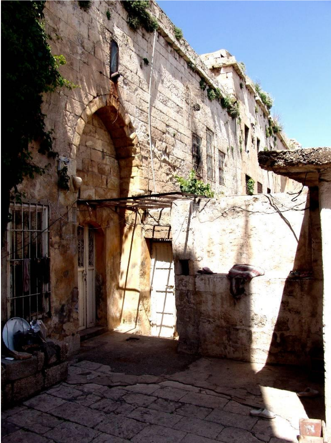
Figure 2.210 : The entrance doorway to the IVU6 volume and IVU6-11 series – looking northeast from the IIIUtW terrace.
