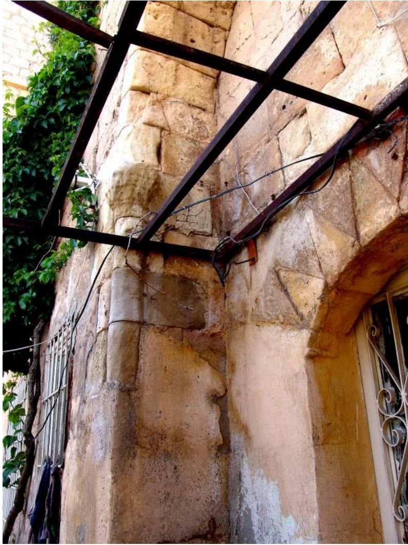
Figure 2.223 : Detail of the doorway-portal leading into the IVU6 volume.
