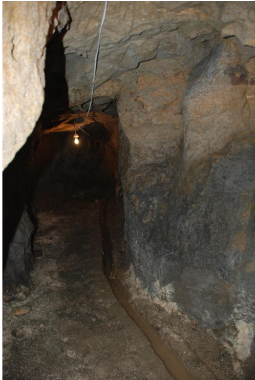
Figure G.9 : The second leg of the tunnel and the water channel on its base – looking east.
