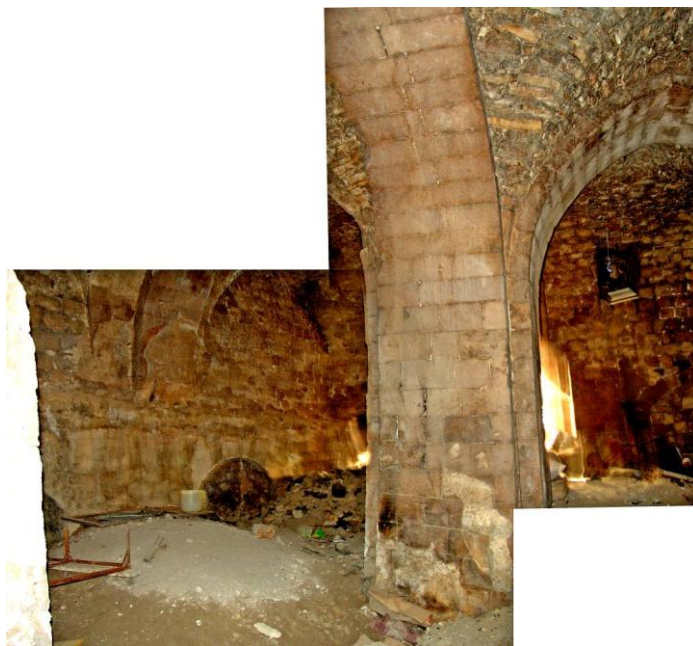
Figure 2.133 : The northern wall, the central column and the eastern wall of the IIM14 volume – looking northeast.
