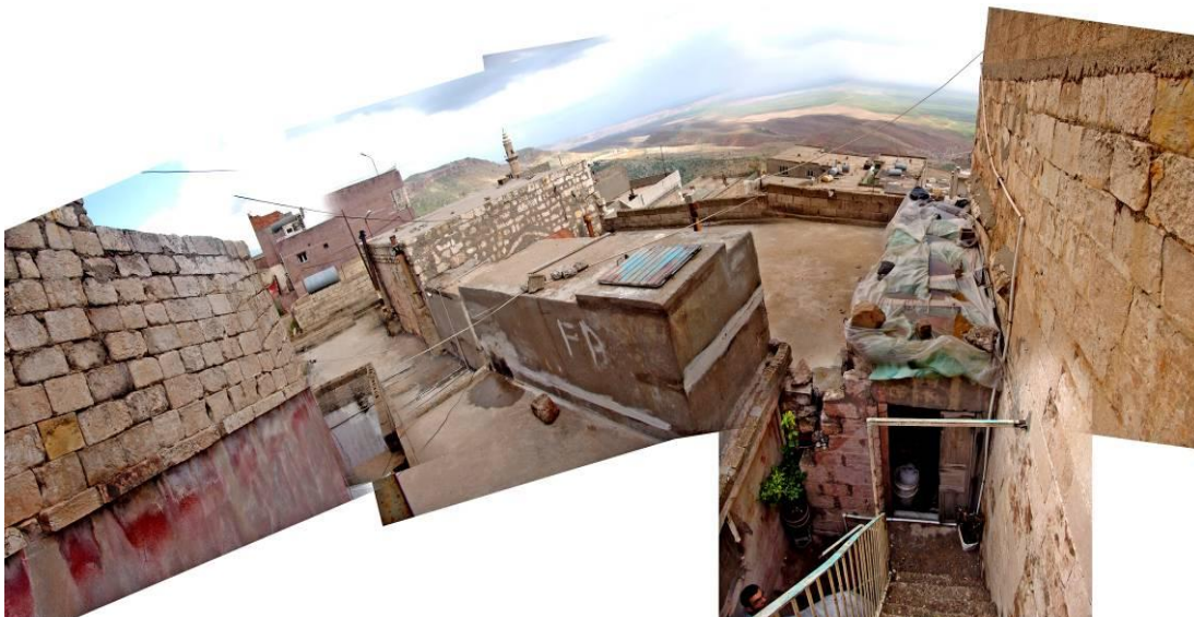
Figure 2.187 : The zone between Block-II and Block-III with the staircase rising to the Block-II terrace – looking south from the terrace level of the staircase.
