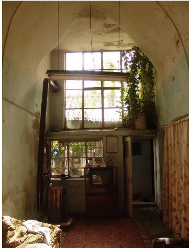
Figure 2.252 : The VM1 vault and the RC slab addition on its west.
