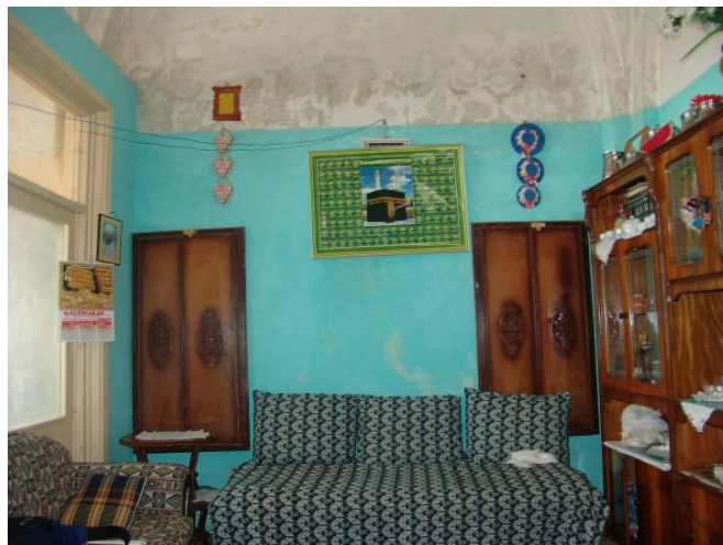
Figure 2.185 : The western wall of IIIM9 with the niches fitted with wooden cabinets.
