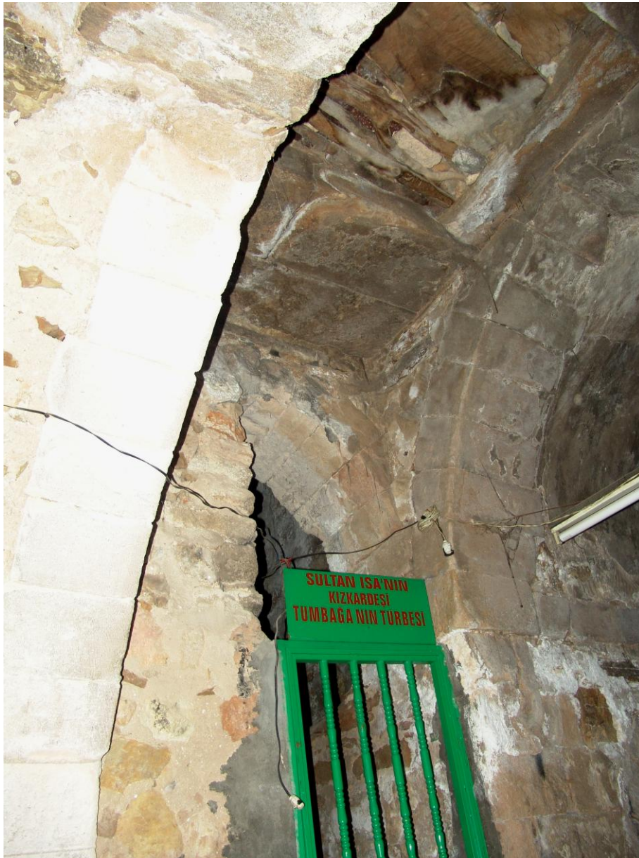
Figure 2.378 : The gate to the passageway leading west to the chamber of ‘Tumbaga’s resting place’, and the slabbed construction between the arches eighter side of its east – looking northwest.
