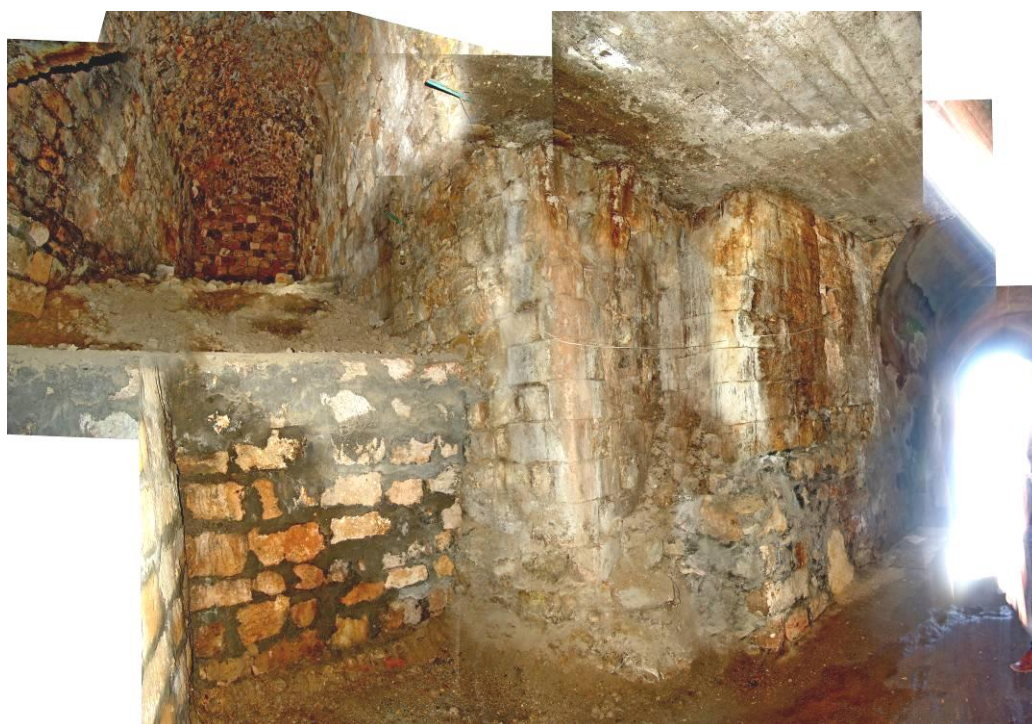
Figure 2.296 : Panoramic view showing the IL L2 volume and the eastern wall of the IL L2 volume – looking southeast.
