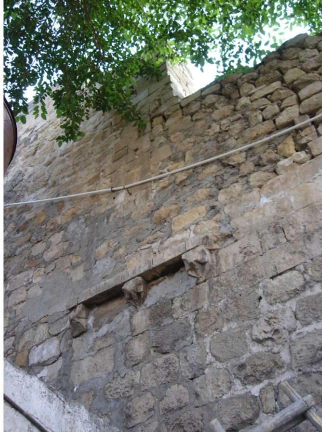
Figure 2.389 : The Corbels on the eastern face of the settlement – eastern face of IIIM4.
