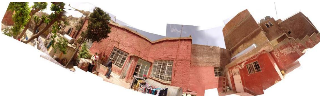
Figure 2.272 : Panoramic view of the eastern wing of Block-V; the southern faces of VM L 2 and VM8 – seen from the VMt3 terrace.
