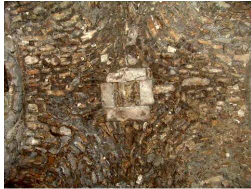
Figure 2.136 : The key stones of the IIM14 cross vaults.
