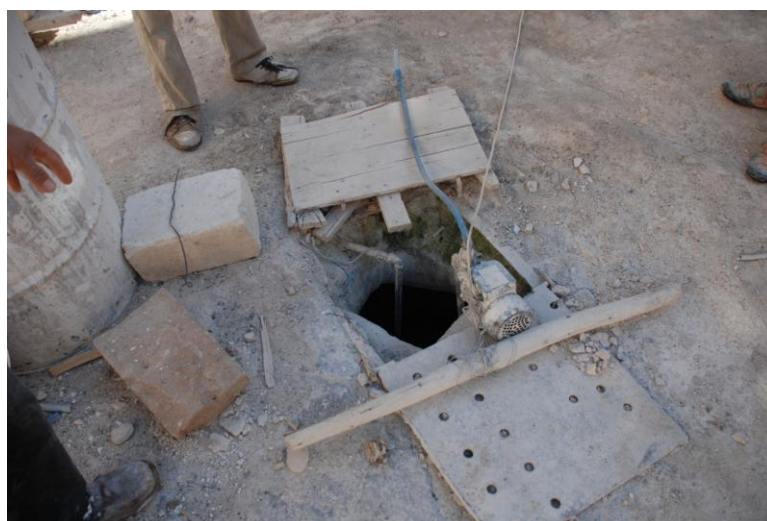
Figure G.2 : The cistern well on the han's courtyard.
