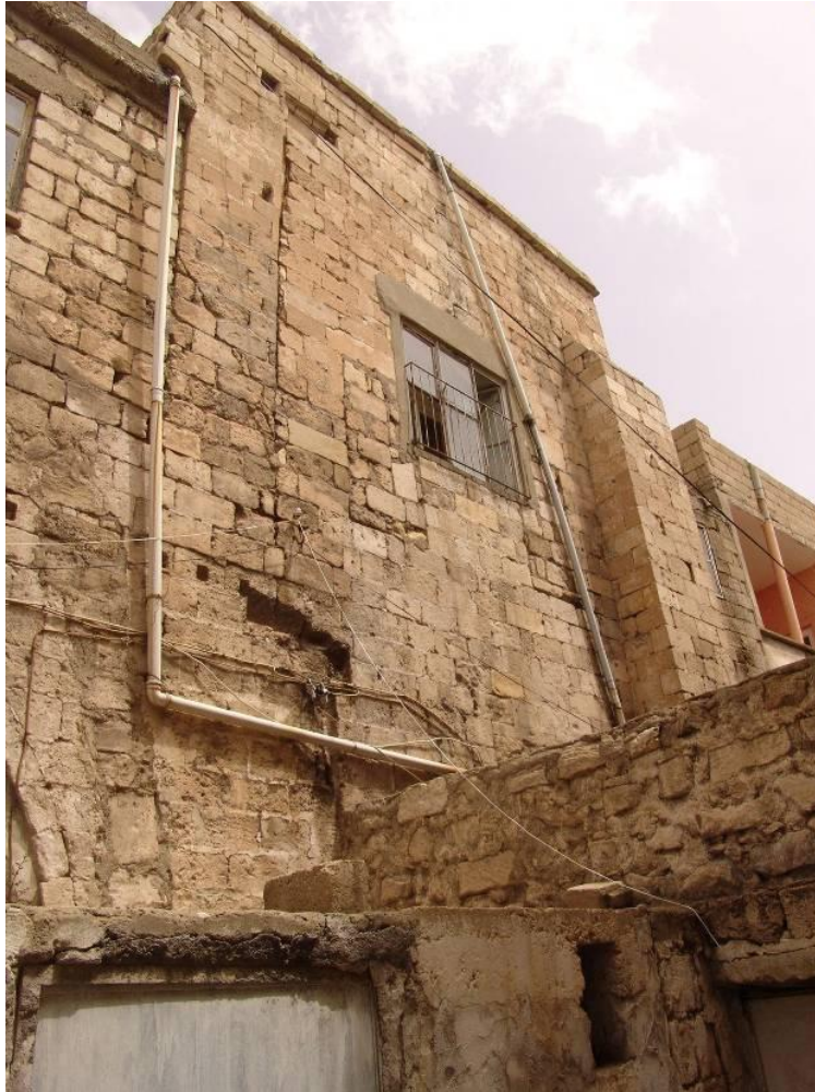
Figure 2.99 : The portal trace and butters/litrine on the southern face of the IIL6/IIM6 mass
