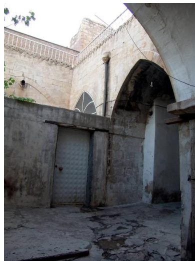
Figure 2.238 : The two southern arches of the lower courtyard of Block-VI and its added subdivision wall.
