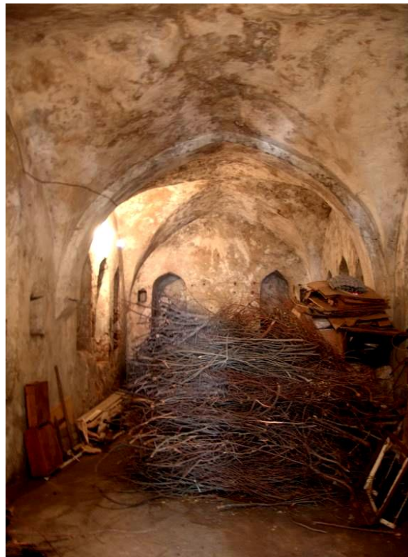
Figure 2.118 : The IIL10-11 – looking north.
