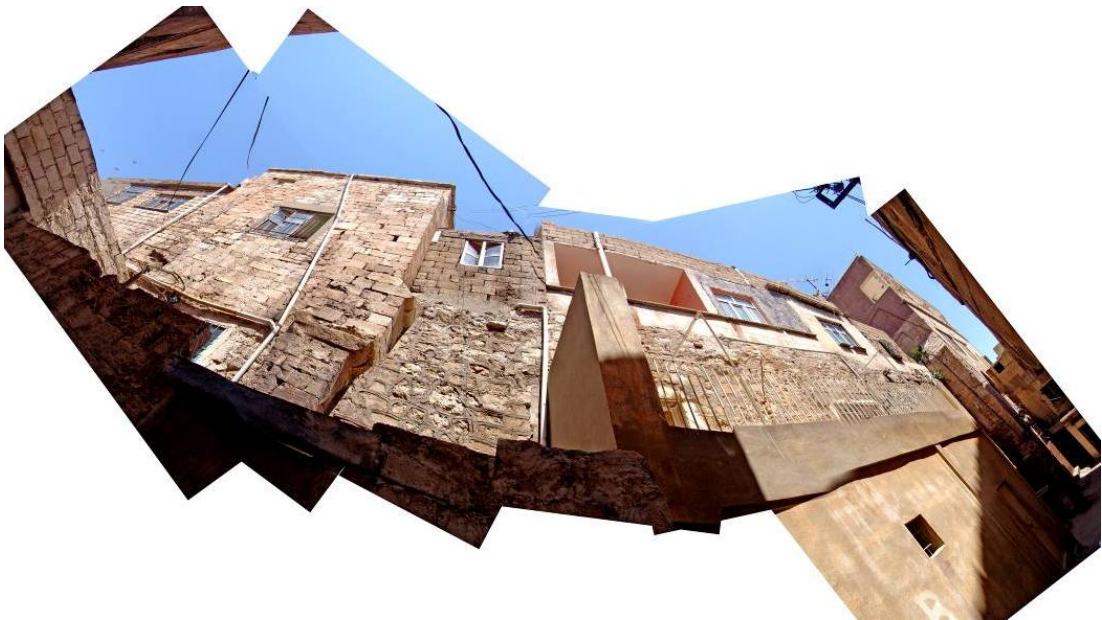
Figure 2.85 : The southern face of the Block-II – looking north at the junction between IIL1-4 group and the portal mass.
