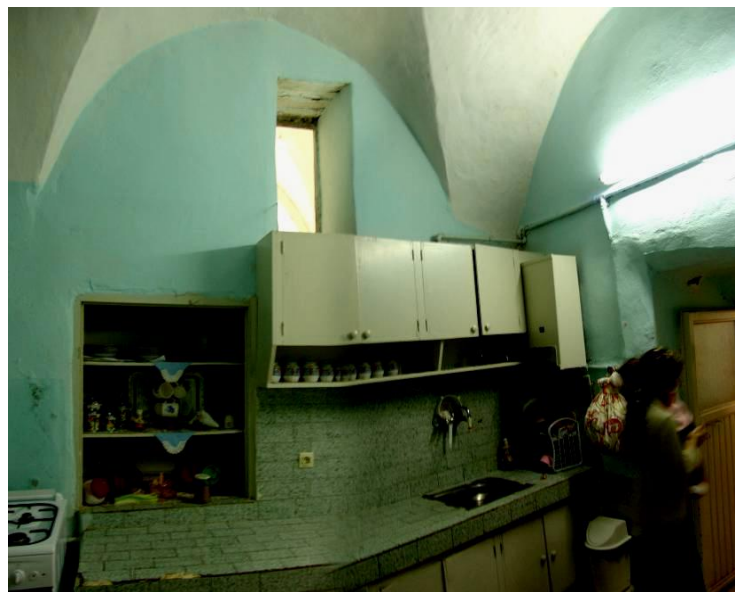
Figure 2.281 : The southern wall of the VM10 volume.
