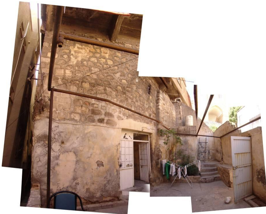
Figure 2.58 : The exterior of IL7 – looking northeast from the ILt terrace.
