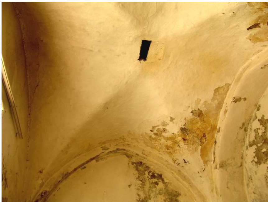
Figure 2.97 : The vault of the IIL6 volume.
