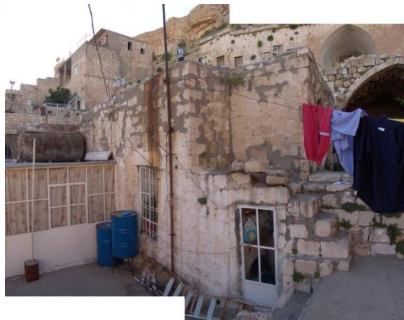
Figure 2.258 : The southwestern exterior corner of VM5 – view from VMt1.
