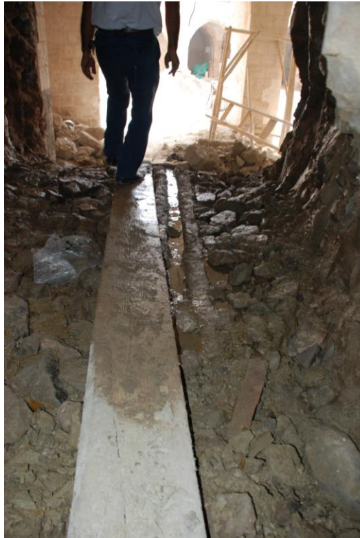
Figure G.5 : The water channel on the base of tunnel – the first leg of the tunnel looking south.
