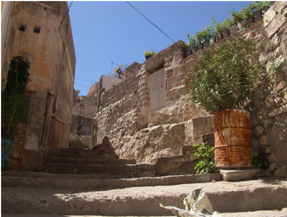
Figure 2.65 : View from the internal street – looking west from the collapsed IIL2 volume.
