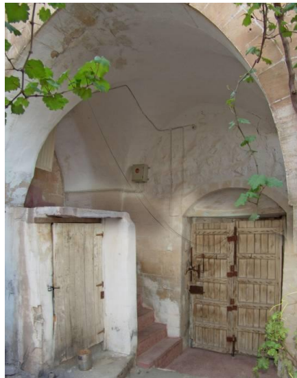
Figure 2.236 : The entrance to the Block-VI residential unit and the staircase going up to the terrace – looking east from within the curtyard.
