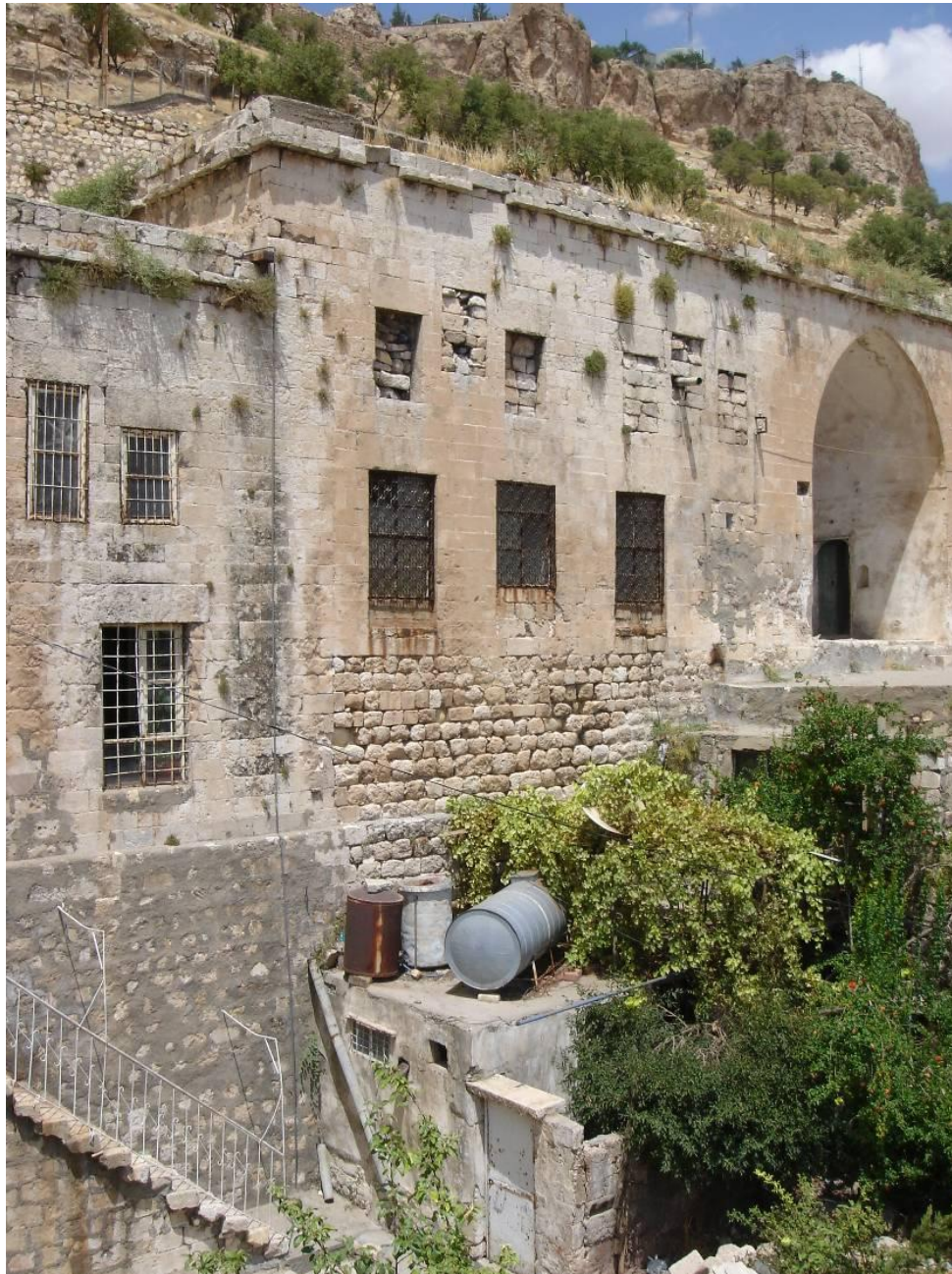
Figure 2.211 : The southern face of the upper layer and the junction detail of its eastern and western wings.
