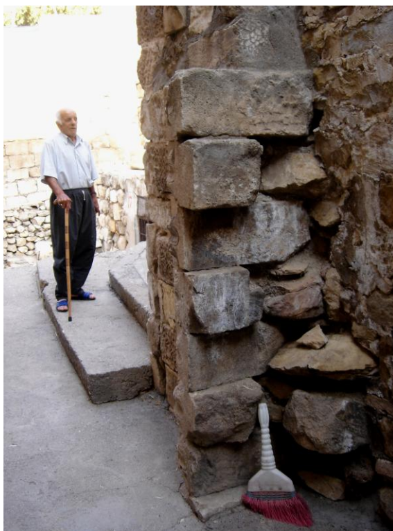
Figure 2.365 : The back of the stone lay holding the Altunboğa Portal remains – looking west.
