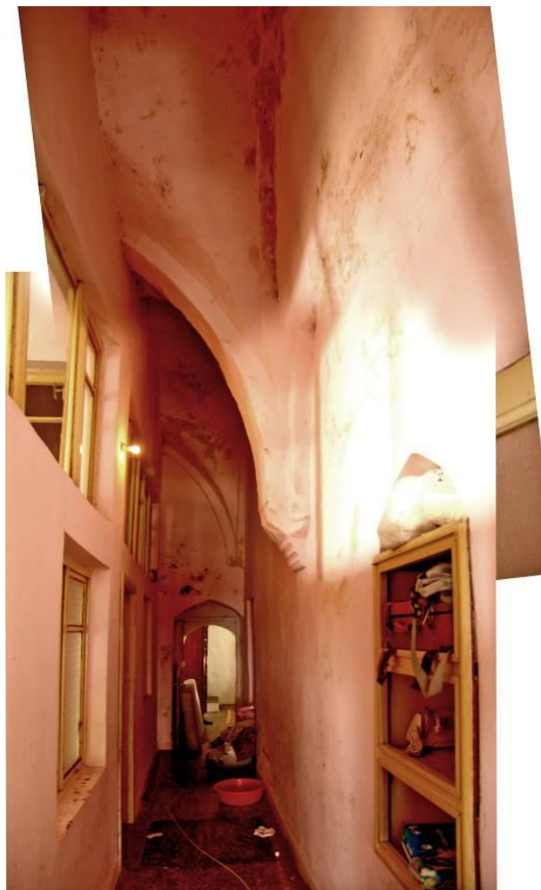
Figure 2.173 : The arch-vault-impost system of the IIIM5-7 volumes – looking north from recent corridor formed.
