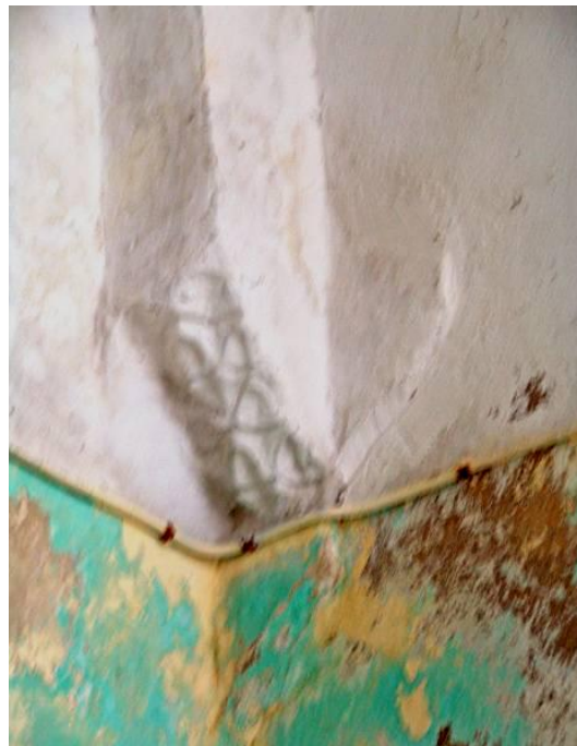
Figure 2.213 : Detail of the muqarnases defining the corner junction of the groin vault frames of the IVU8 volume.
