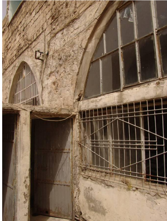
Figure 2.112 : The arches of IIL8 and IIL12 opening to the Pınarcık Street.
