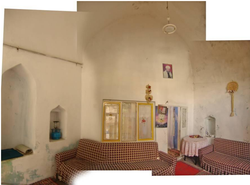
Figure 2.193 : The IIL5 volume – looking west.
