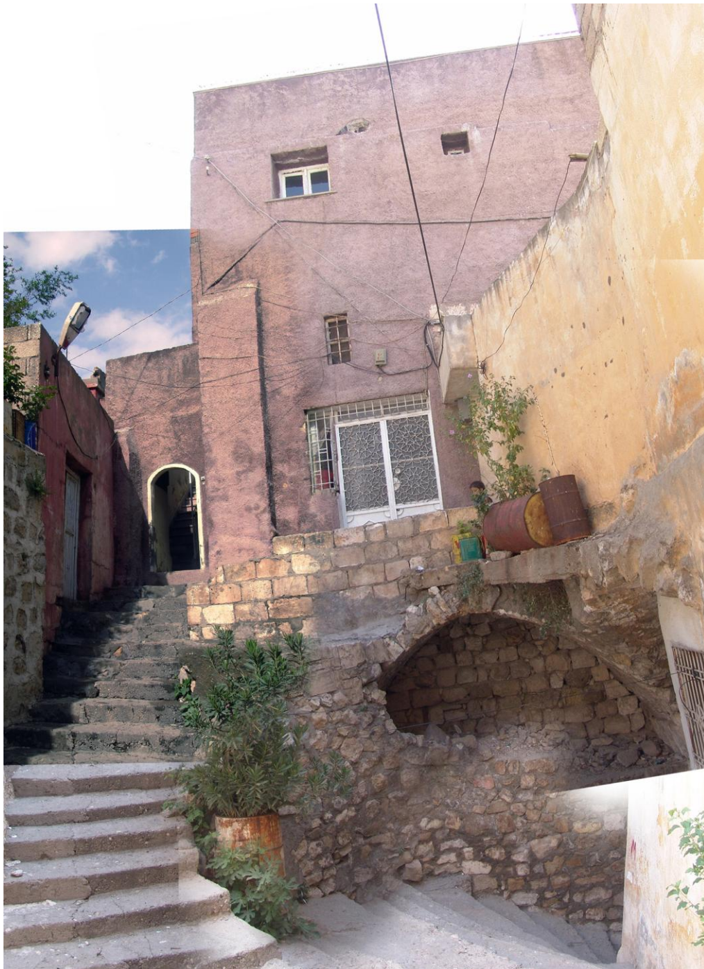
Figure 2.293 : The western face of Block-I and the northern buttresses holding the IL1-2 volumes.
