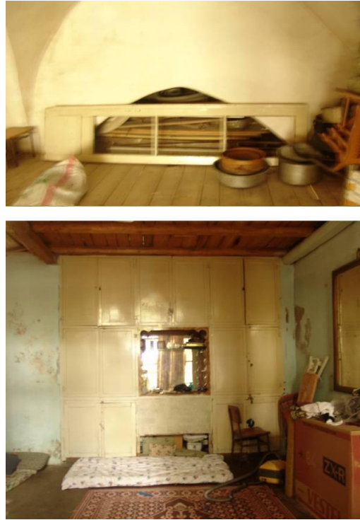
Figure 2.253 : The western wall of VM3.
