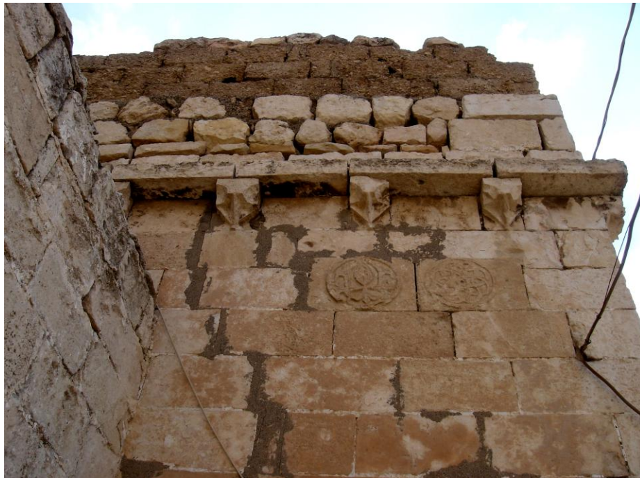
Figure 2.387 : The stone mason's seals on the eastern wall of the IIIM7 volume in its context.
