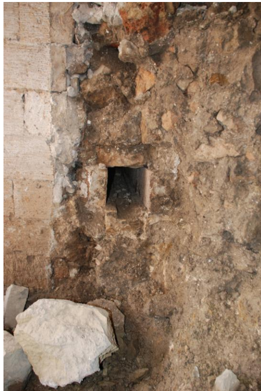
Figure G.6 : The water channel running about a meter high right behind the retaining wall – looking west from the discovered entrance.
