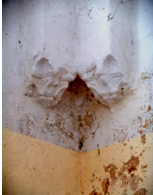
Figure 2.212 : Detail of the muqarnases defining the corner junction of the groin vault frames of the IVU10 volume.
