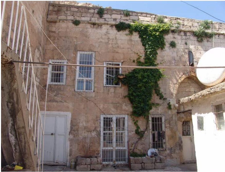
Figure 2.216 : The northern face of the IVU10 and IVU6 volumes.
