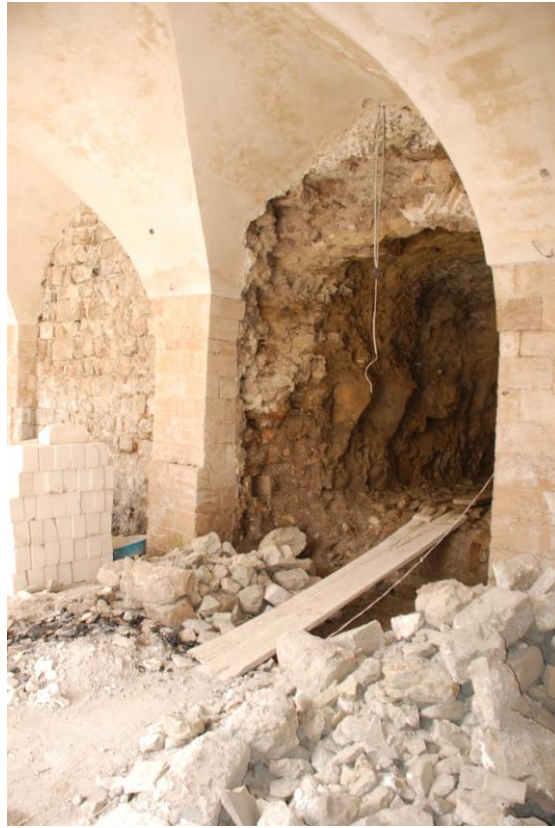
Figure G.3 : The discovered entrance to the northern tunnel – the eastern end of the tunnel aligning with the han's retaining wall.
