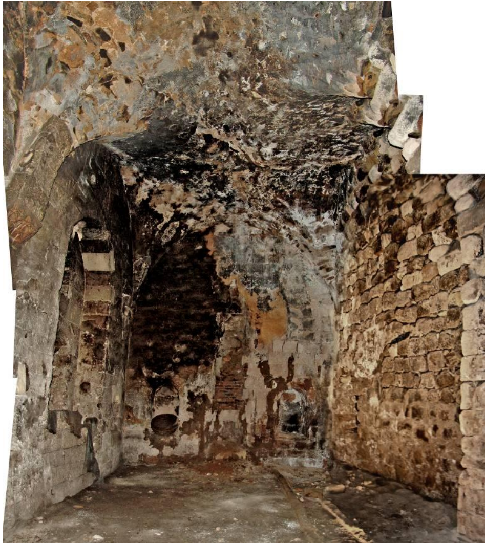
Figure 2.329 : The eastern wall of the IL5/zaviye volume.
