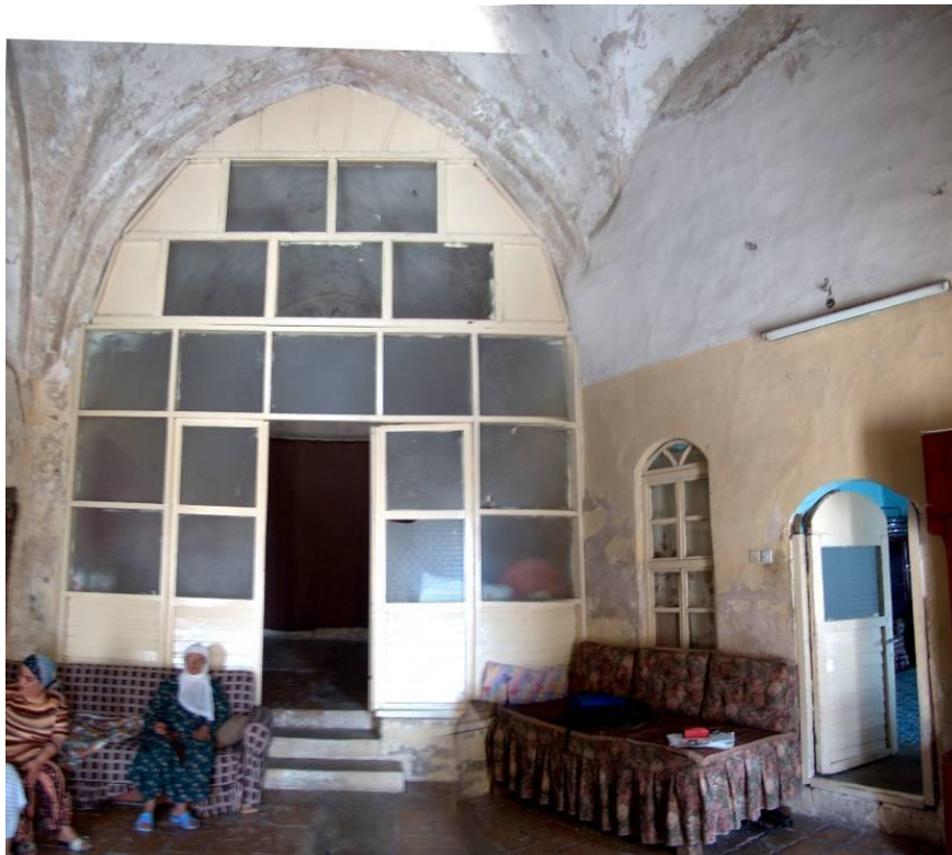
Figure 2.221 : The northern division wall and level difference between the IVU6 and IVU7 volumes – looking north.
