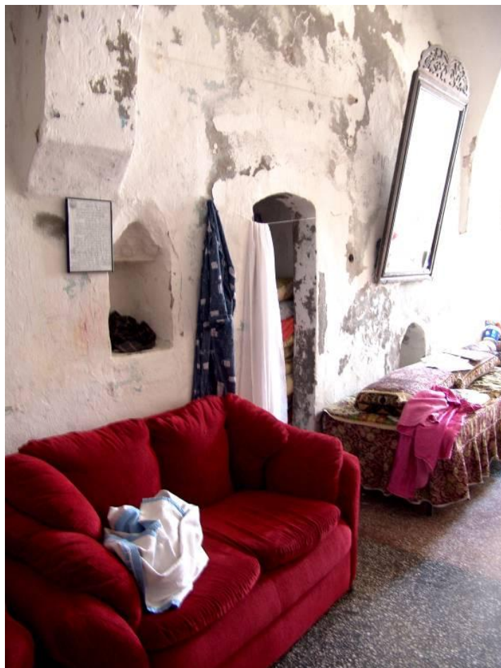
Figure 2.160 : The muqrnas niche between IIIM2 and IIIM3; and the closed doorway to IIIM14 from IIIM2.
