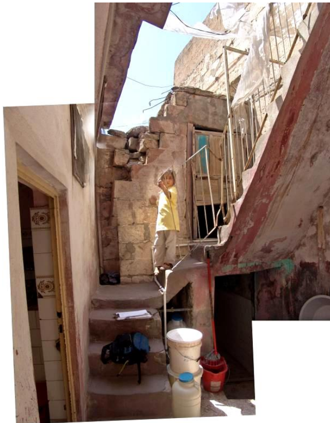
Figure 2.68 : The zone between Block-II and Block-III with the staircase rising to the Block-II terrace – looking south from the middle layer courtyard level.
