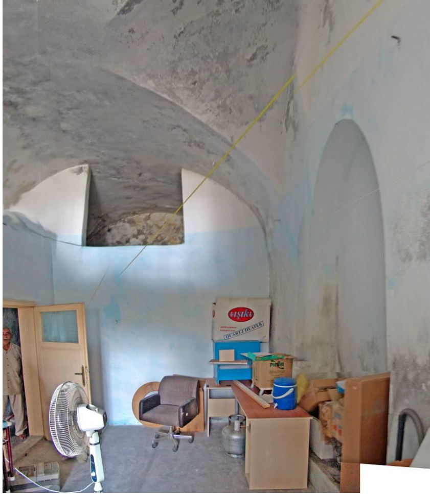
Figure 2.169 : The northern LB concrete-block internal division wall of the IIIM4 volume.
