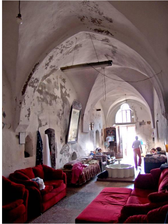
Figure 2.153 : The IIM1-4 volume – looking east from IIM3.
