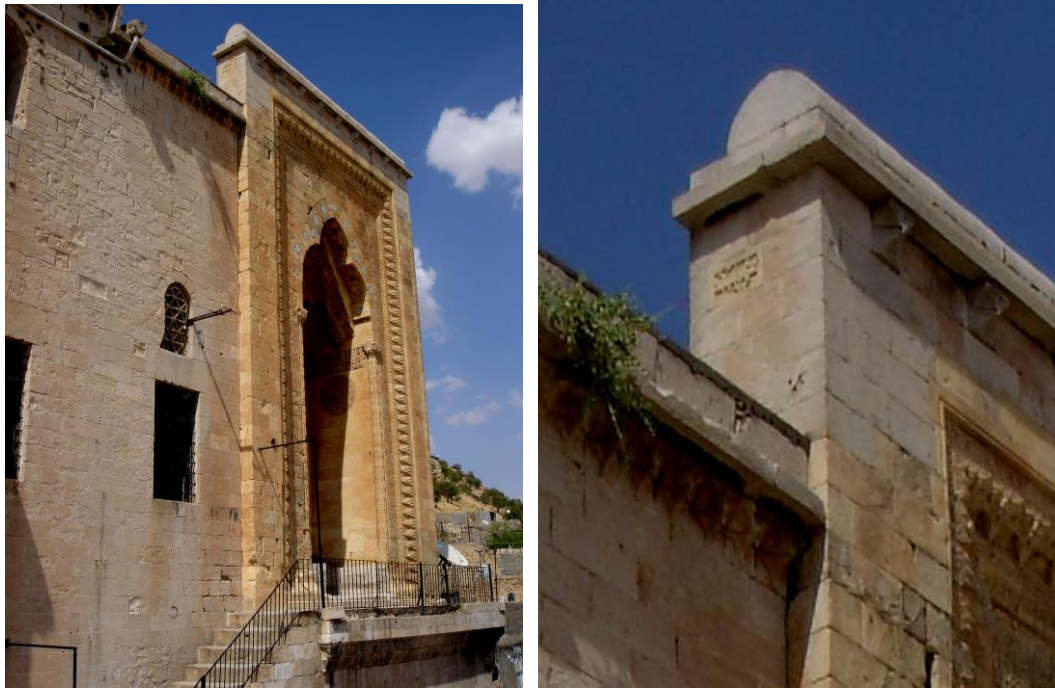
Figure 2.388 : The stone mason's seals on the eastern wall of the Zincirye Medrese's portal.
