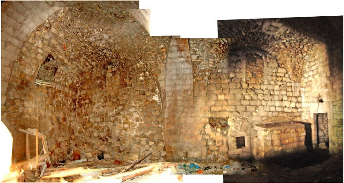
Figure 2.134 : The western walls of the IIM14 volume.
