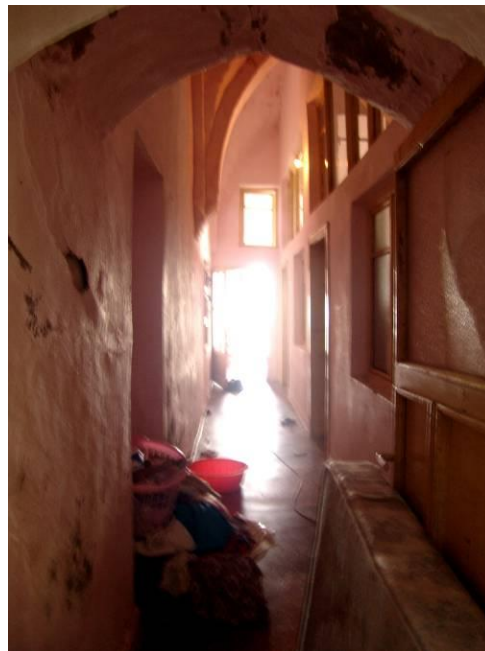
Figure 2.181 : The corridor formed by "the internal subdivision wall within the IIM5-7 system; and the enclosed doorway between IIM5 and IIM10.
