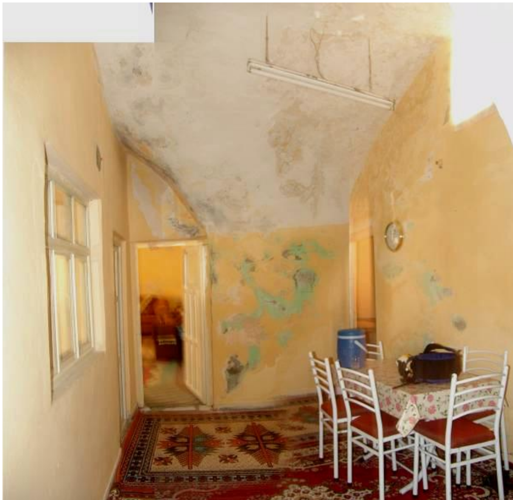
Figure 2.88 : The IIL3 volume – looking west.
