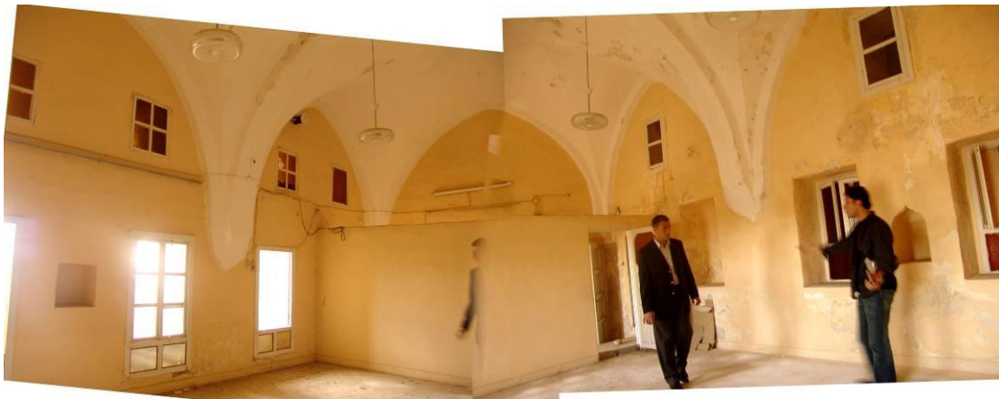
Figure 2.347 : The IM10 volume – looking west.
