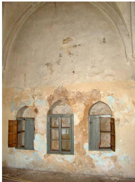
Figure 2.201 : The northeastern wall of the IVU4 volume.
