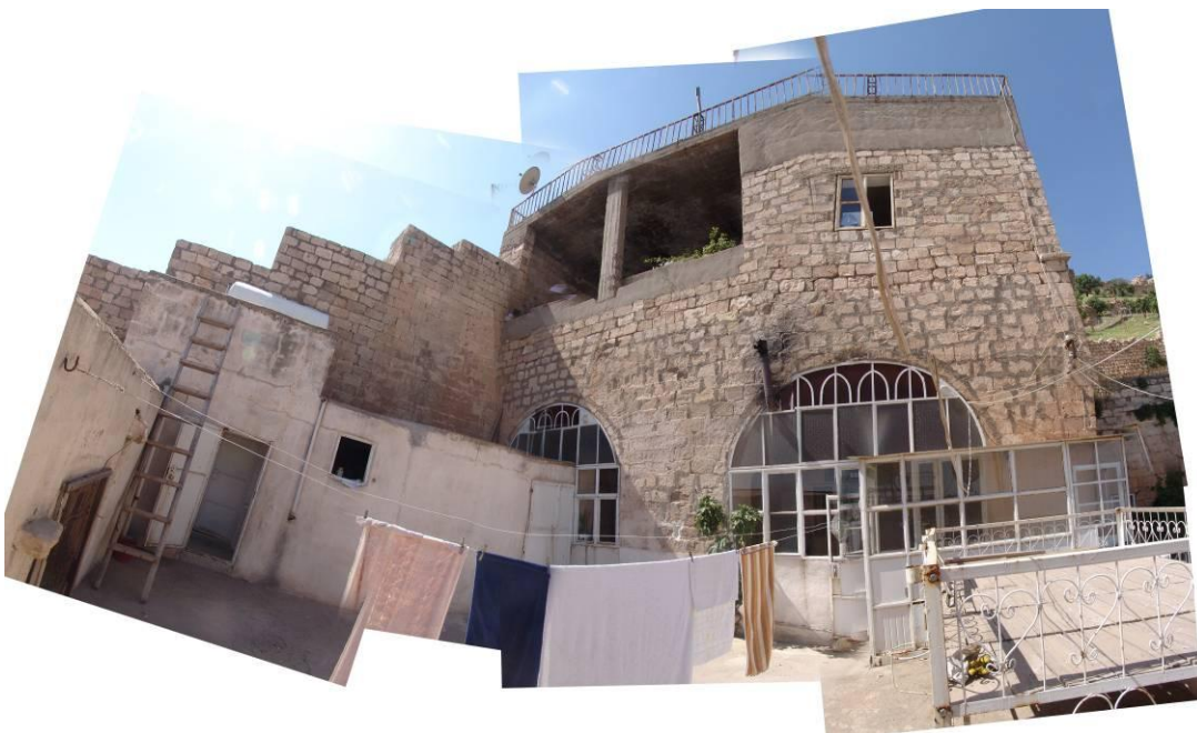
Figure 2.227 : The courtyard between the IVU13 and IVU14 volumes.
