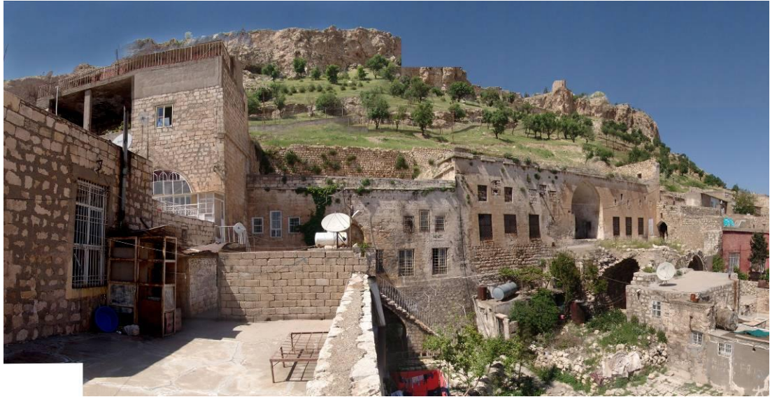
Figure 2.75 : The main courtyard, the collapsed VM3 aiwan and the upper layer, and the Block-III terraces – looking north from the IIIUt terrace.
