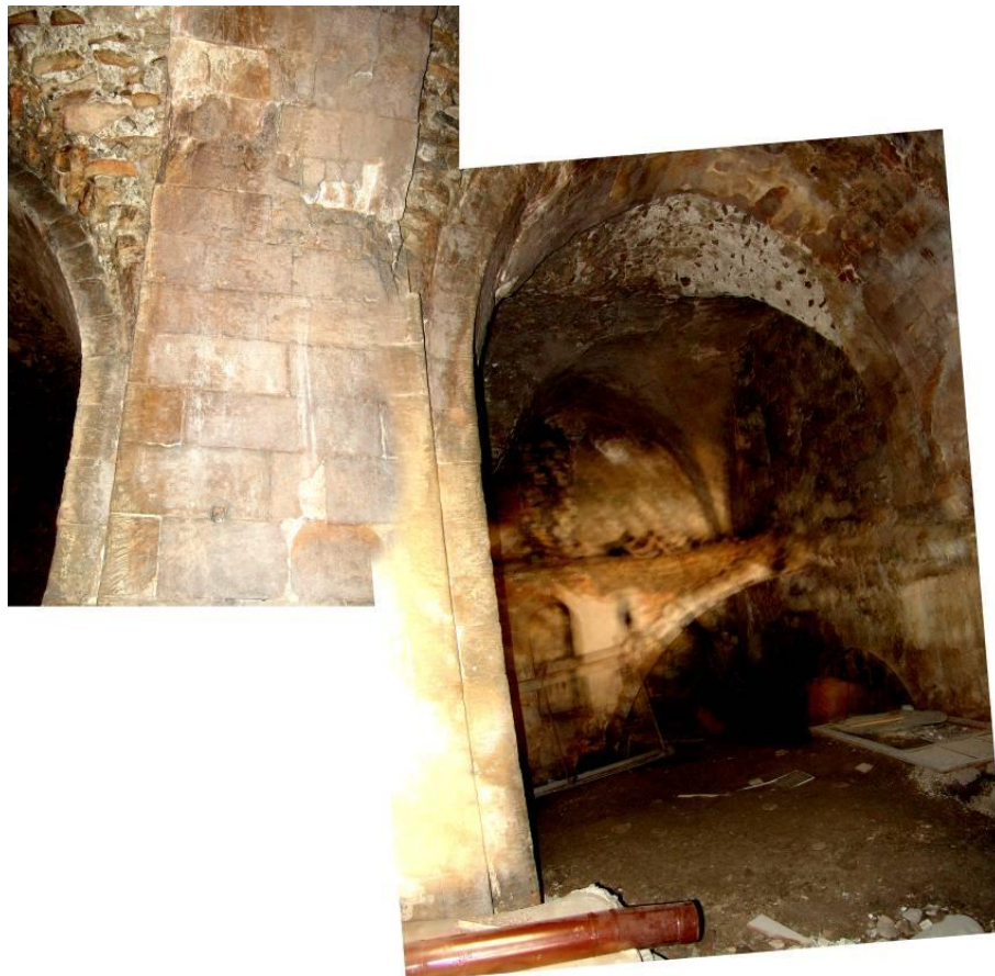
Figure 2.131 : The central column holding the four vaults of IIIM14 – looking to the northeastern corner.
