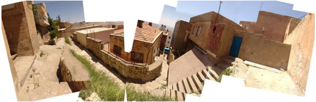
Figure 2.44 : Panoramic view of the eastern entrances to the settlement – from the entrance to the eastern independent house (left) to the southeastern entrance to the settlement (right).
