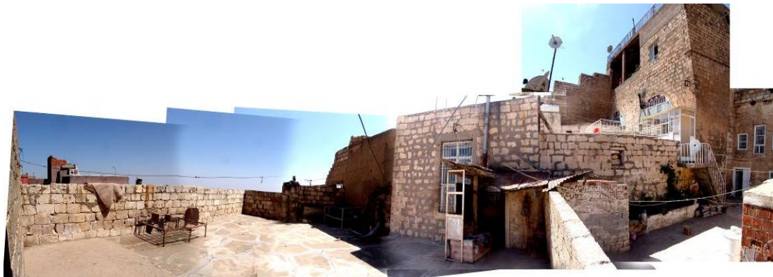
Figure 2.225 : Panoramic view of the western wall rising between the IIIUtW and IIIUtw3 terraces.
