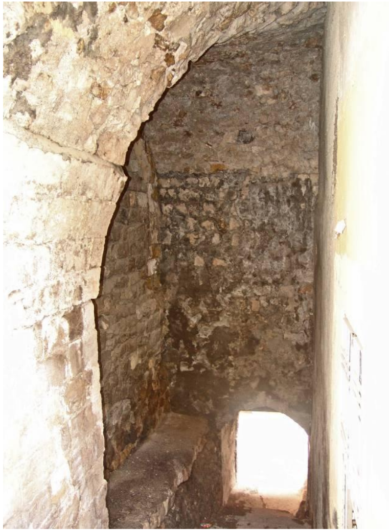
Figure 2.47 : The entrance volume to the settlement – looking north from the ruined passageway.
