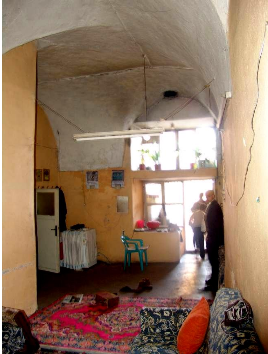
Figure 2.286 : The southern wall and entrance of the VM L 1-2 volumes.
