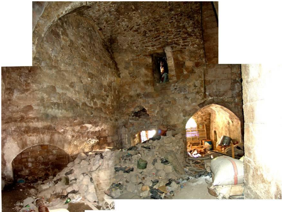
Figure 2.135 : The northeastern wall, cooking hearths of the IIM14 volume; and the arches leading to IIM13.
