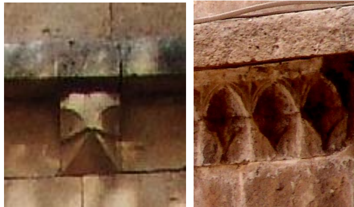
Figure 2.394 : Detail showing the the corbel geometry on the Firdevs Köşk and the Sultan Hamza Mousoleum – the Sultan Hamza Mousoleum (right).
