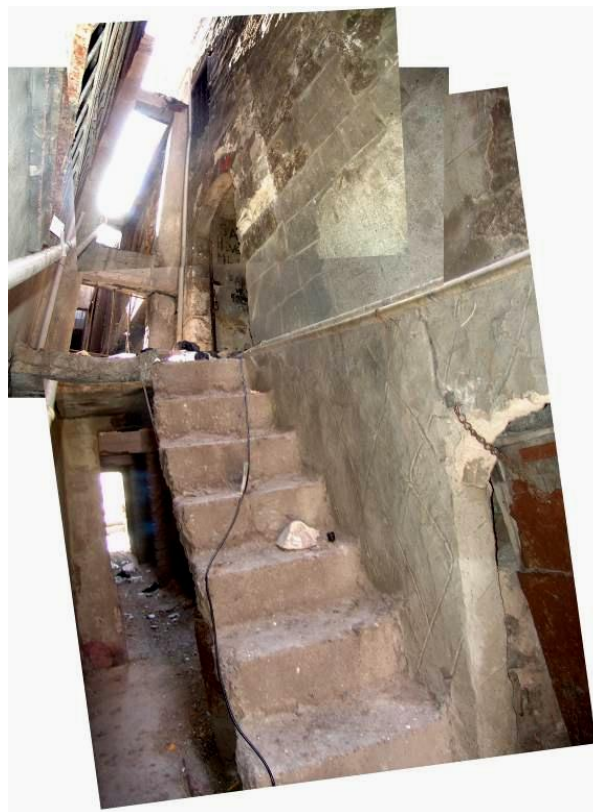
Figure 2.313 : The staircase on Pınarcık Alley leading up to the entrance doorway of the IL4 volume – looking west.
