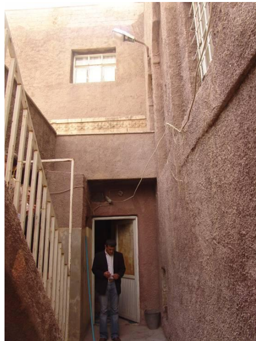
Figure 2.344 : The eastern end of the internal street: the western passageway opening to Block-I and the entrance to the IM7 – looking west.
