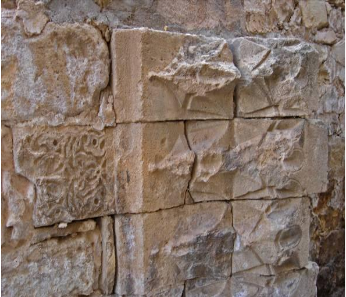
Figure 2.27 : The remains of the Altunboğa Medrese Portal.
