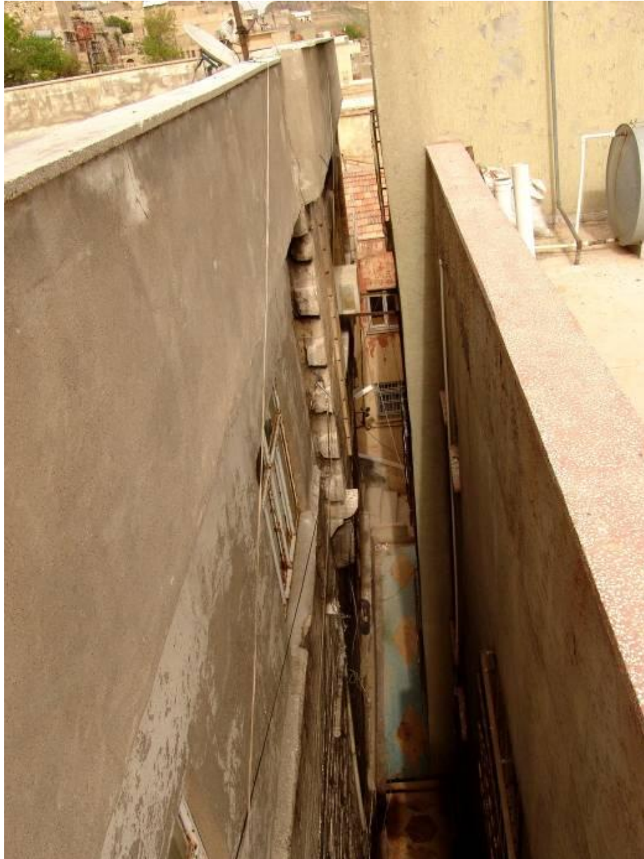
Figure 2.346 : The Pınarcık Alley seen from the top – looking west.
