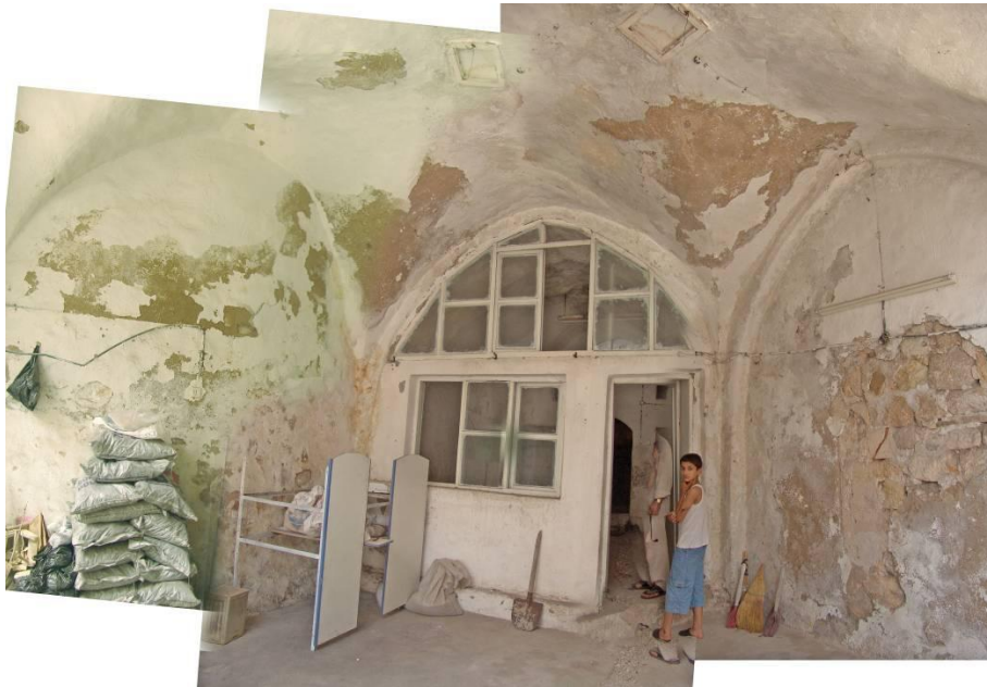
Figure 2.114 : The IIL8 volume opening to IIL9 – looking north.
