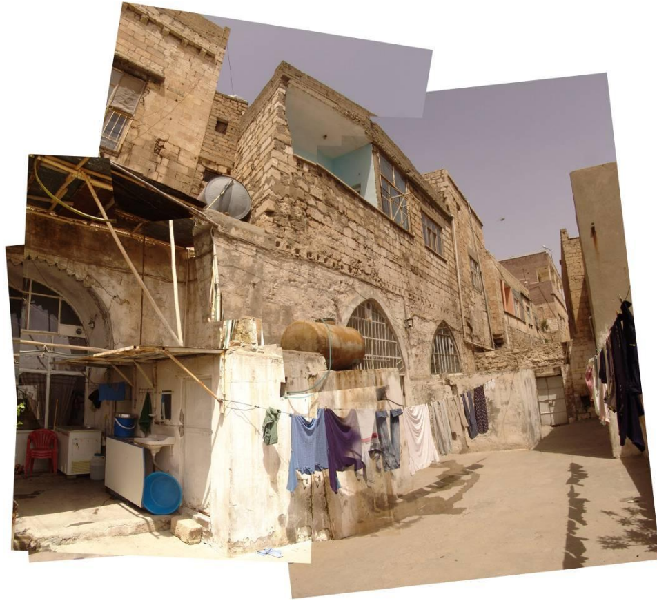
Figure 2.13 : The middle part of the southern façade.
