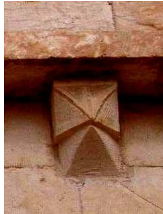
Figure 2.392 : Detail showing the the corbel geometry on the Zinciriye and Kasimiye Medreses and the Büyük Han – from the Kasimiye Medrese.
