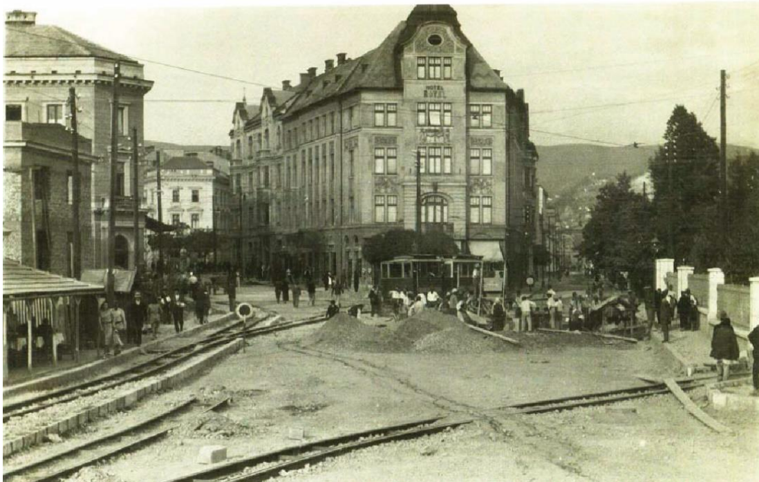
Figure 3.12 : Establishment of the tram tracks at Aleksandrova Street in Marijin Dvor (URL-12).
