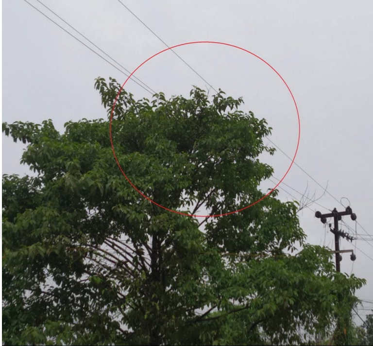
Figure 2.1 : HIF due to the contact of tree limb with a primary conductor [16]
