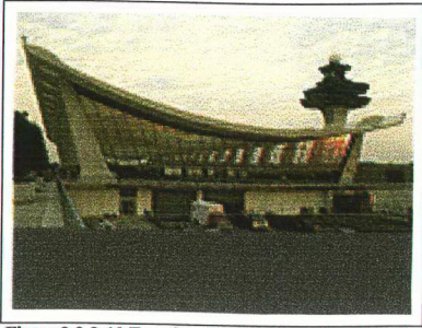
Figure 3.2.3-10 Eero Saarinen: Dulles International Airport, Terminal Building, 1958-1962, Chantilly. Exterior at night.
