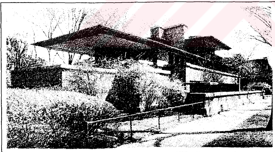
Figure 3.1-3 Frank Lloyd Wright: Frederick C. Robie House, Chicago, Illinois, 1906-1909. Street view.
