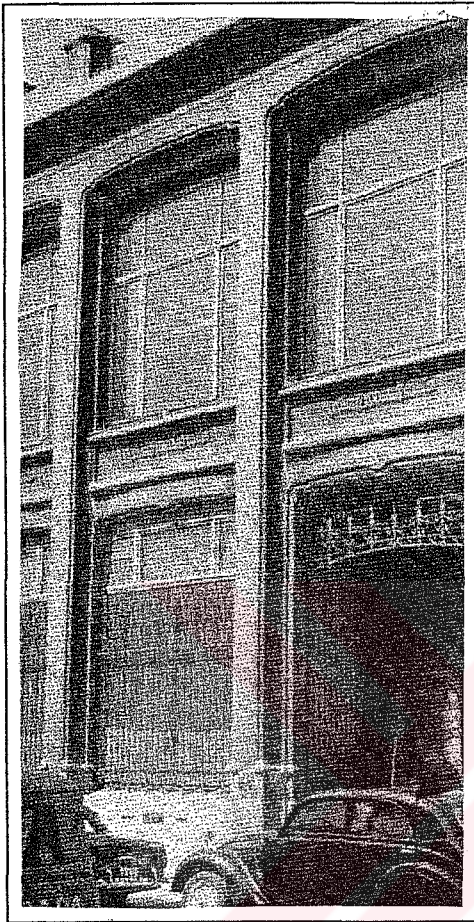
Figure 2.2-5 Victor Horta: Gross Waucquez Building, Brussels, 1903-05. Façade detail.
