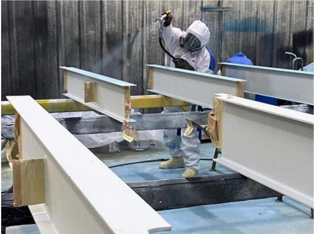
Figure F.1 : Surface protection coatings to the steel structure.
