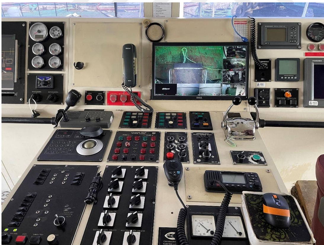
Figure H.4 : Control panel of SH-SUTLUCE.
