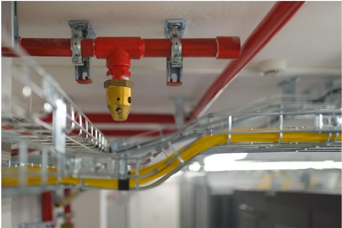
Figure B.1 : Fire extinguishing systems.
