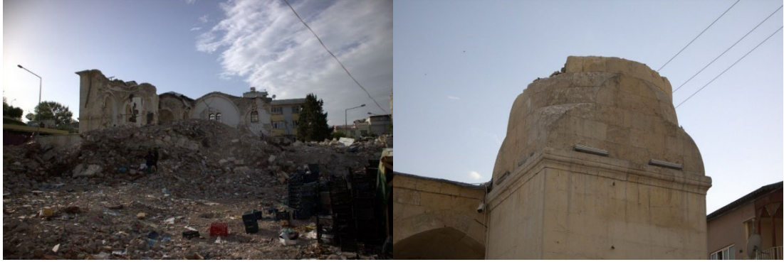
Figure 2.4 : (a) The most important mosque in Adiyaman, Adiyaman Grand Mosque, after the earthquake. (b) Base of the minaret, minaret is missing (Cilesizoglu, 2023).
