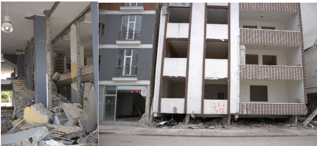
Figure 2.6 : (a) A case of two-story height floor. (b) A case of soft story, the ground floor completely collapsed (Cilesizoglu, 2023).
