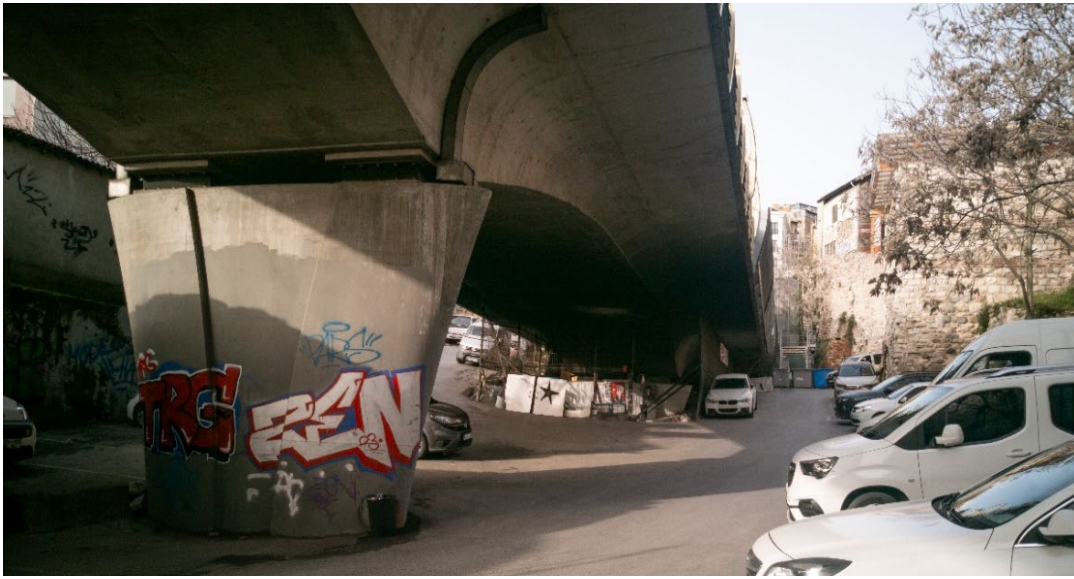
Figure 5.1 : Project area, underside of Haliç Metro Bridge intersecting with historical walls and urban fabric of Azapkapı (Cilesizoglu, 2023).
