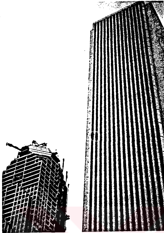
Photo 13, Amoco Standard Oil Building Chicago, 1990 Photo by Murat Mayor
