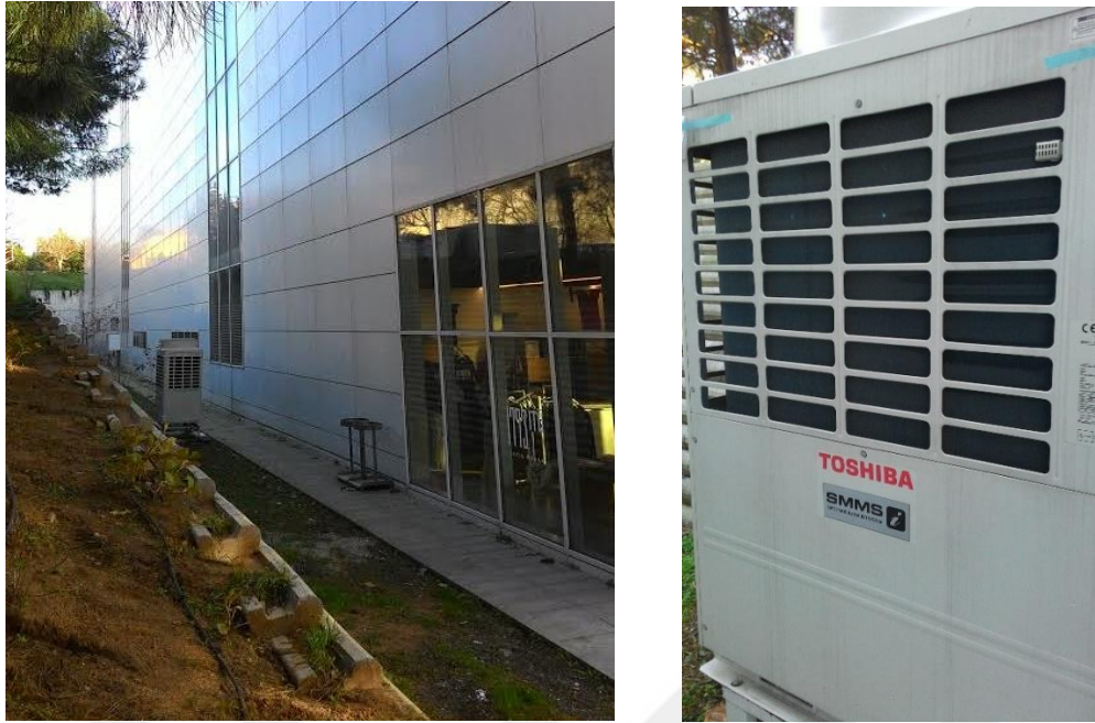
Figure 5.8 : VRF outdoor units in MED garden.
