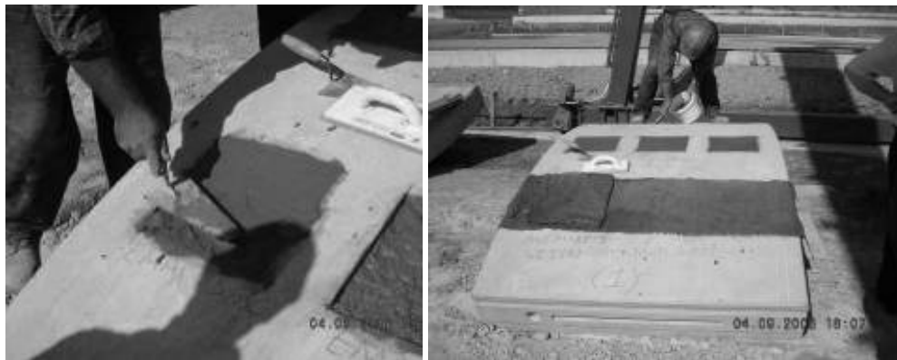
Figure 5.6 : Application and Curing of the Repair
