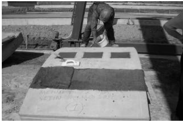
Figure 3.3 : Curing of the Repair
