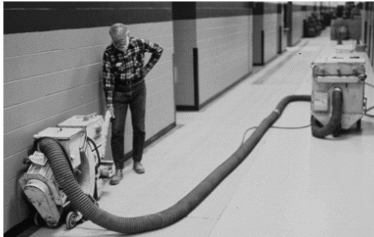
Figure 3.2 : Shot blasting Equipment to Remove Shallow Concrete Deterioration [4]
