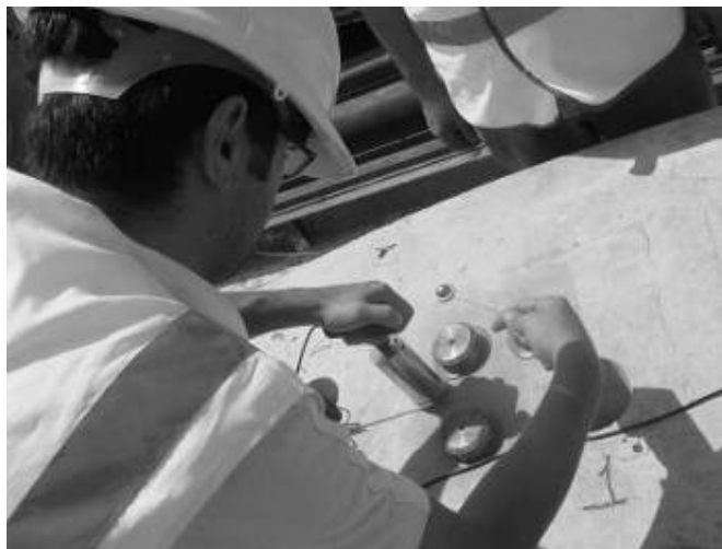
Figure 5.10 : Impact-Echo Testing on the Construction Site
