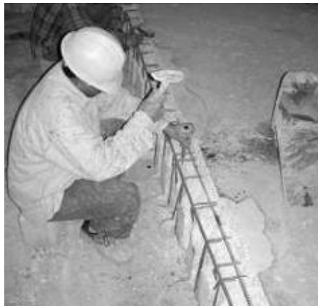
Figure 3.1 : Impact Removal Technique
