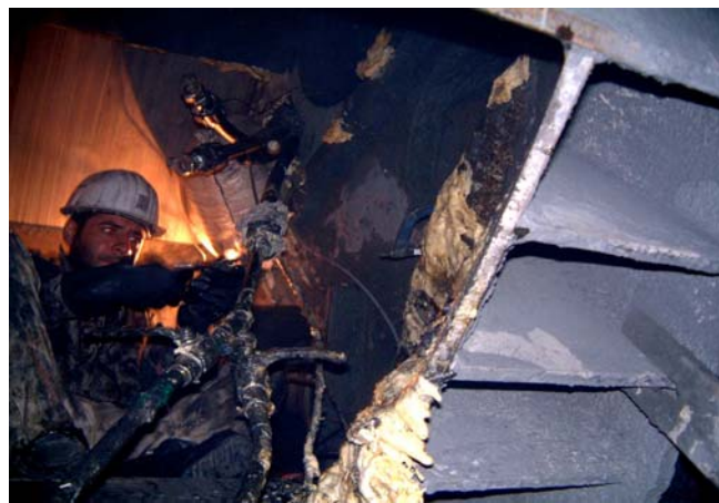
Figure 6.14 : PU and PUR post grouting injection in Mavi (Blue) Tunnel.
