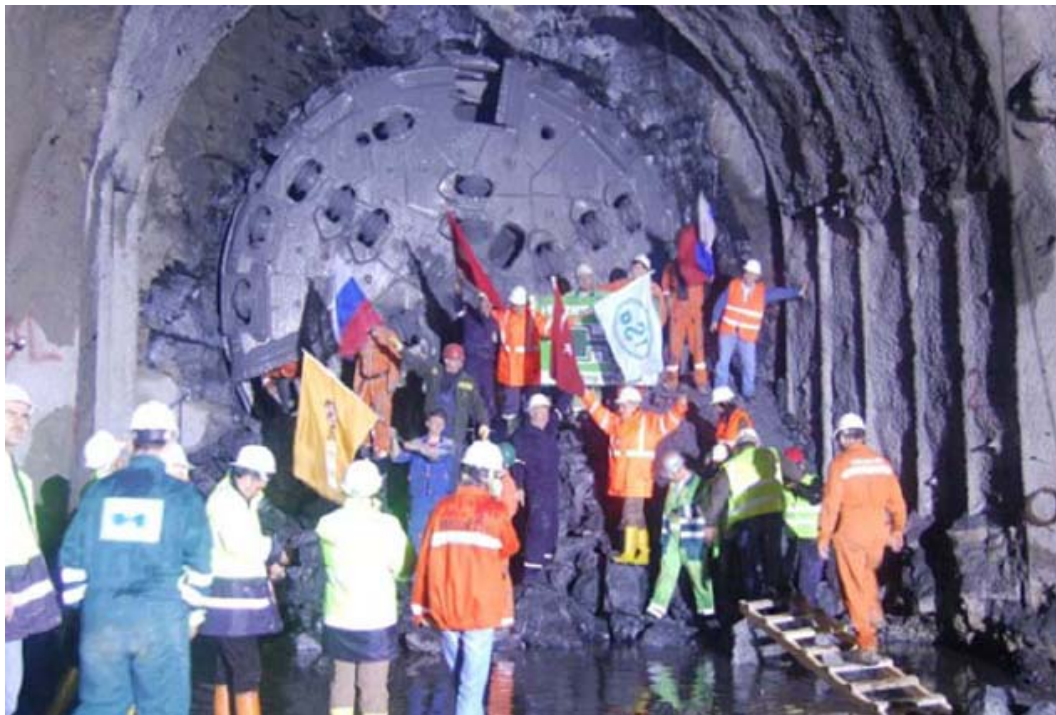
Figure 6.28 : Breakthrough Ceremony of Melen (Bosphorus Crossing) Tunnel.
