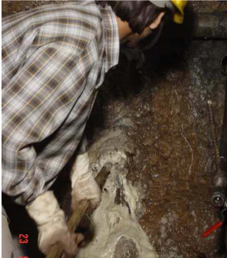
Figure 6.15 : PU injected as post grouting behind the segments in Mavi (Blue) Tunnel- Expansion reaction is ongoing.
