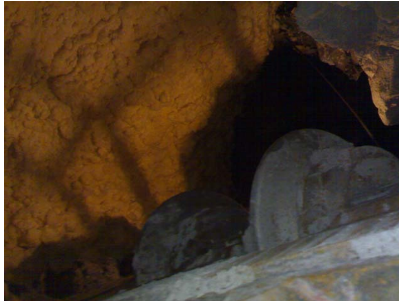
Figure 6.17 : Foamed PU in front of the cutterhead.
