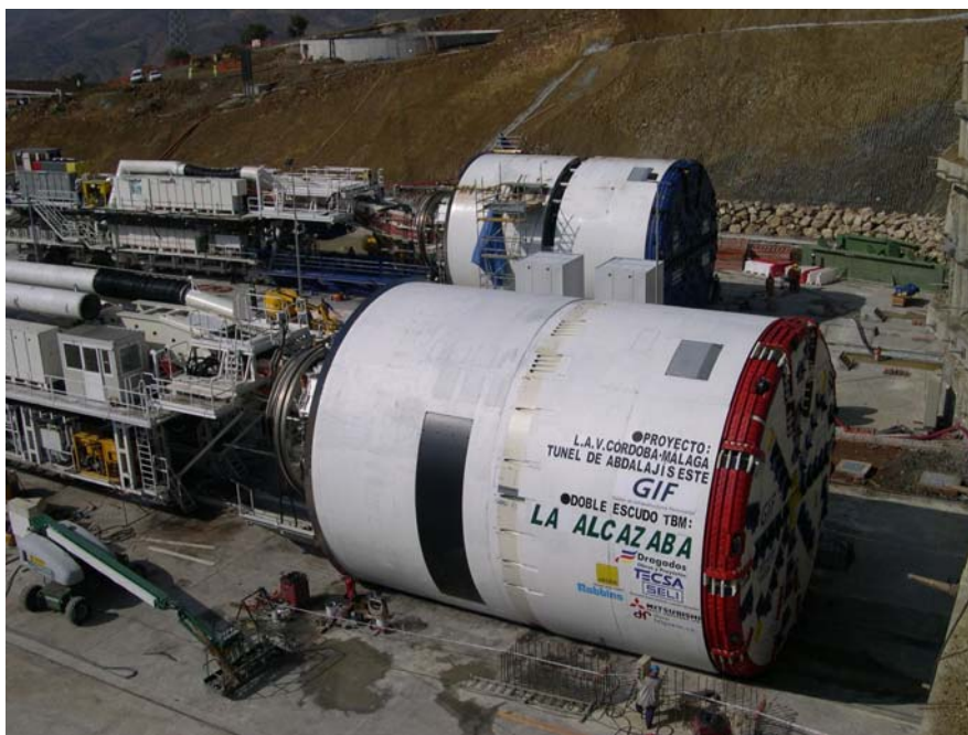
Figure 5.10 : The abdalajis project-Double shield TBM.
