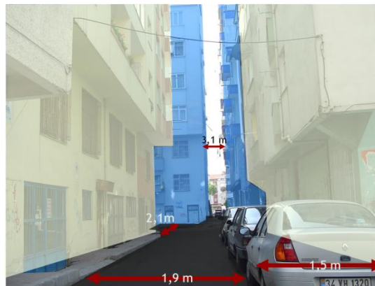
Figure 4.4: A Street scene showing narrowness in Çırpıcı – Zeytinburnu.
