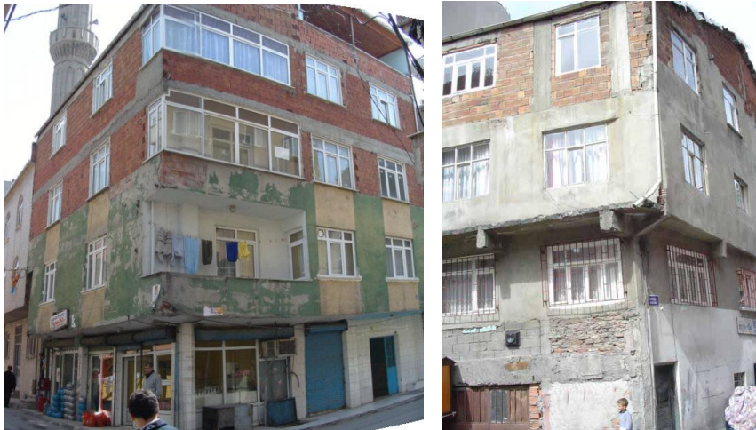
Figure 5.2: Zeytinburnu - Poor quality concrete building stock.
