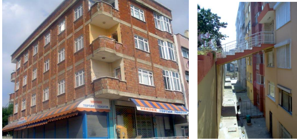
Figure 5.23: Southern Avcılar - Concrete buildings having entrance from upper floors only.
