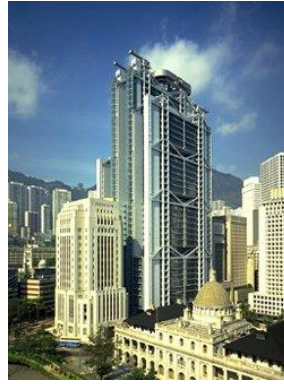
Şekil 4.40 Hong Kong and Shanghai Bank, Norman Foster
