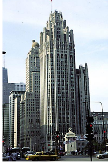
Şekil 4.17 Chicago Tribune Building Raymond Hood & John Mead Howells.
