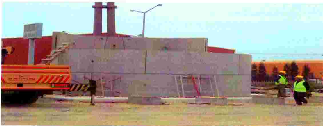
Figure 9.9 : Checking of Ring geometry at the site.
