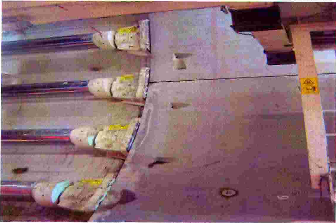
Figure 9.1: Jacks of TBM.
