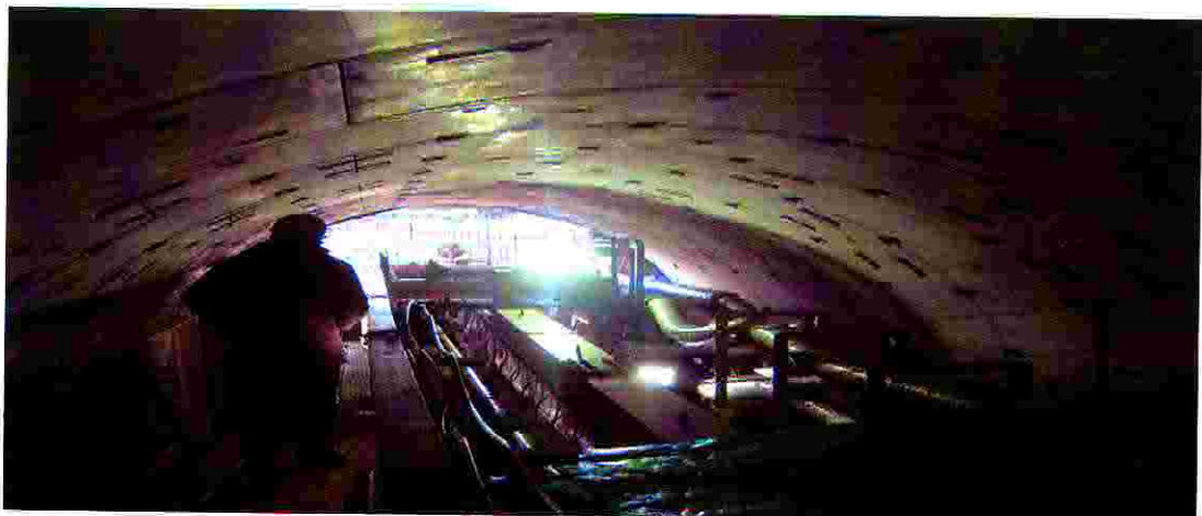
Figure 9.5: After assembling the segments
