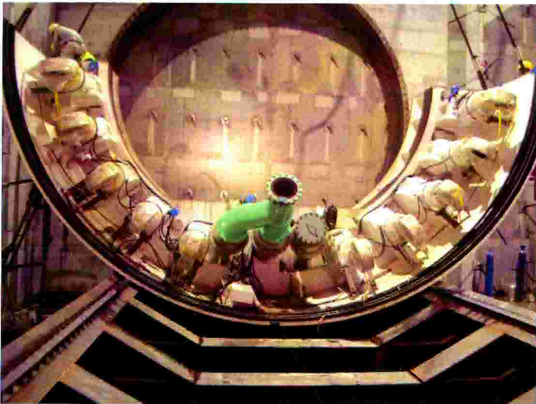
Figure 11.4: Fixing of TBM Saddle
