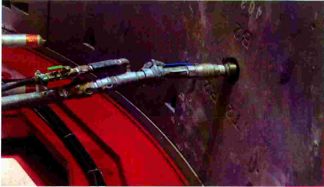
Figure 9.2: Backfill process.
