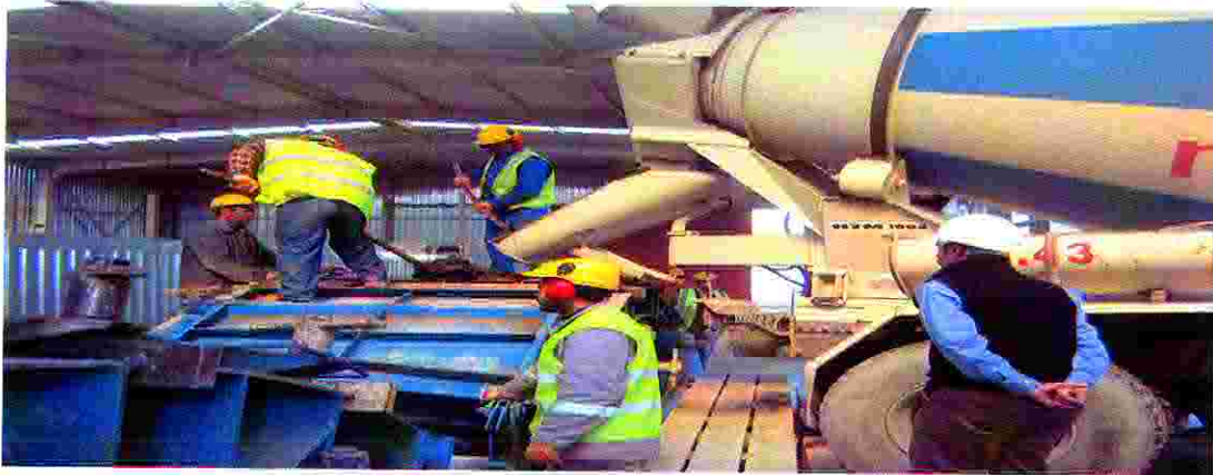
Figure 9.12: Casting of R/C Segment Concrete for TBM.
