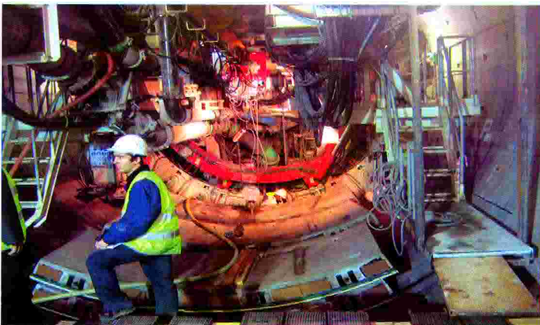
Figure 9.3: Erector operation
