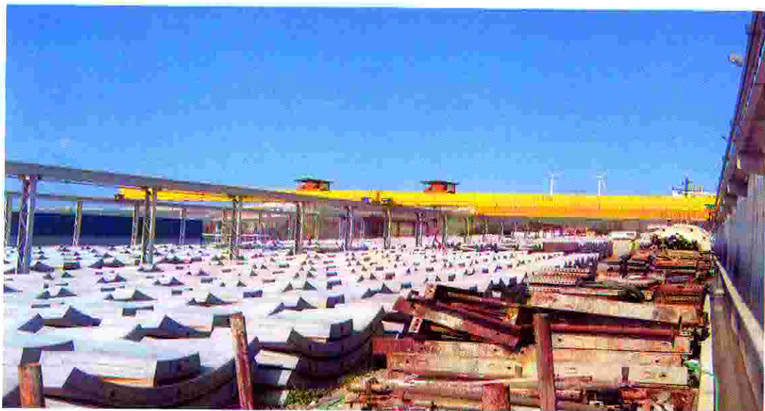
Figure 9.14: Storage of segments prepared for TBM
