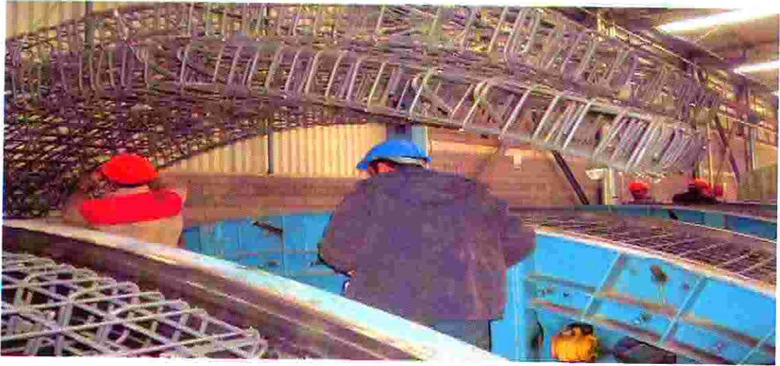
Figure 9.7: Preparation of R/C Segment reinforcement
