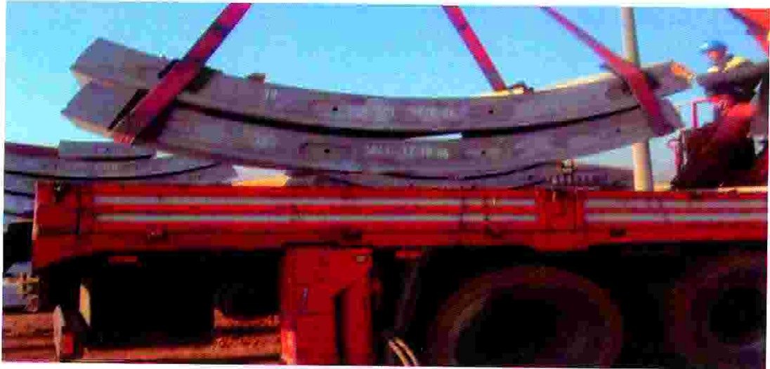
Figure 9.4: Transportation of the segments
