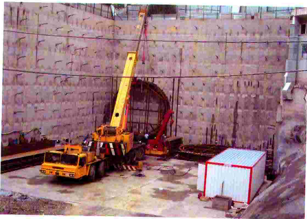
Figure 11.1 Setting of Entrance Hardware
