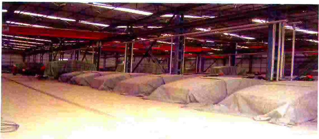
Figure 9.13: Curing period of R/C Segment Concrete for TBM.
