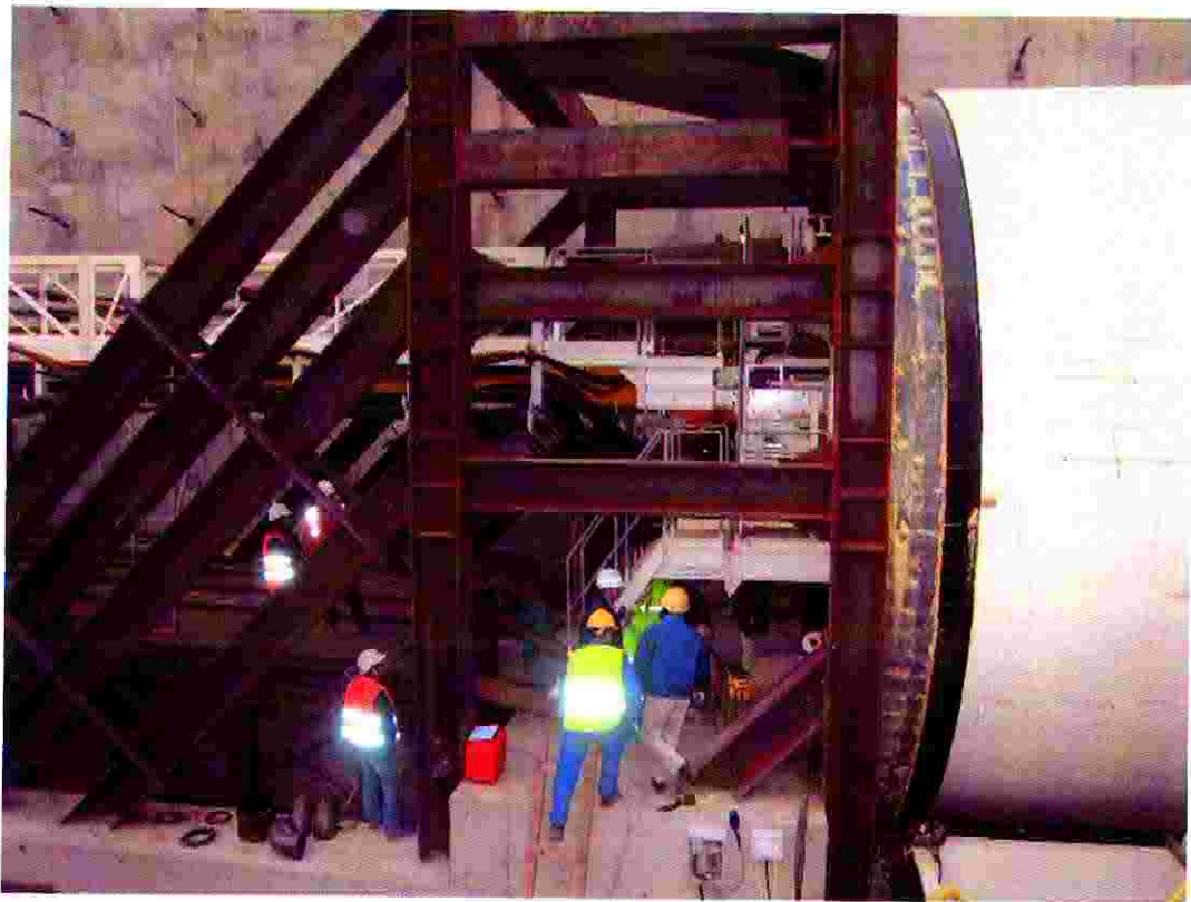
Figure 11.5: Setting of reaction beam
