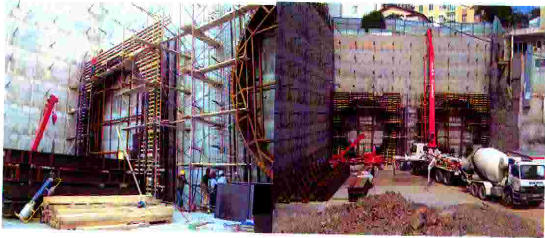
Figure 11.2: Formwork and Casting Concrete
