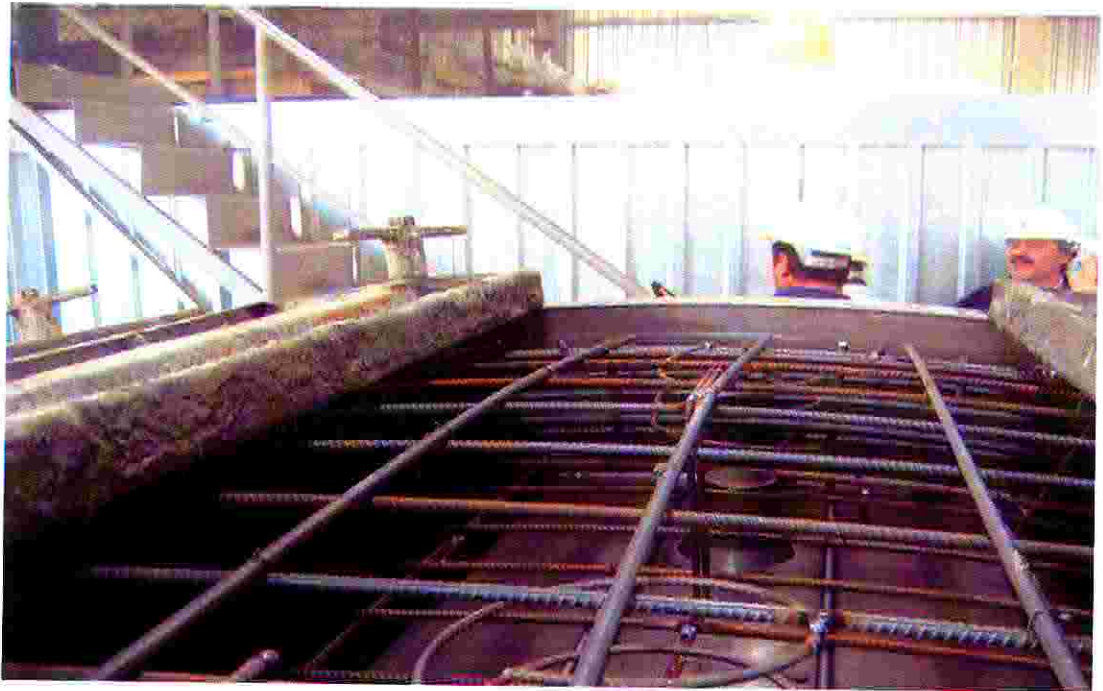
Figure 9.8 : After preparation of R/C Segment reinforcement.
