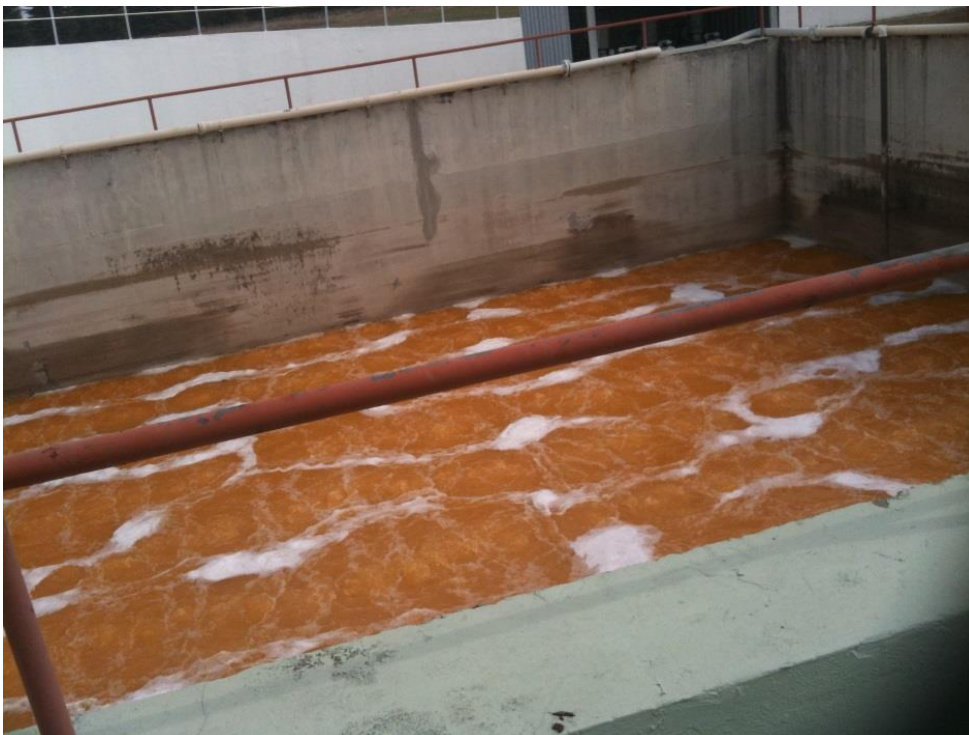
Figure 3.12. Neutralization Pool.
