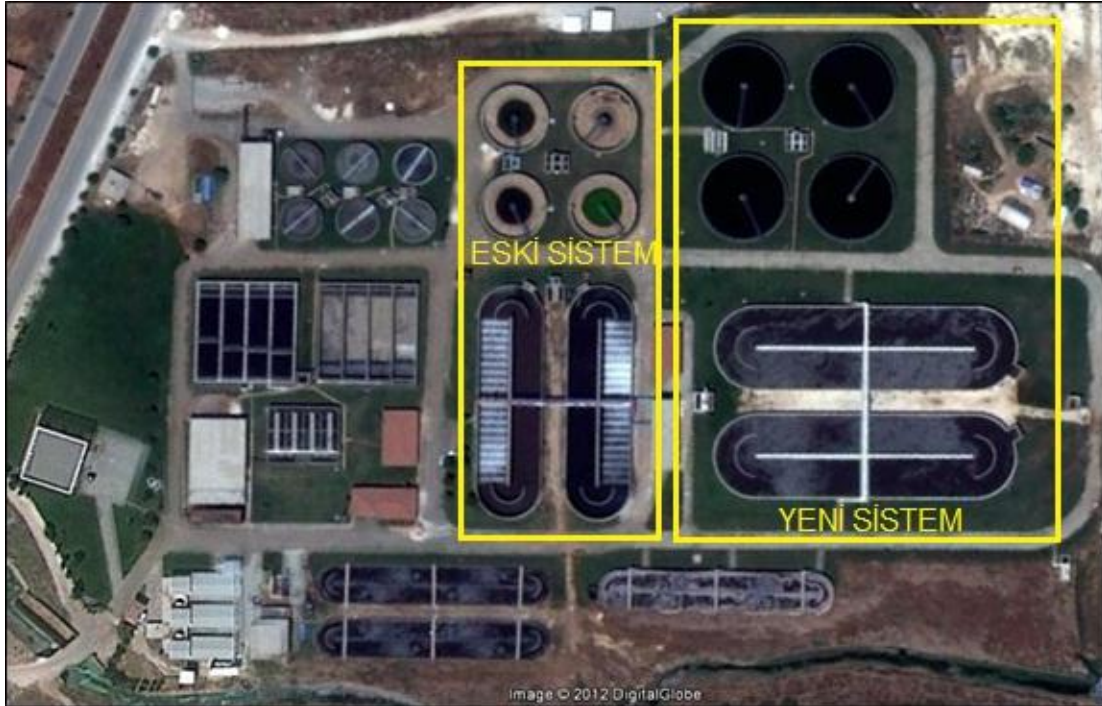
Figure 3.1 : Satellite Image of GaOID Wastewater Treatment Plant
