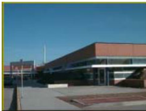
Figure 4.4: High sidelighting clerestory exterior lightshelves in elementary school [33].
