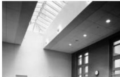
Figure 4.11: Patterned linear top lighting
