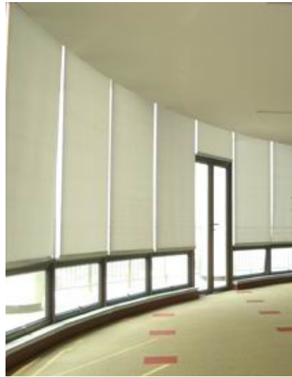
Figure 3.23: Internal roller blinds [54].
