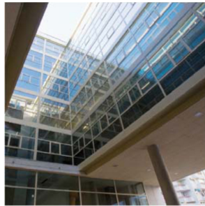
Figure 5.8: View from the interior patio [69].
