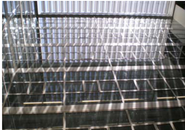
Figure 4.12: Lamellas over central patio seen from below [70].
