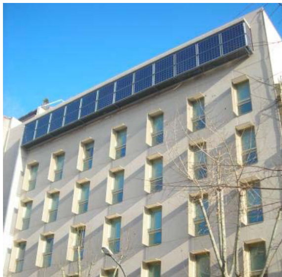
Figure 4.15: Front façade view with fixed shading [69].
