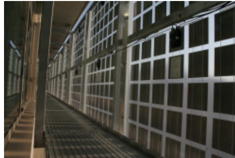
Figure 4.17: PV installation on façade [70].
