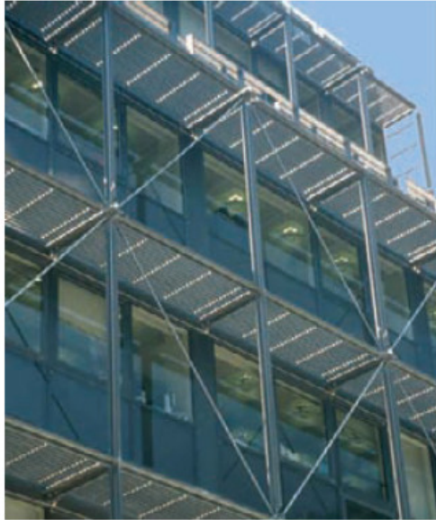
Figure 3.7: Metal overhangs of Office Building in Finsbury Avenue, London [12].
