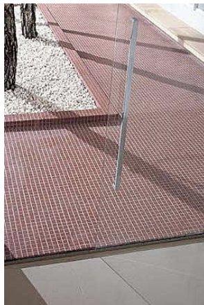
Figure 4.2 : Floor application of non-slip ceramic mosaic tiles [51]
