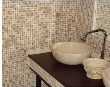
Figure 4.6 : Wall application of stone mosaic tiles [51]
