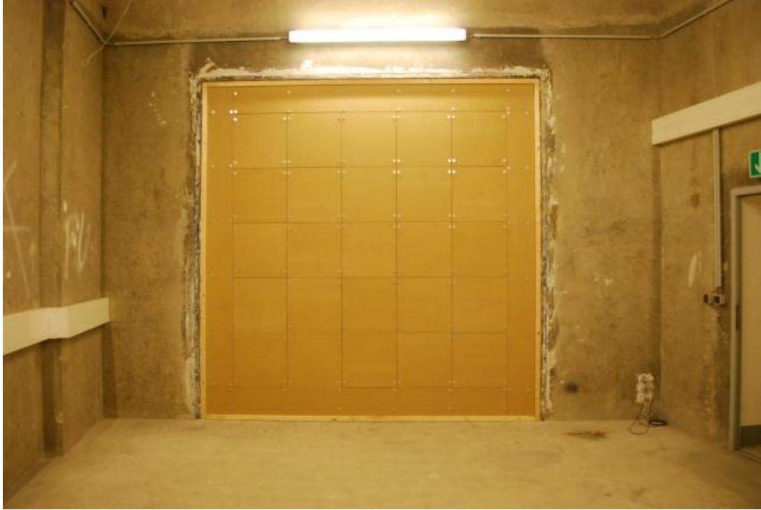
Figure 3.8: Completed double façade experiment wall.
