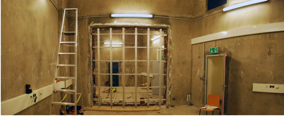
Figure 3.6: Finished aluminium structure inside the test opening.
