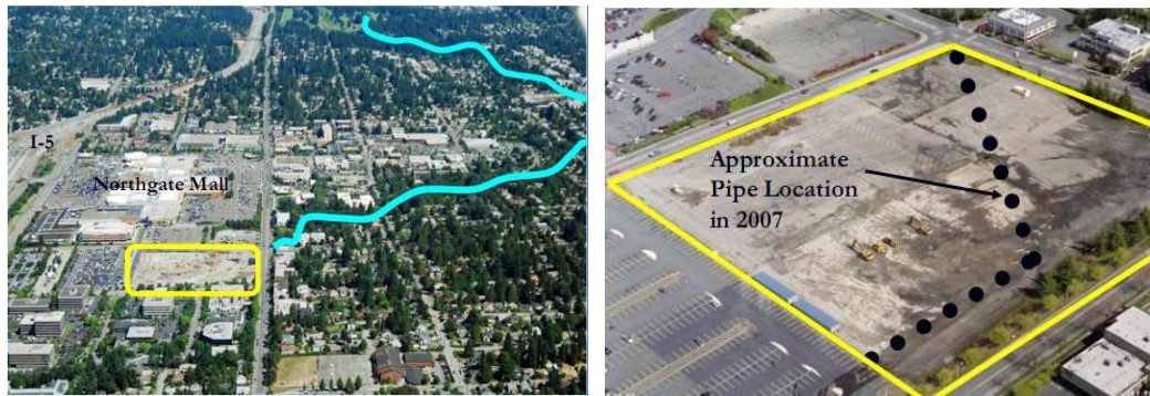
Figure 4.4 : Thornton Creek Water Quality Channel and the parking lot with pipe under it. (Mayhew, 2009).
