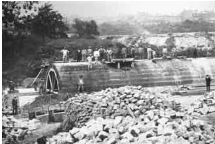
Figure 4.1 : Wingohocking Creek Sewer Construction in 1909 (Buchholz and Younos, 2007).
