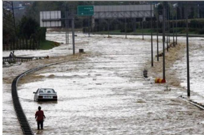
Figure 5.17 : Main roads served as drainage channels (Basin Expres link road, September 9, 2009) (Ozcan and Musaoglu, 2010).
