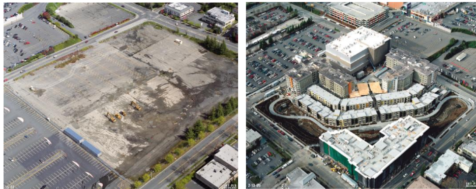
Figure 4.13 : Thornton Creek before and during construction (Mayhew, 2009).
